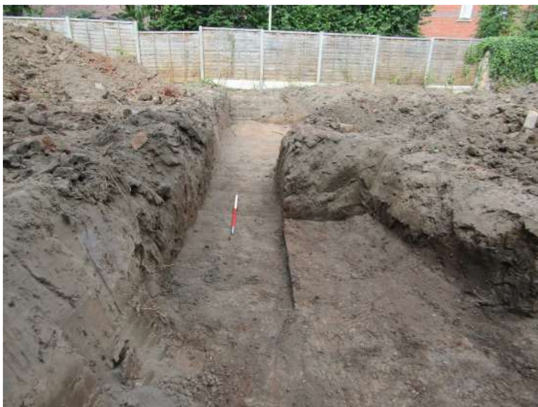
Figure 29: Stripped Area 2 (centre), looking north
