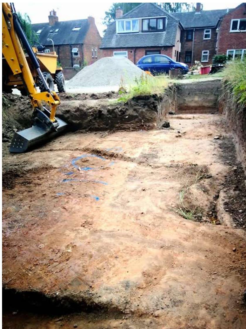
Figure 4: Area 1, working shot showing Trench 1 left open, looking east
