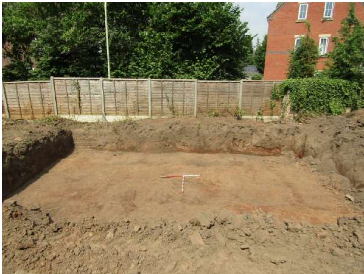
Figure 27: Stripped Area 2 (north), looking north
