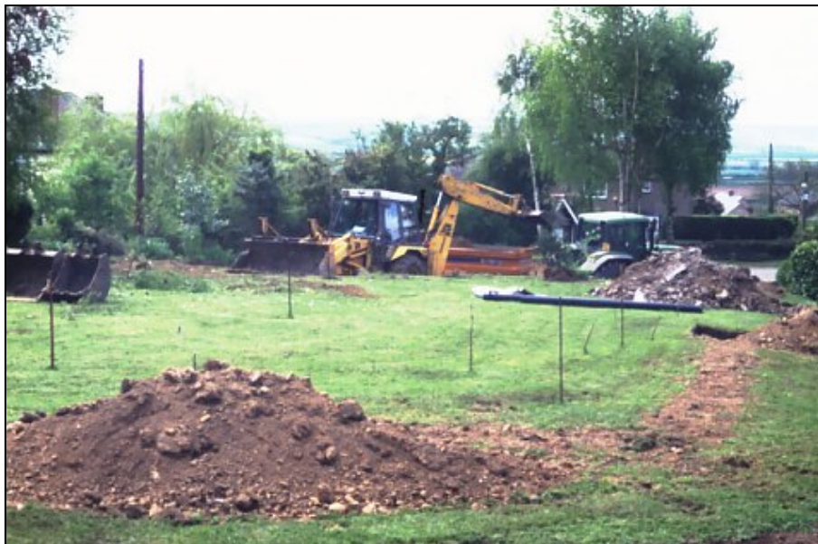
Plate 2. Site viewed from existing house looking south. Half of site excavated.
