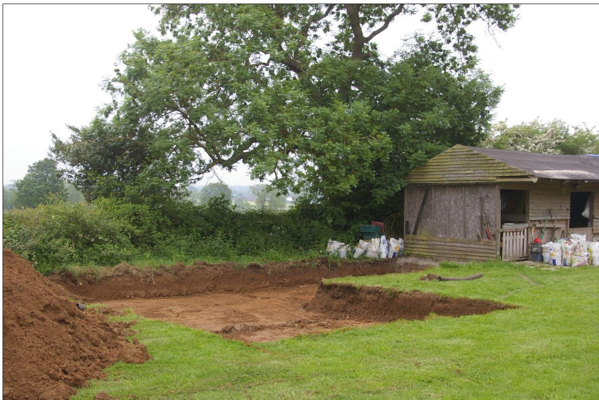
Figure 8: Area 1 following excavation
