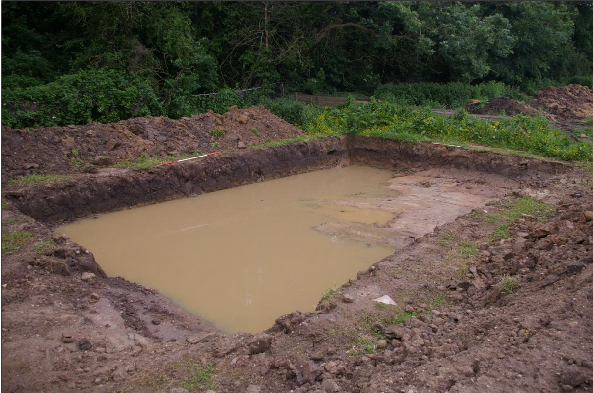
Figure 10: Area 2 following excavation. Natural ground observed prior to flooding
