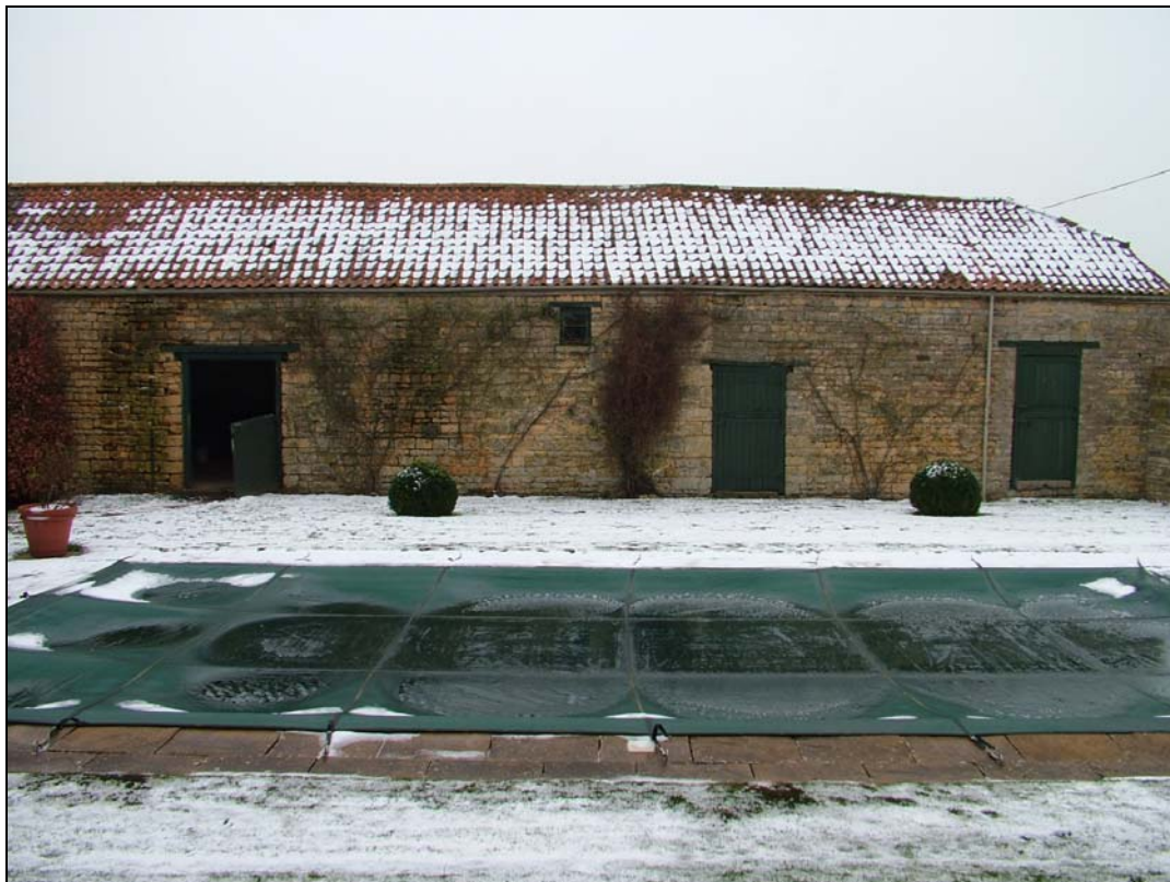
Plate 7. Northwest elevation of Barn E
