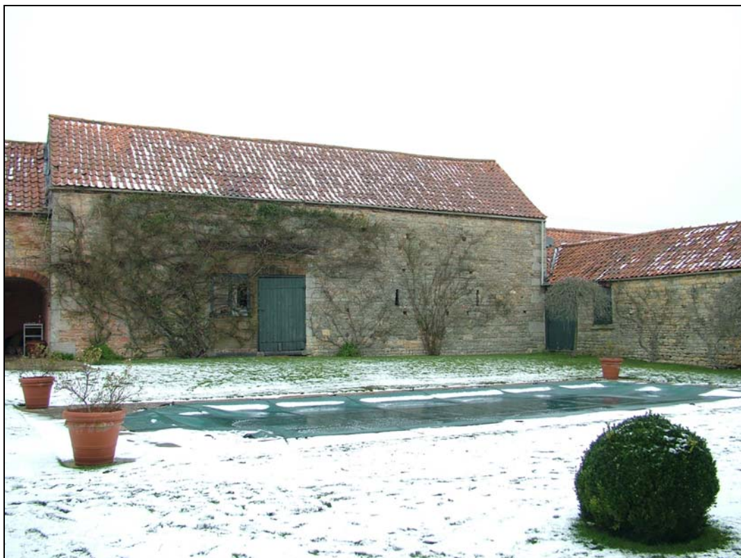
Plate 2. Southeast face of Barn B.
