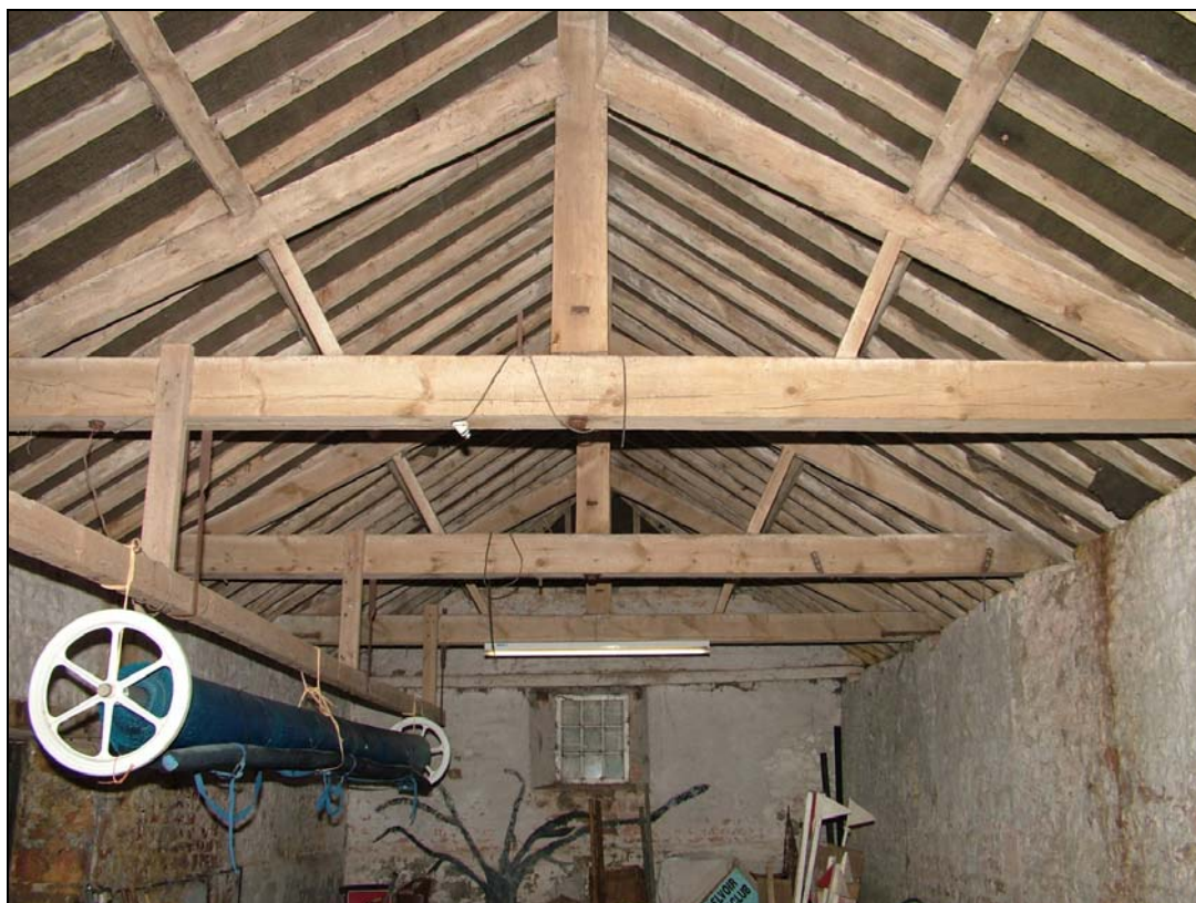
Plate 8. Roof structure of Barn E
