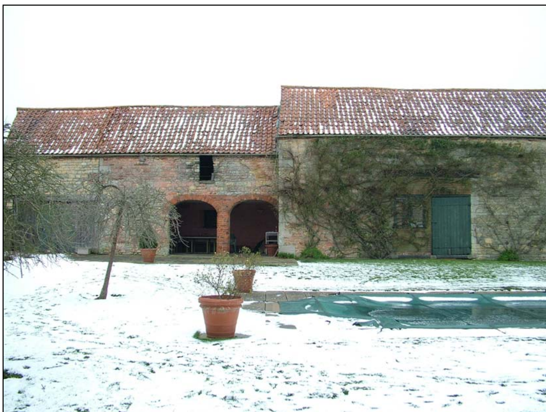
Plate 3. Southeast face of Barn A and B
