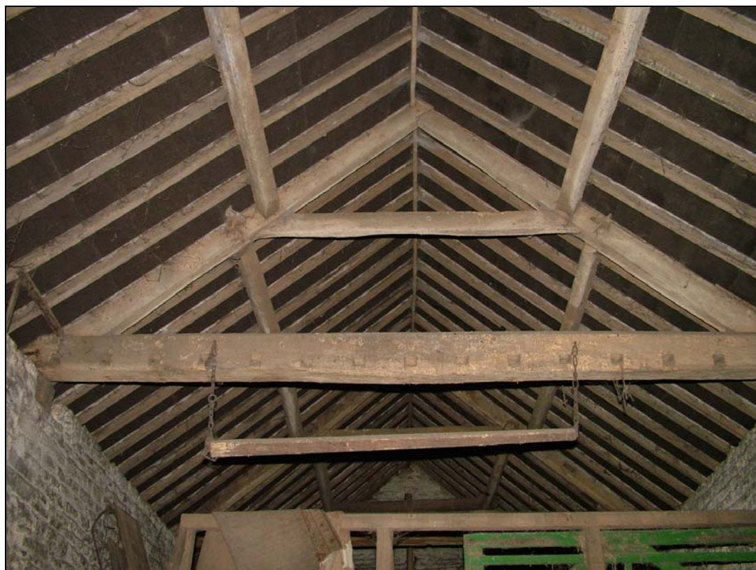
Plate 6. Roof structure of Barn B
