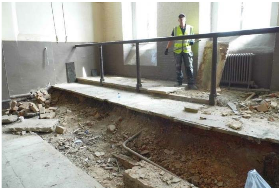
Figure 26: Public gallery removal
