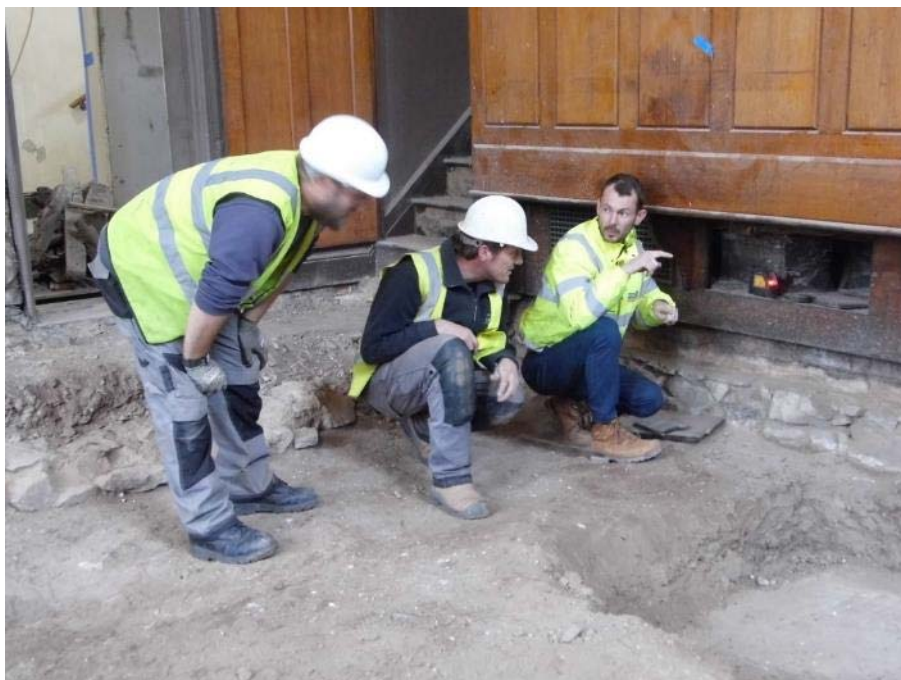
Figure 37: Levelling the western aisle padstone
