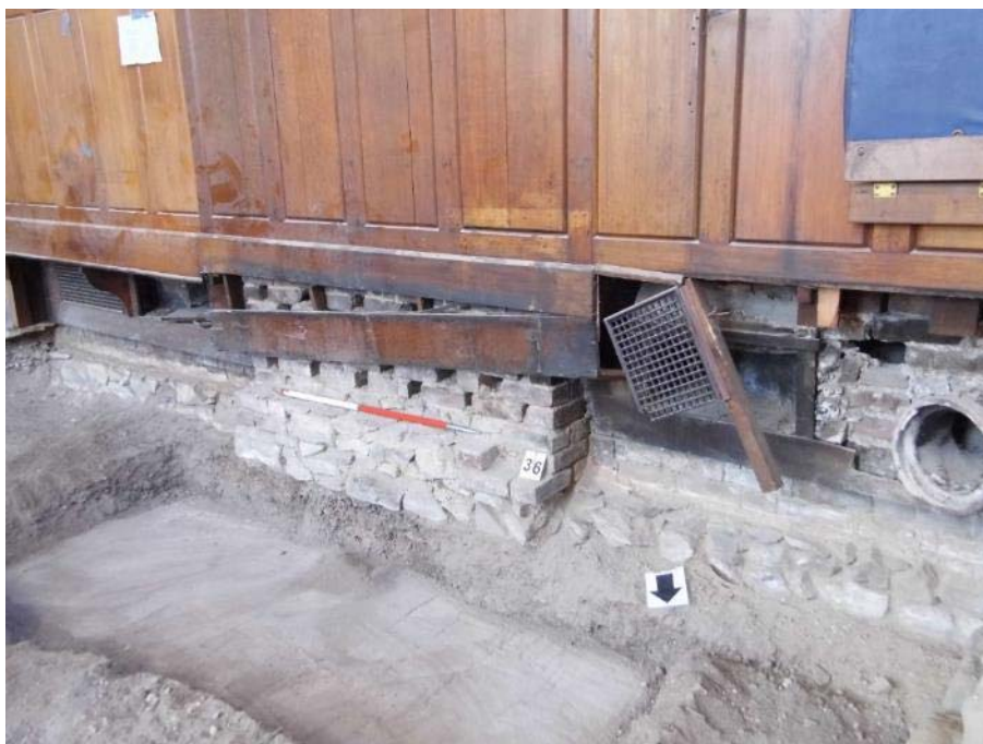
Figure 43: Stone support (36), looking southwest, 1m scale
