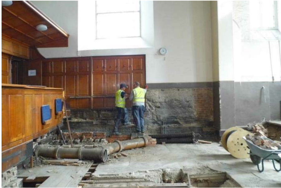
Figure 24: Removing panelling, north wall
