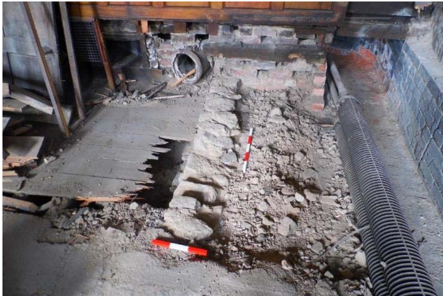
Figure 25: Stone supports revealed
