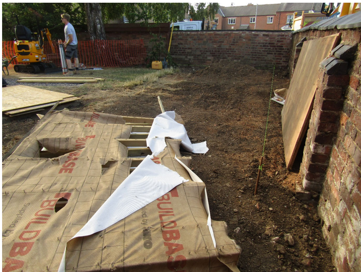
Figure 5: Area prior to excavation looking south
