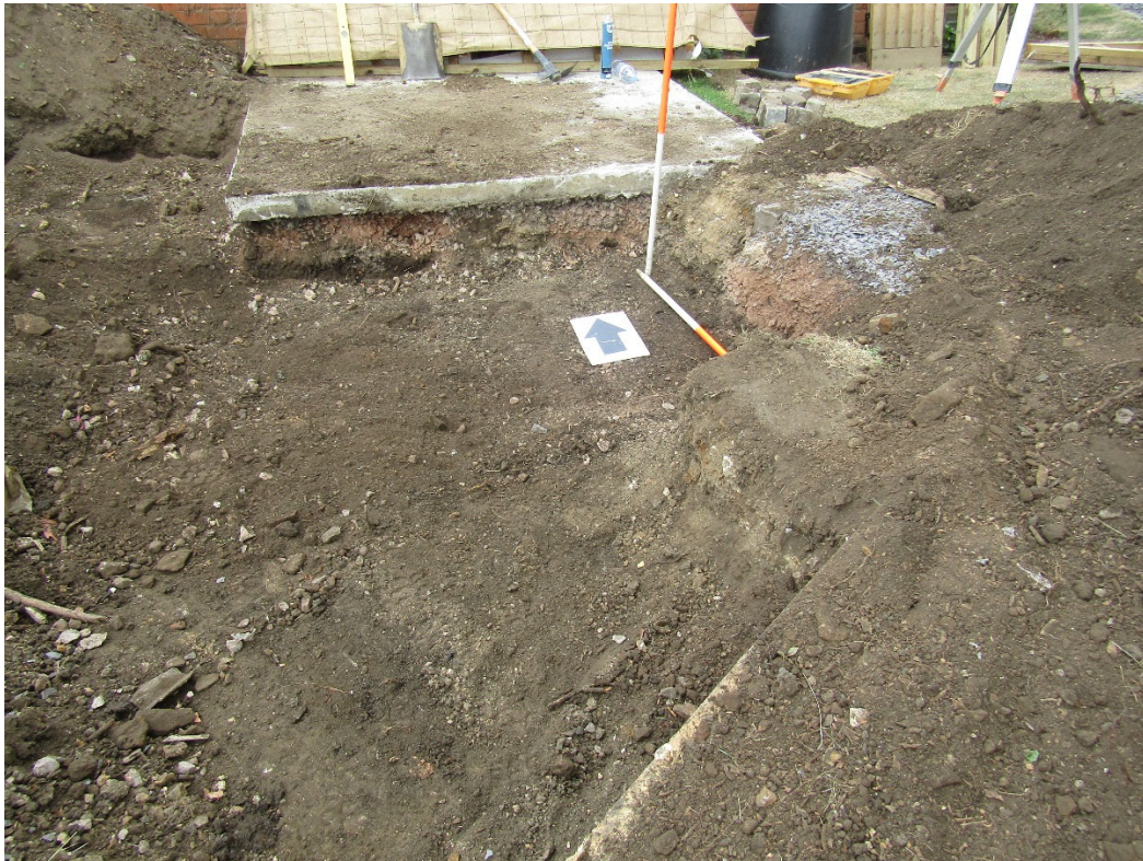
Figure 9: Remaining part of the north eastern corner post excavation looking north. Photograph shows the existing concrete shed base and its hard-core footing which will be removed to the same depth as the rest of the area. Scale 1.0m
