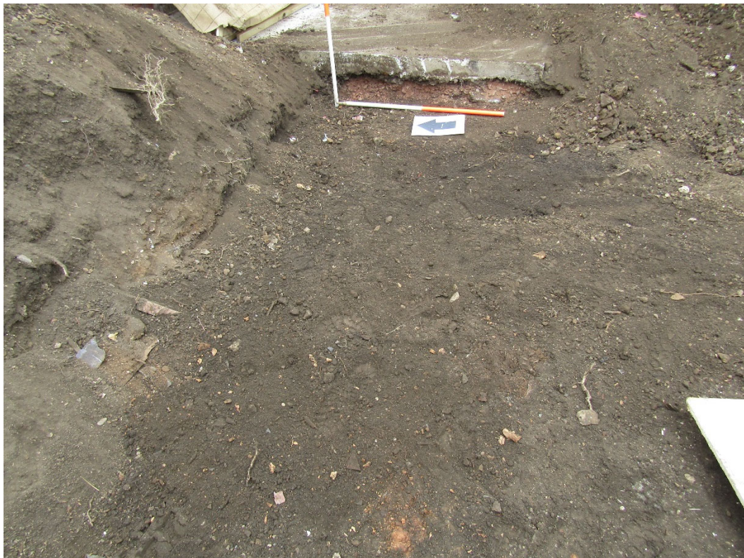
Figure 8: Part of the north eastern corner post excavation looking east. Photograph shows the existing concrete shed base and its hard-core footing which will be removed to the same depth as the rest of the area. Scale 1.0m.
