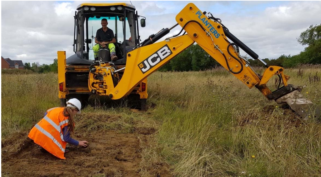
Figure 3: Ecologist inspecting excavation area prior to machining
