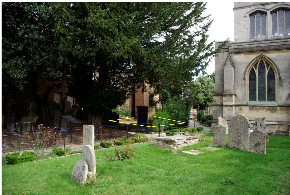
Figure 3 Proposed building location Looking north-east. Boiler-house outlined in yellow. North transept on right
