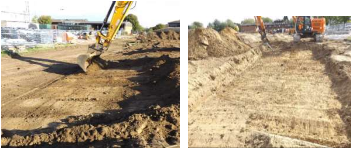
Figures. 6 & 7. The removal of the made ground with mechanical excavator
