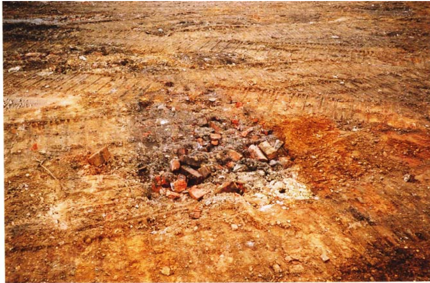
Figure 4 Coal cellar disturbance cutting the substratum at the northern end of the site.
