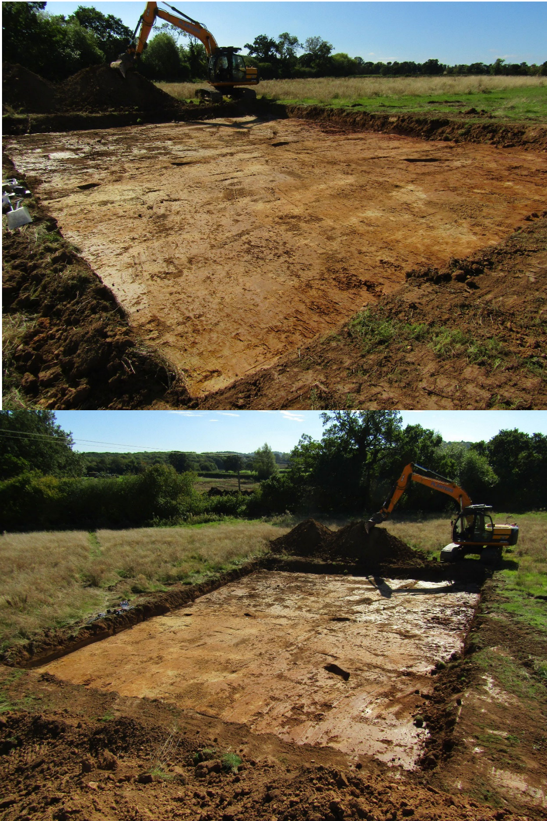
Figure 7: Views of excavated area looking SW and SE
