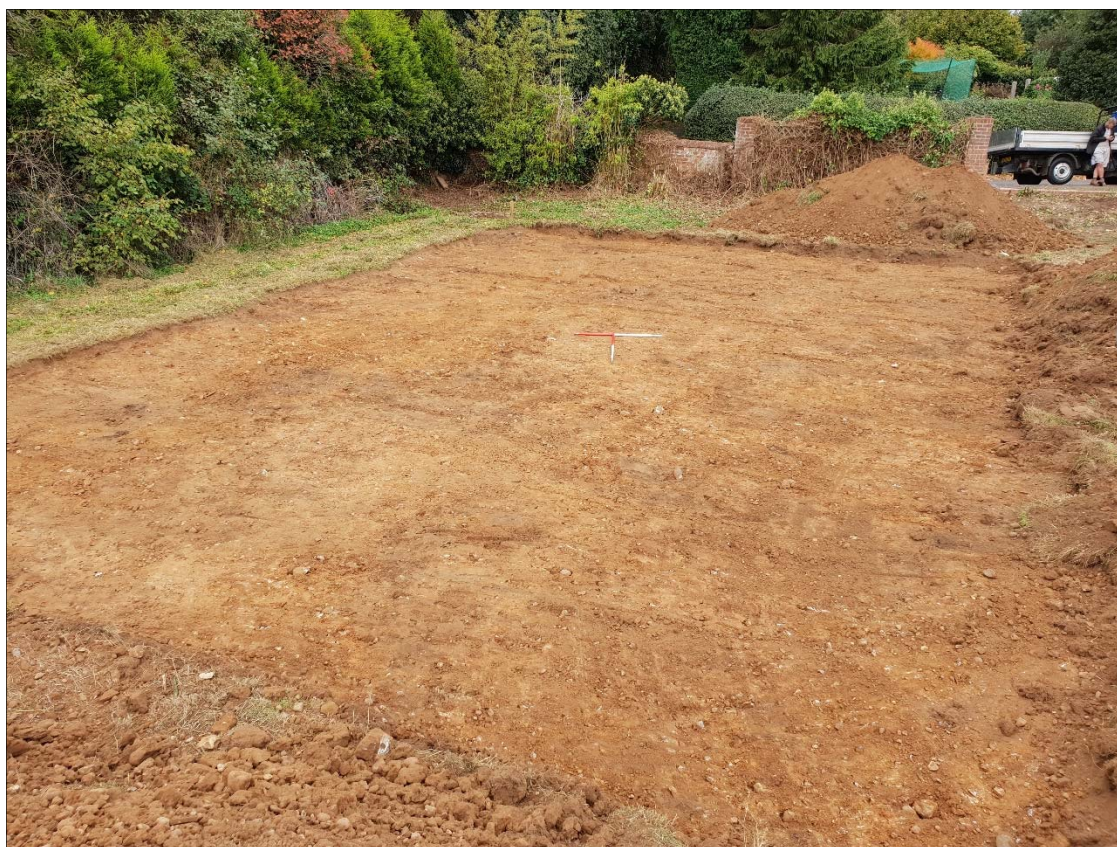
Figure 5: Exposed footprint of proposed dwelling, looking north-west
