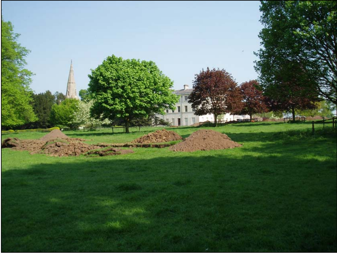
Plate 1. Looking northeastwards over trenches towards Hall and church.
