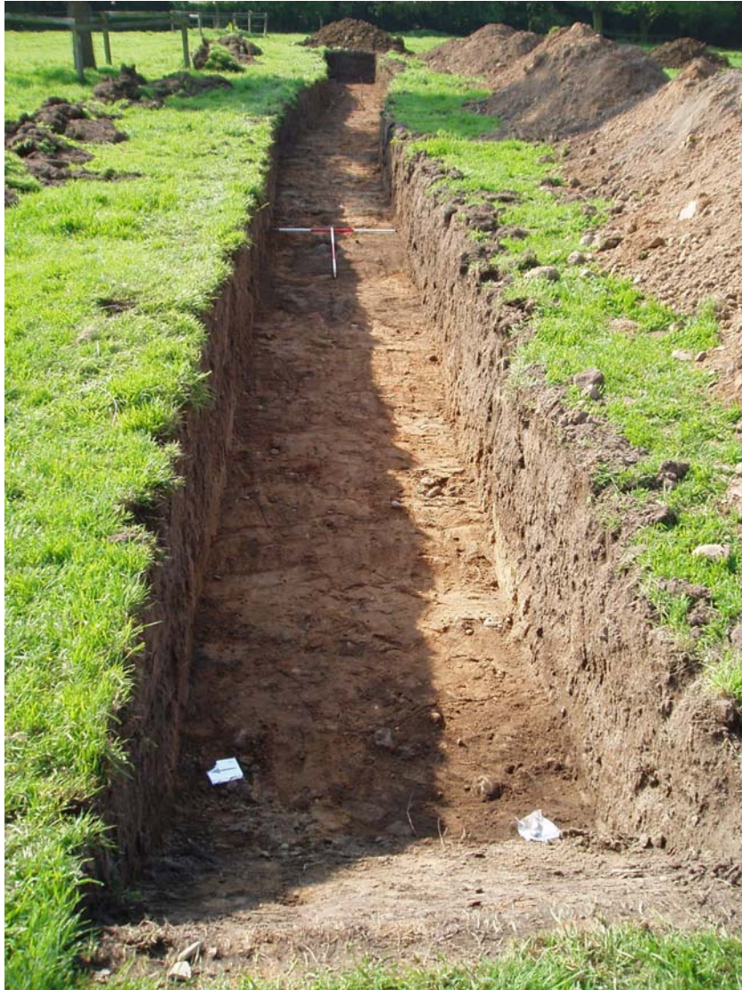
Plate 3. Trench 1 looking east.
