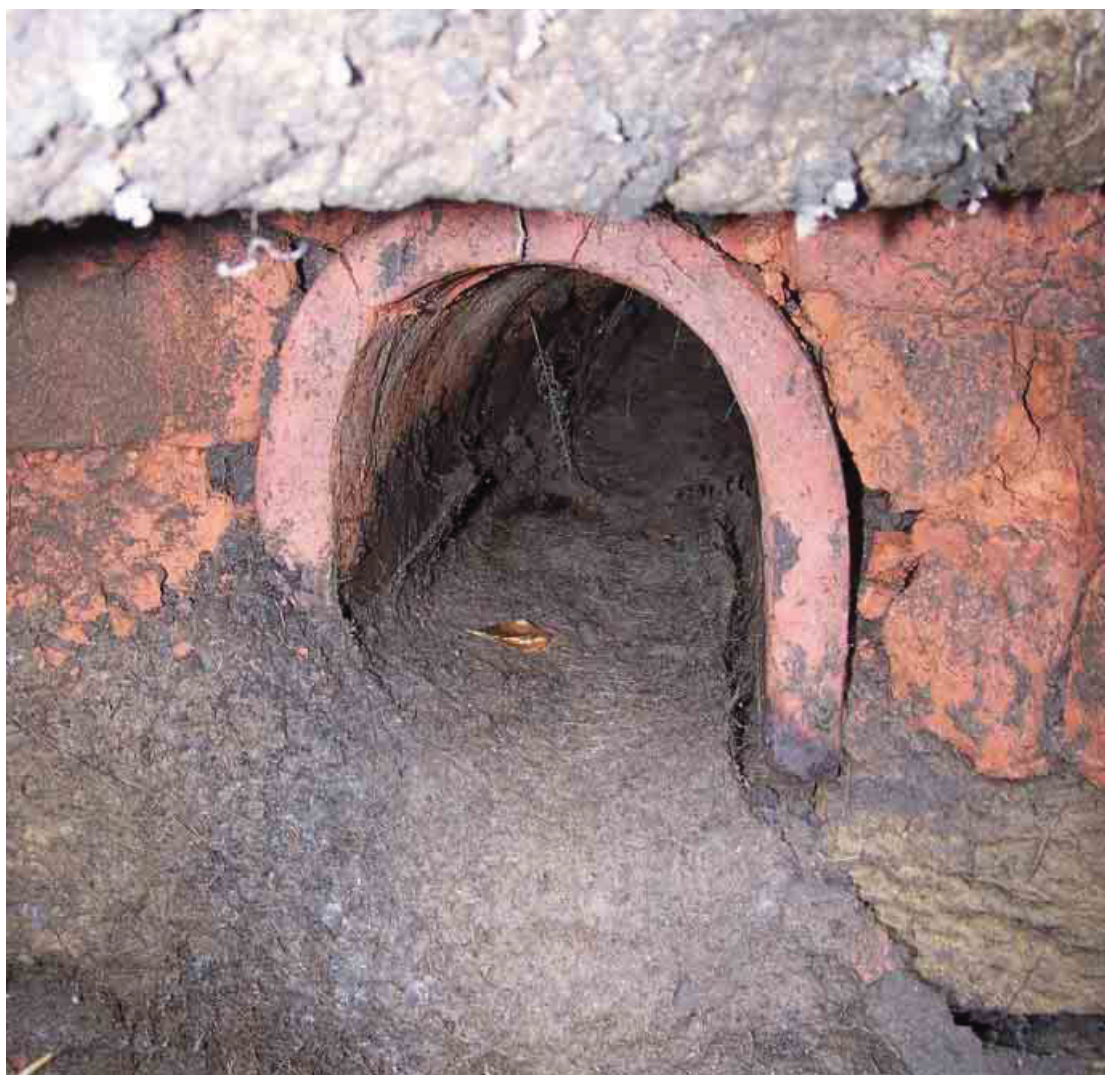
Plate 3: Horseshoe land drain at top of 'well' – note that the drain was dry
