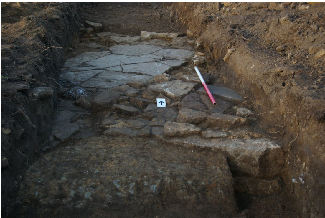
Figure 5 – View of building remains, showing small hand-excavated slot to the south-east that revealed a second course of iron-stone foundations
