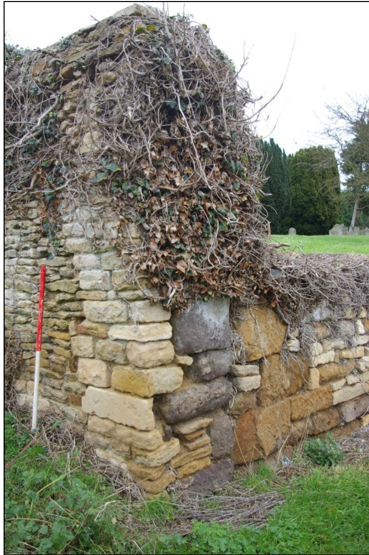
Figure 8 – Evidence for earlier building within boundary wall of Church Farm and All Hallows Church, looking north-east from Church Lane
