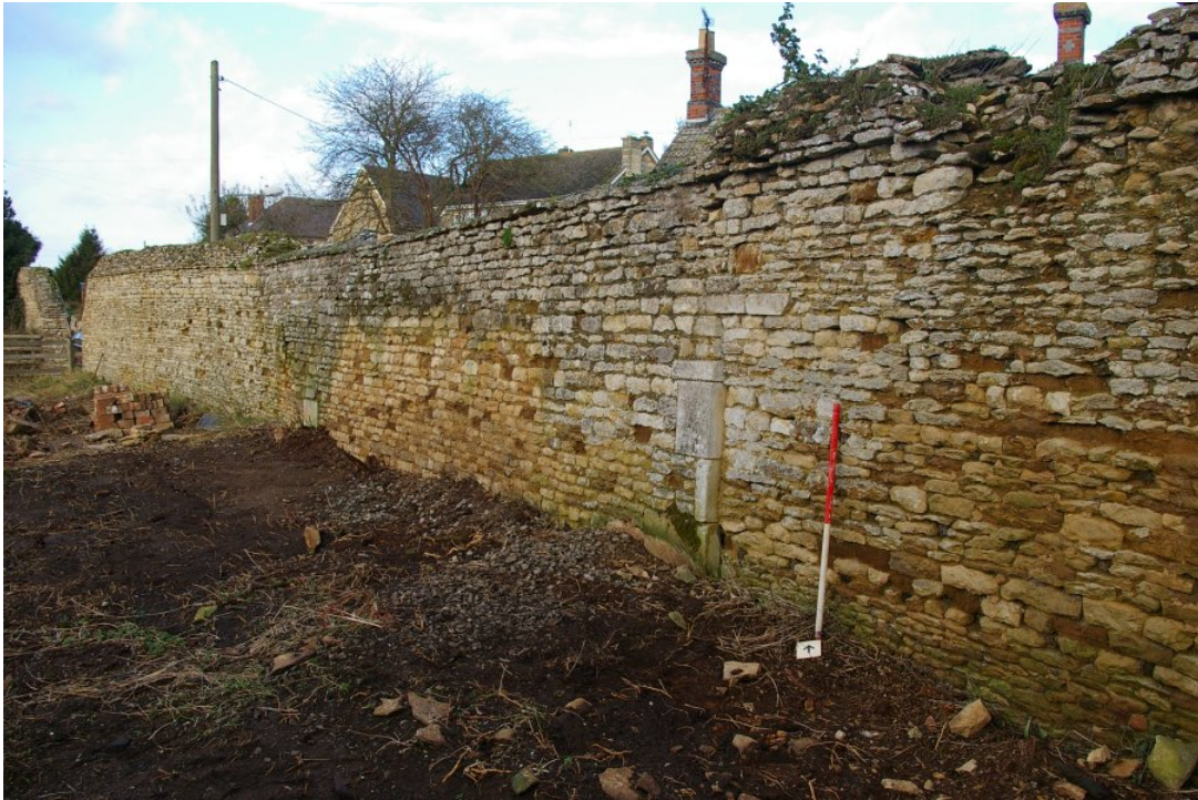
Figure 6 – Evidence for earlier building within surrounding wall of Church Farm, looking north from within grounds of Church Farm.
