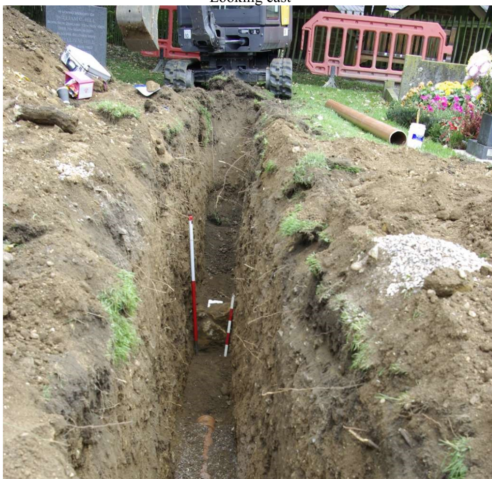
Figure 12 North to south wall Looking east. 1 and 0.5m scales
