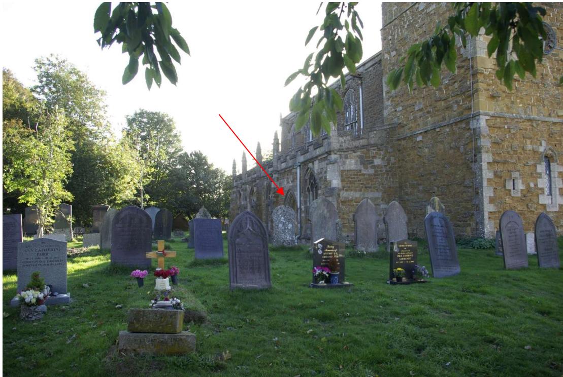
Figure 4 North side of the north aisle Looking south-east. 1m scale. Red arrow points to the blocked north door
