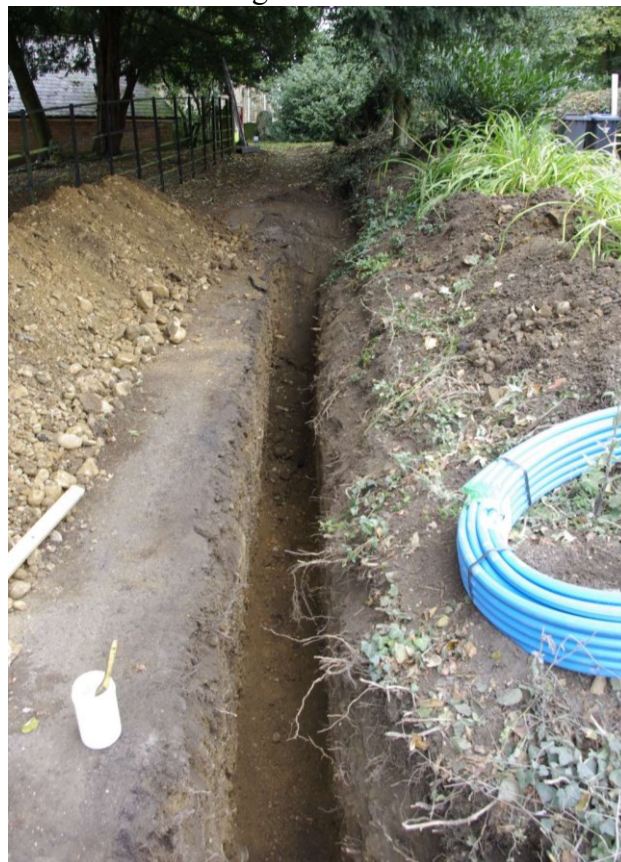
Figure 14 Trench along pathway to Oakham Road Looking west
