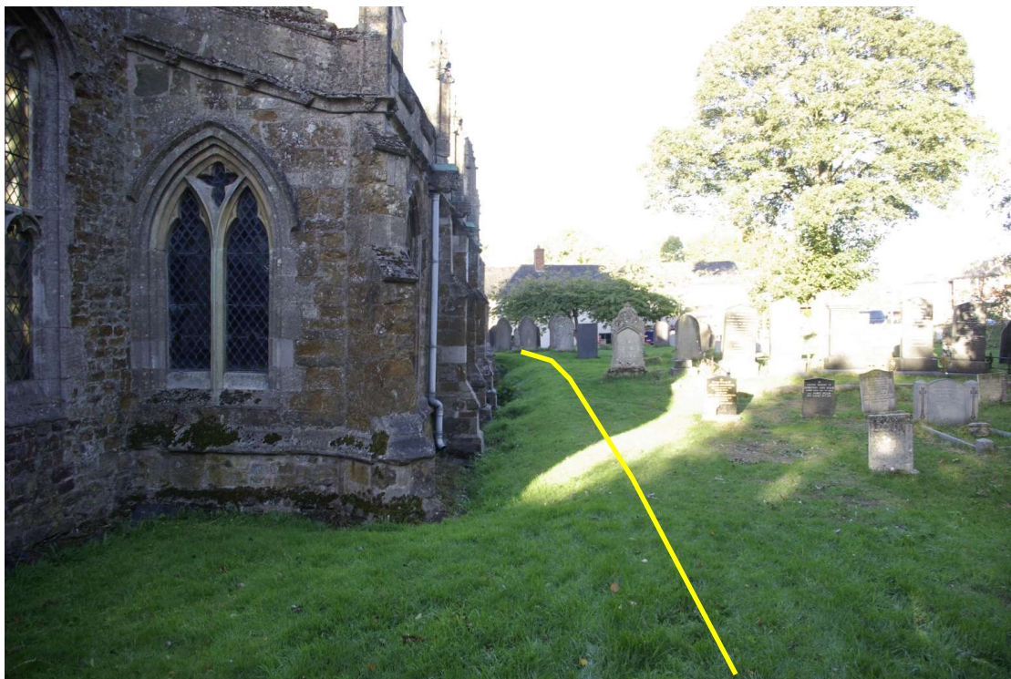
Figure 5 North side of the north aisle Yellow line shows approximate line of pipe trench. Note difference in height of grassed churchyard and the base of the church walls
