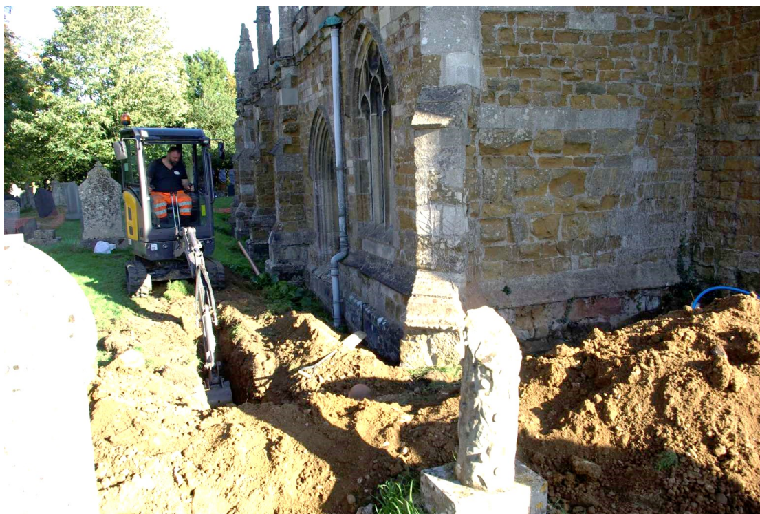
Figure 11 Sewer trench being excavated eastwards Looking east
