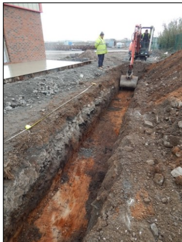
Figure 5 Excavation of the new service trench looking east
