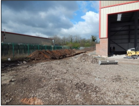
Figure 4 New service trench looking west
