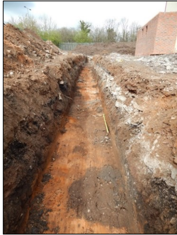
Figure 6 Excavated trench looking northwest
