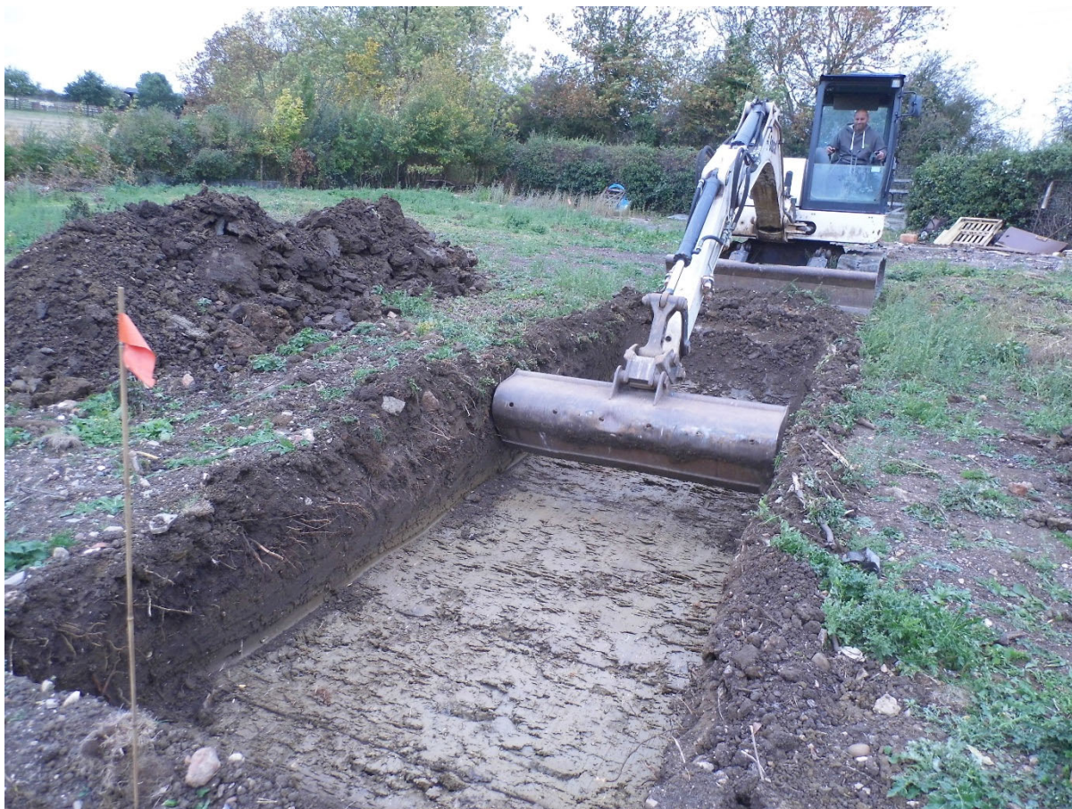
Figure 4: Excavation of the trenches.
