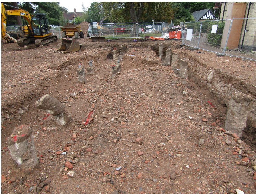
Figure 9: Upper portion of site, looking west towards London Road.
