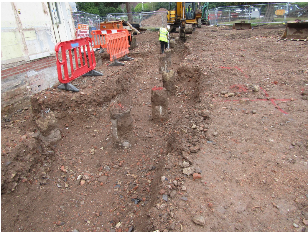
Figure 8: Foundation trenches in the upper area, looking west towards London Road.
