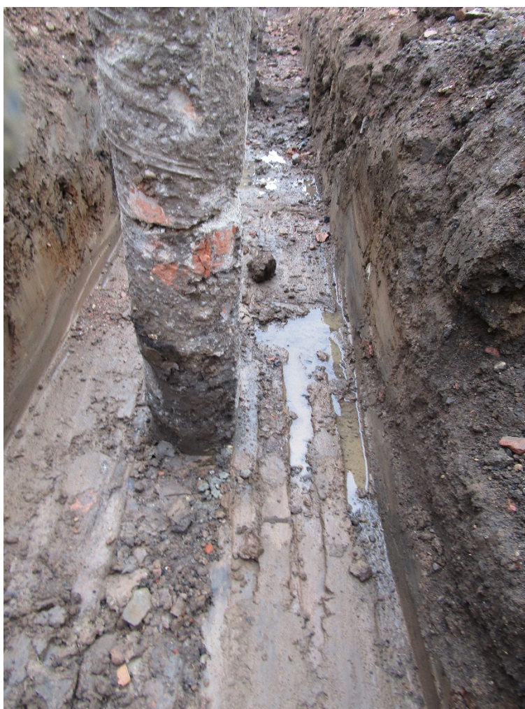
Figure 10: Deeper foundation trench (c1.10m) looking north.
