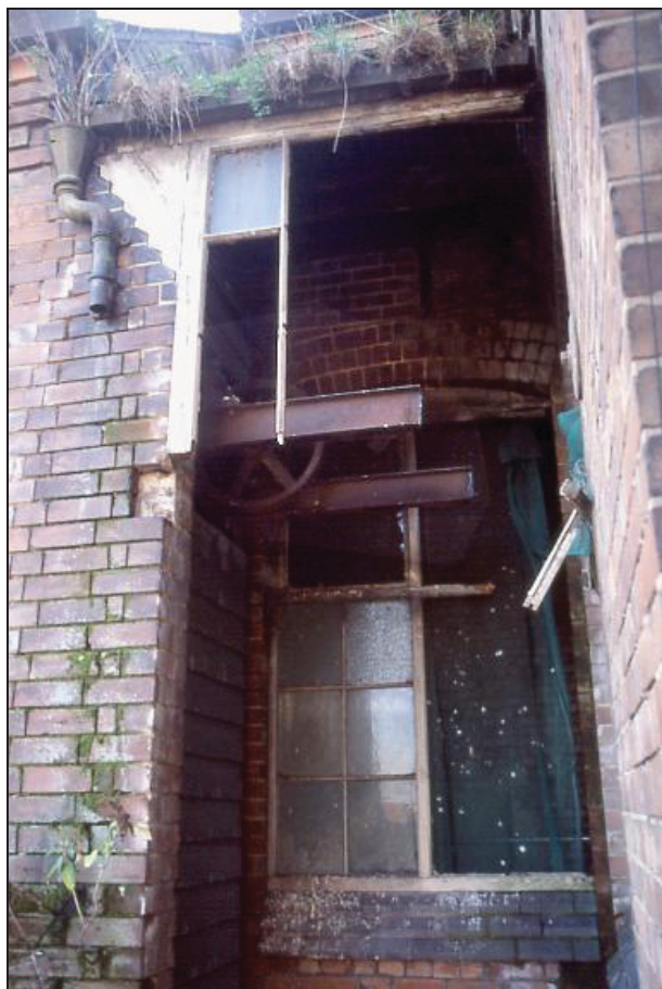
Plate 23 Top floor exterior: part of lift mechanism in south west wing
