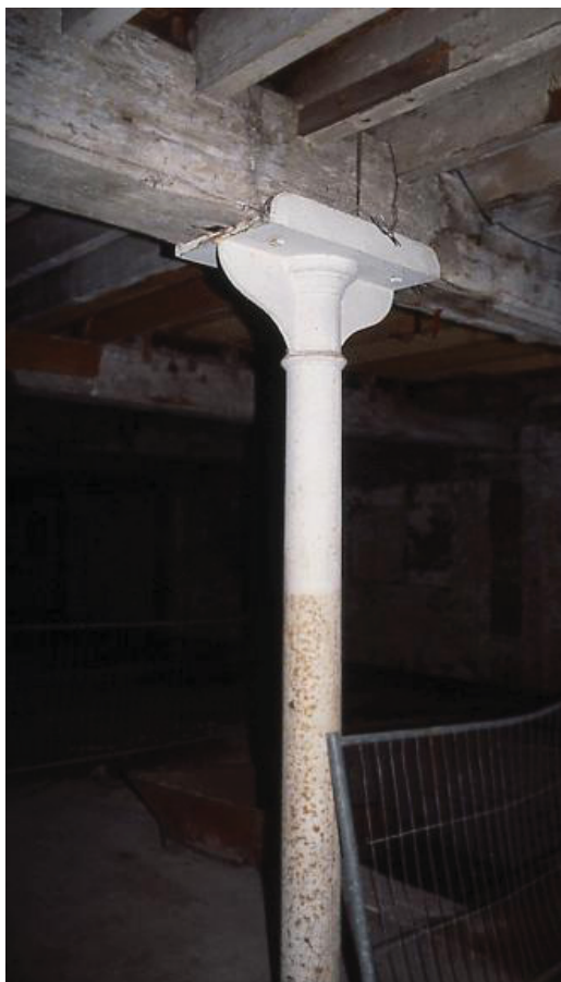
Plate 9 Detail of column in basement
