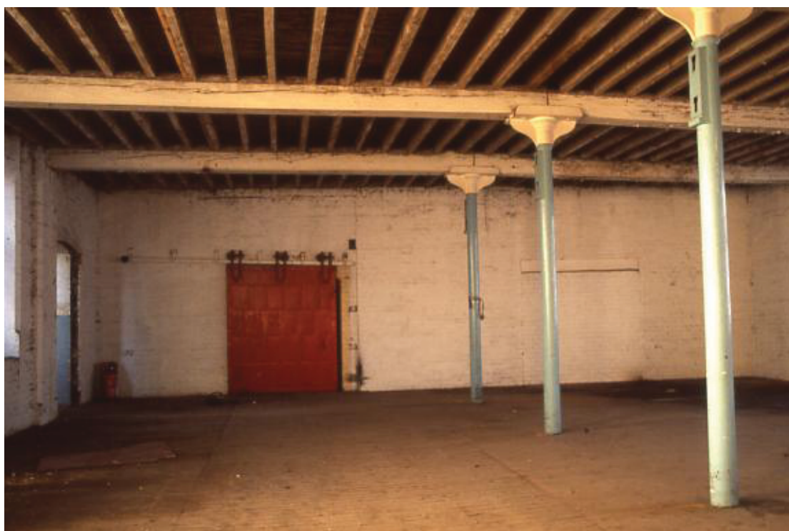
Plate 16 First floor looking west
