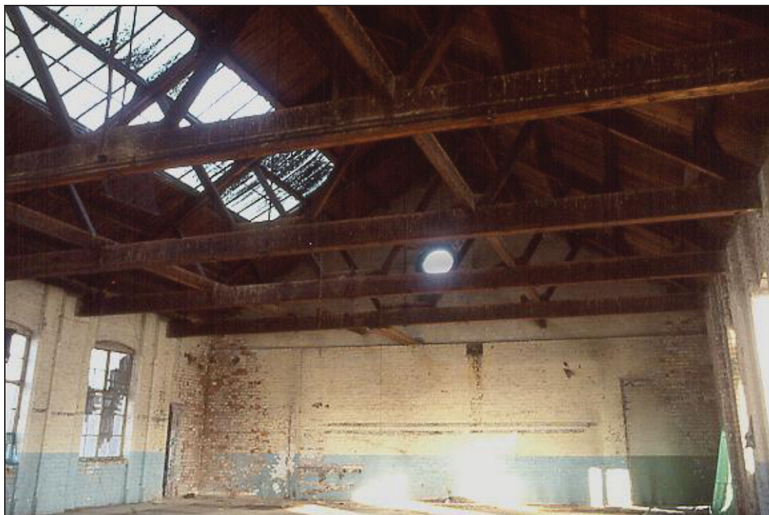
Plate 21 Top floor looking east
