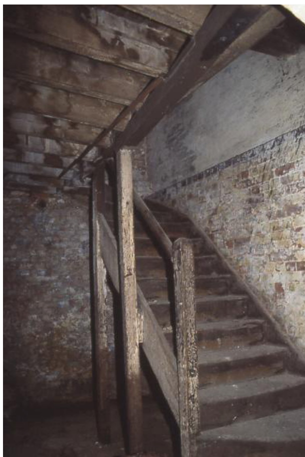
Plate 11 West staircase in basement
