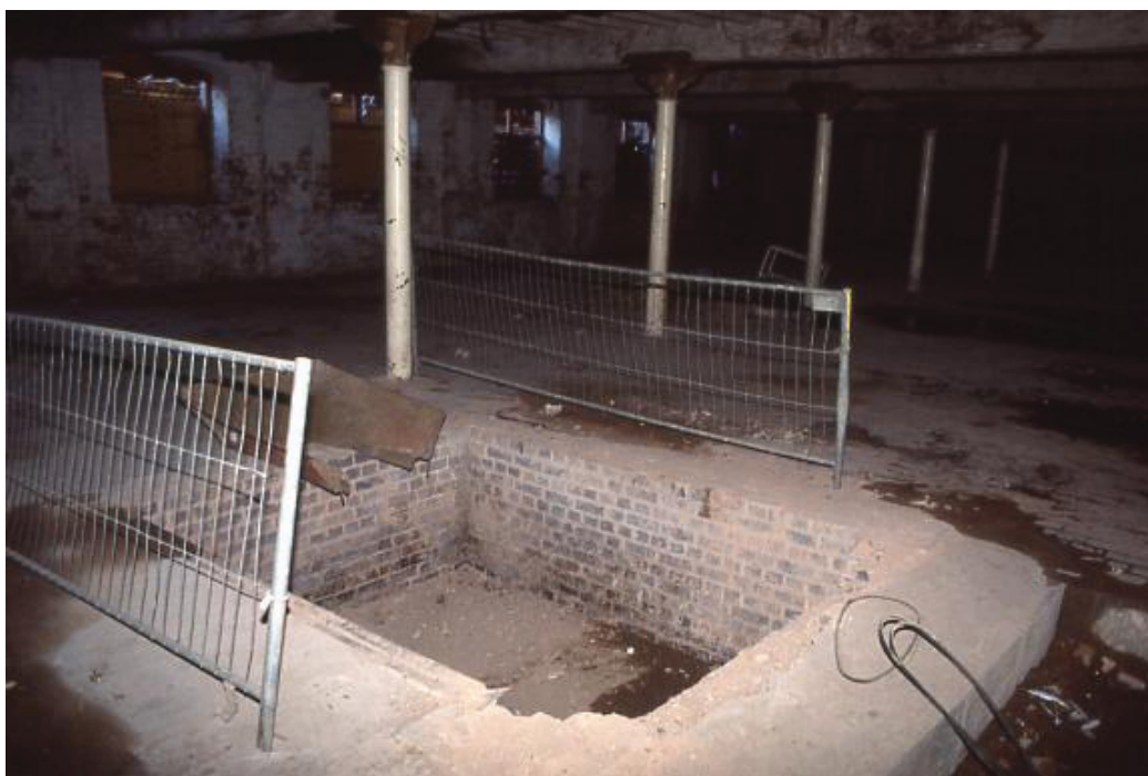
Plate 10 Modern lift base in basement
