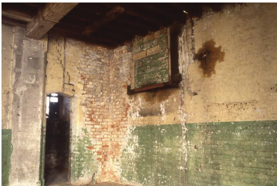
Plate 18 Second floor looking into north east corner
