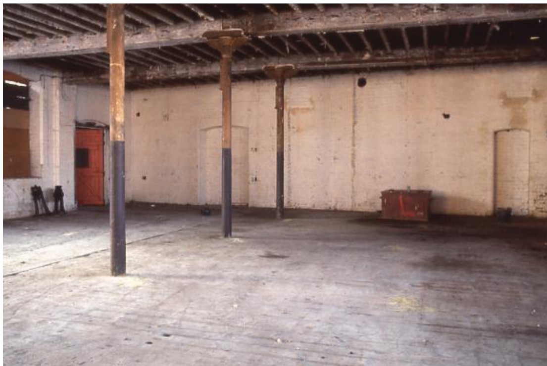
Plate 15 Ground floor looking to south west corner
