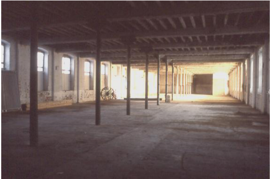
Plate 13 Ground floor looking east
