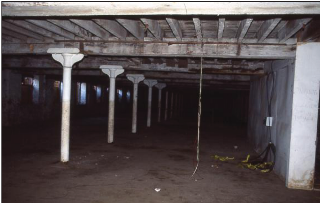
Plate 8 Basement looking west
