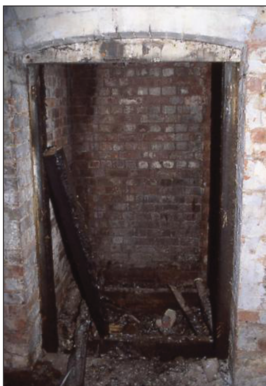
Plate 12 Base of lift shaft
