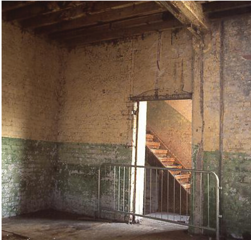
Plate 19 Second floor looking into south east corner
