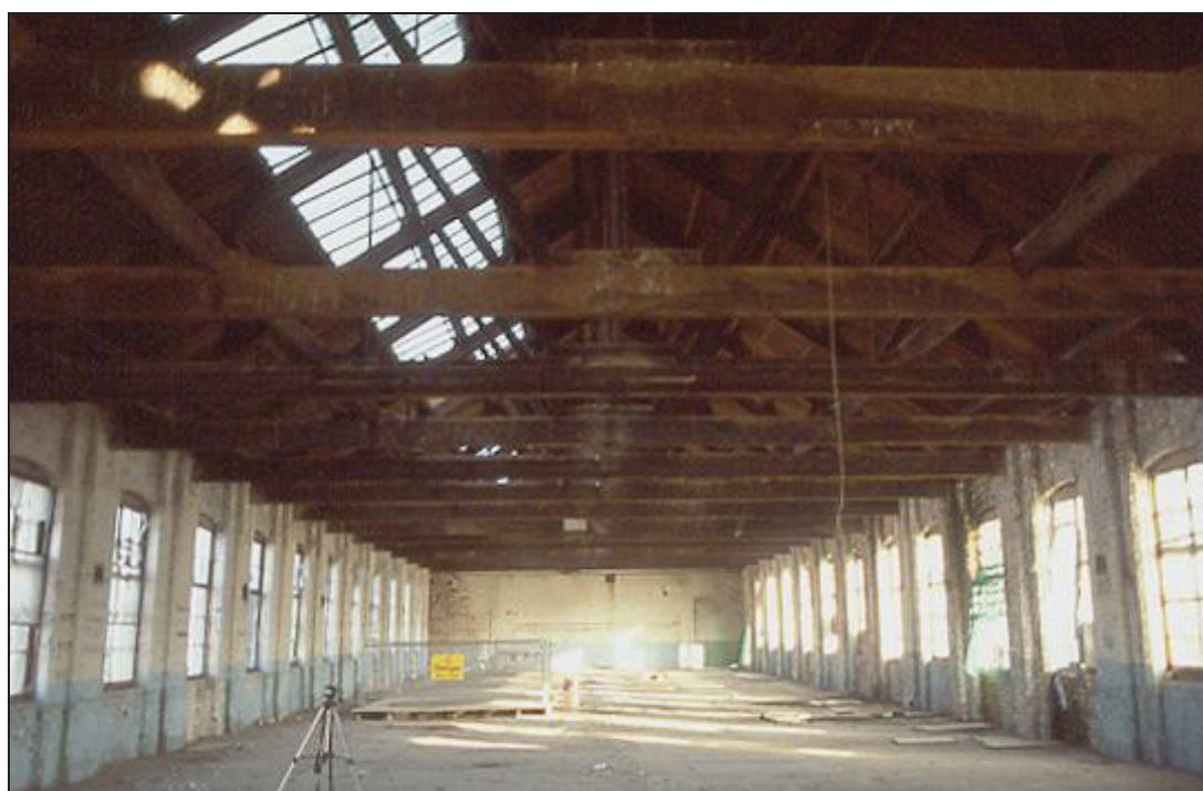
Plate 22 Top floor looking east
