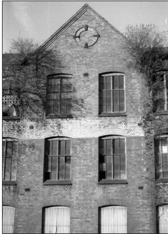
Plate 5 South facade central gable
