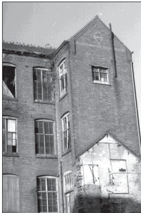
Plate 6 South facade east wing
