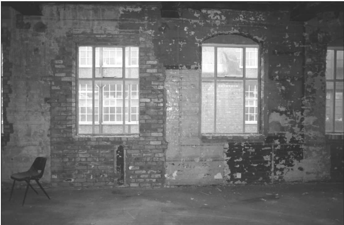
Plate 13 Deacon St range looking south east to Luke Turner building
