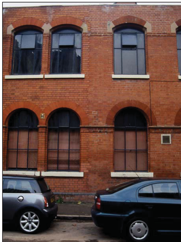
Plate 19 Grange Lane, junction of builds
