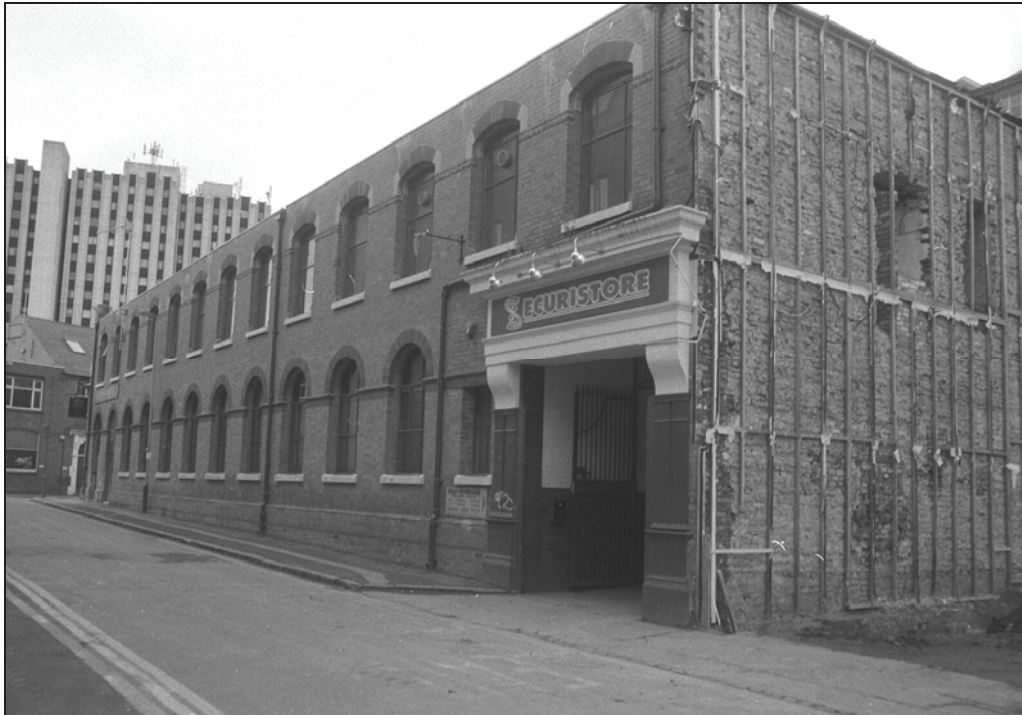
Plate 2 Deacon St frontage looking east, demolished component to the right
