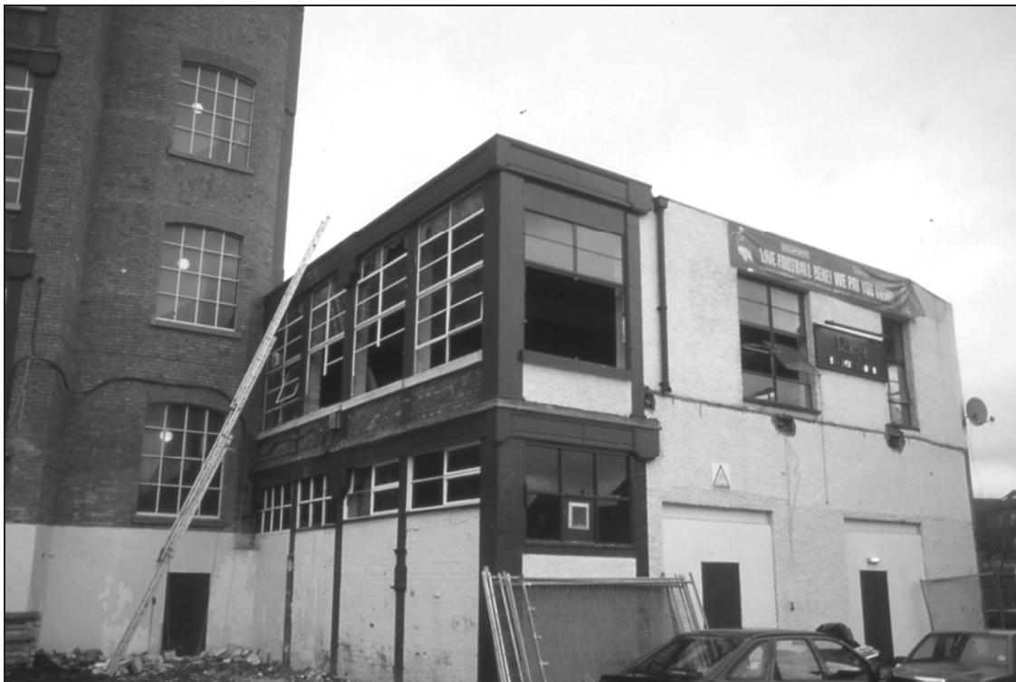
Plate 4 Rear of Grange Lane range, looking north
