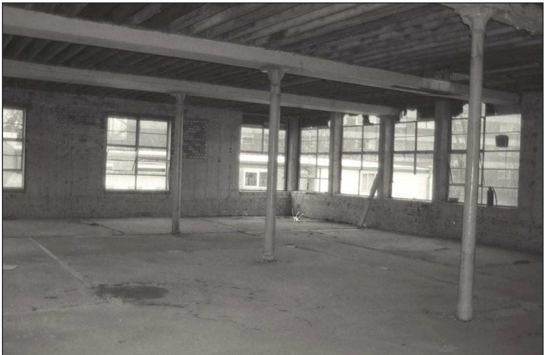
Plate 10 Interior of Grange Lane range, looking south
