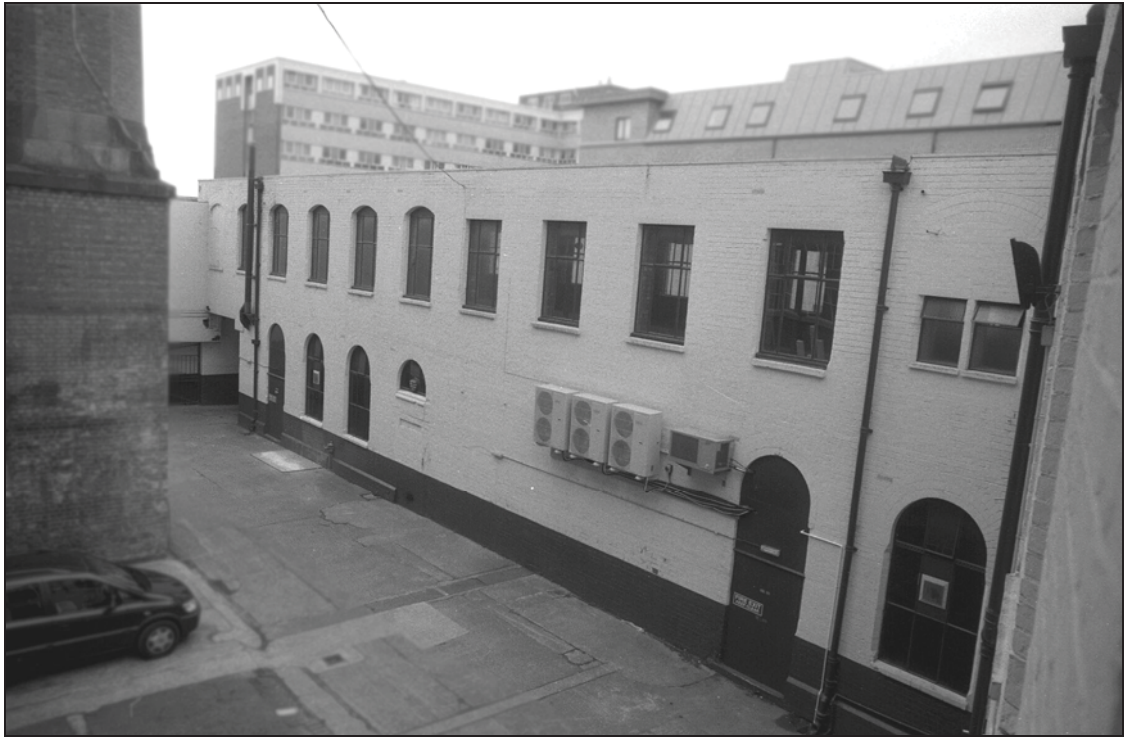
Plate 16 Courtyard and back of Deacon St range looking north west
