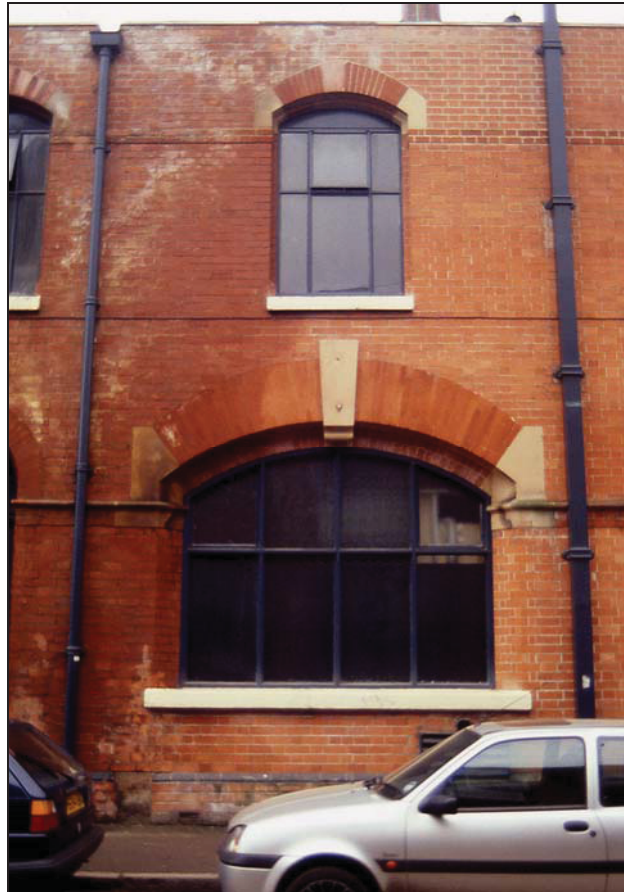
Plate 18 Grange Lane, possible blocked wagon entrance
