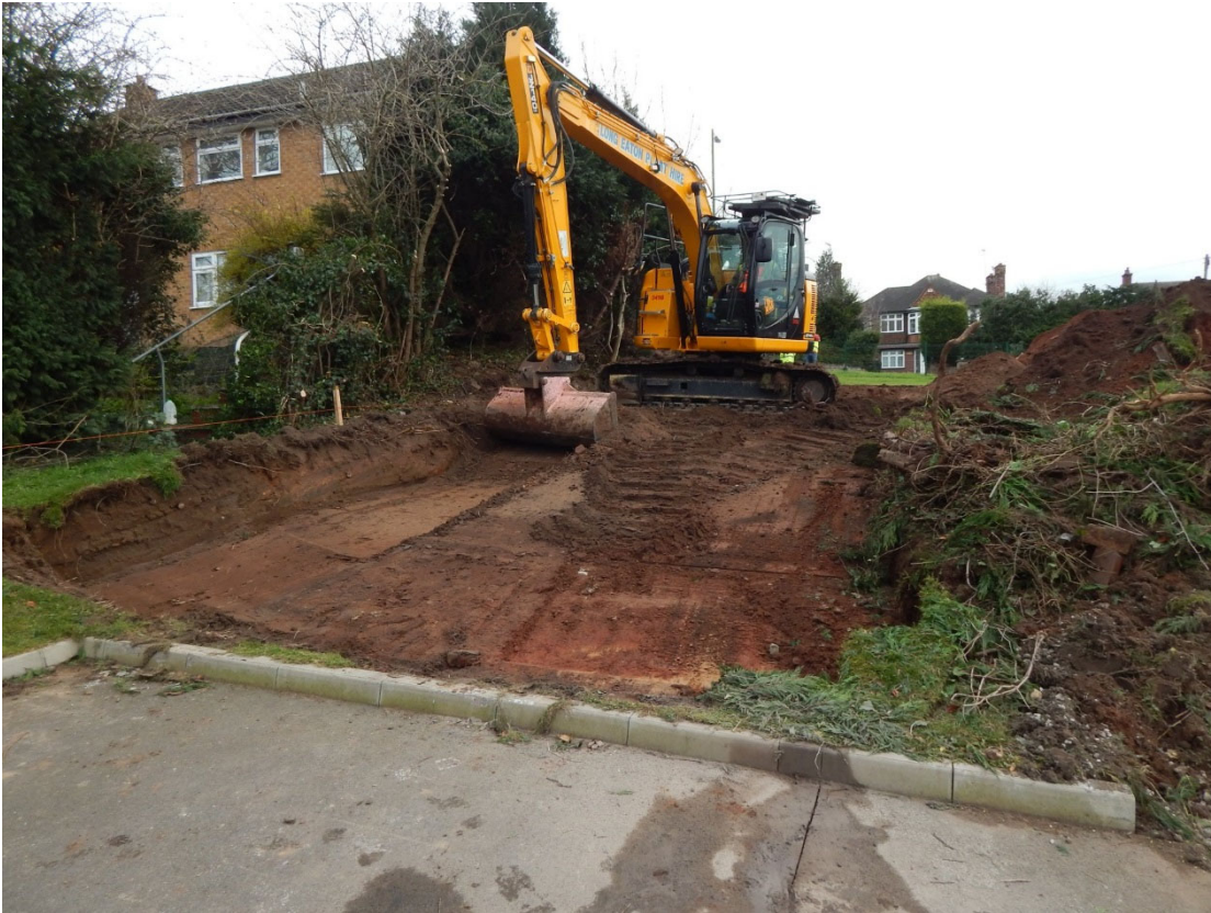
Figure 7: Excavations at north-western end of site, looking south-west
