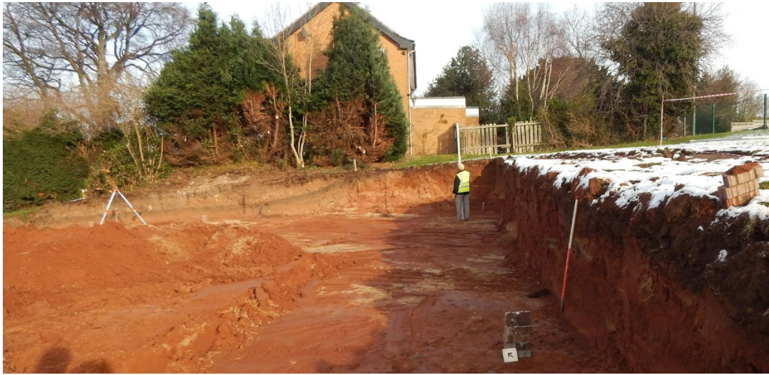
Figure 9: Excavations almost complete, looking north-east
