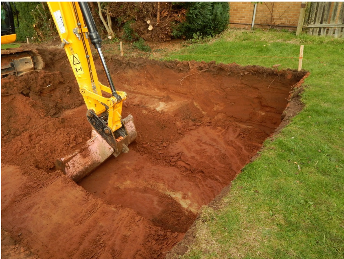
Figure 6: Work in progress on full depth dig, north-east corner
