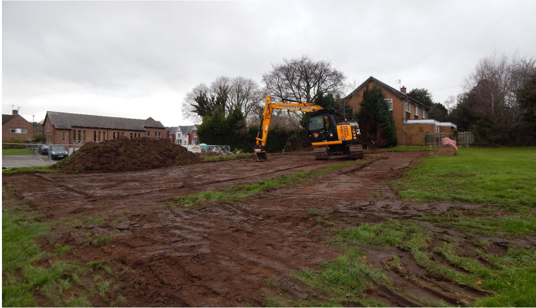
Figure 4: Work in progress, looking north
