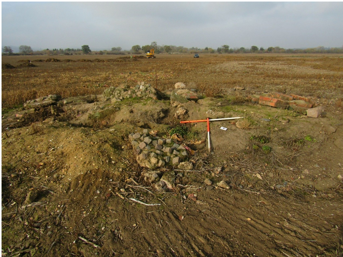
Figure 28: Photograph showing demolished structure, looking north.
