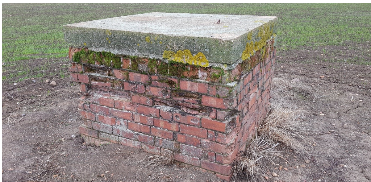
Figure 29: Complete sewage outlet in situ in adjacent field.
