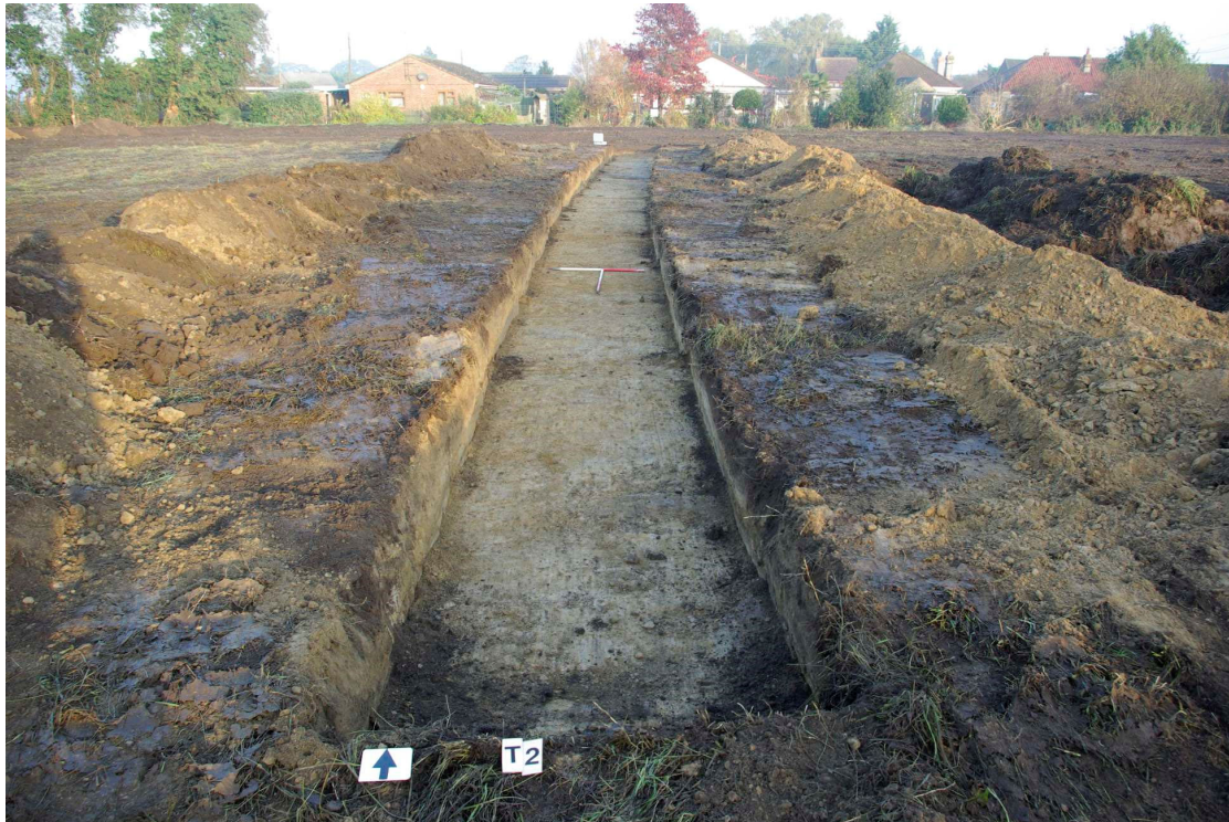
Figure 13 Trench 2 Looking towards houses on New Road. 1m scales
