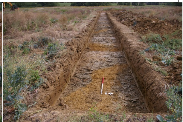
Trench 2 northern field
