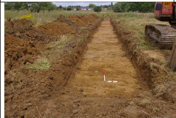
Trench 13 northern field
