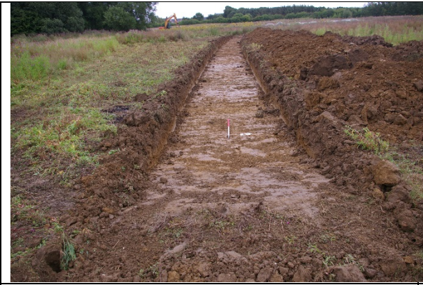
Trench 9 northern field
