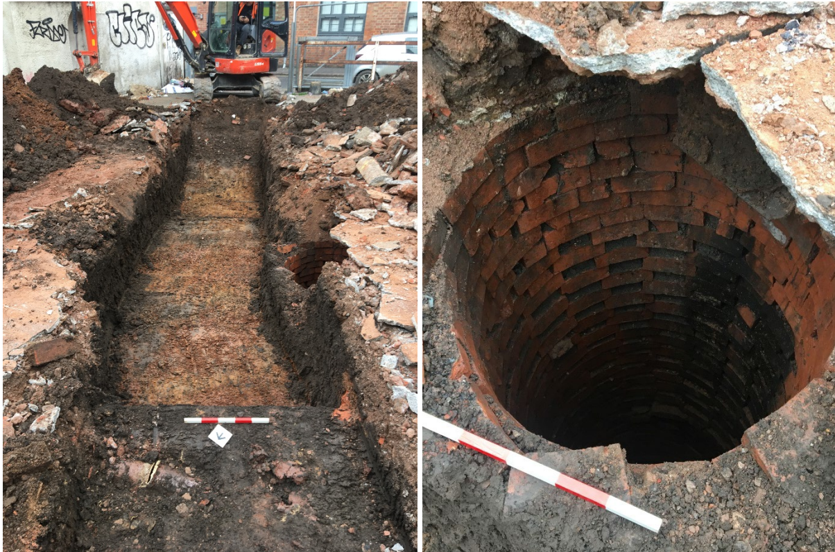
Figure 4: Left, looking south-east at Trench 1 with modern service pipe in foreground and well in the middle ground to the right. Right, the brick-lined well.
