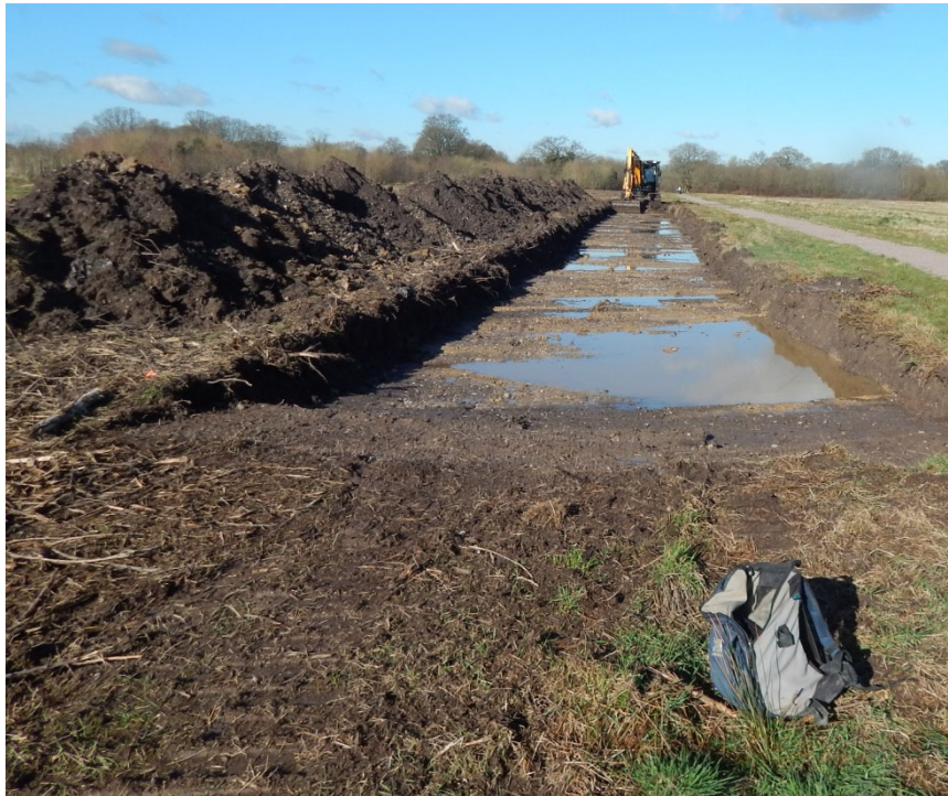
Figure 6: Top-soil stripping of Area 1. Viewing west.
