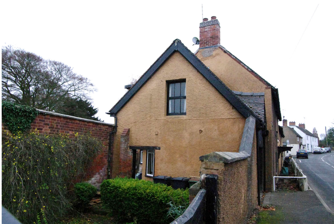
Figure 9 Gable end of covered gateway Looking south-west. Main Street on right
