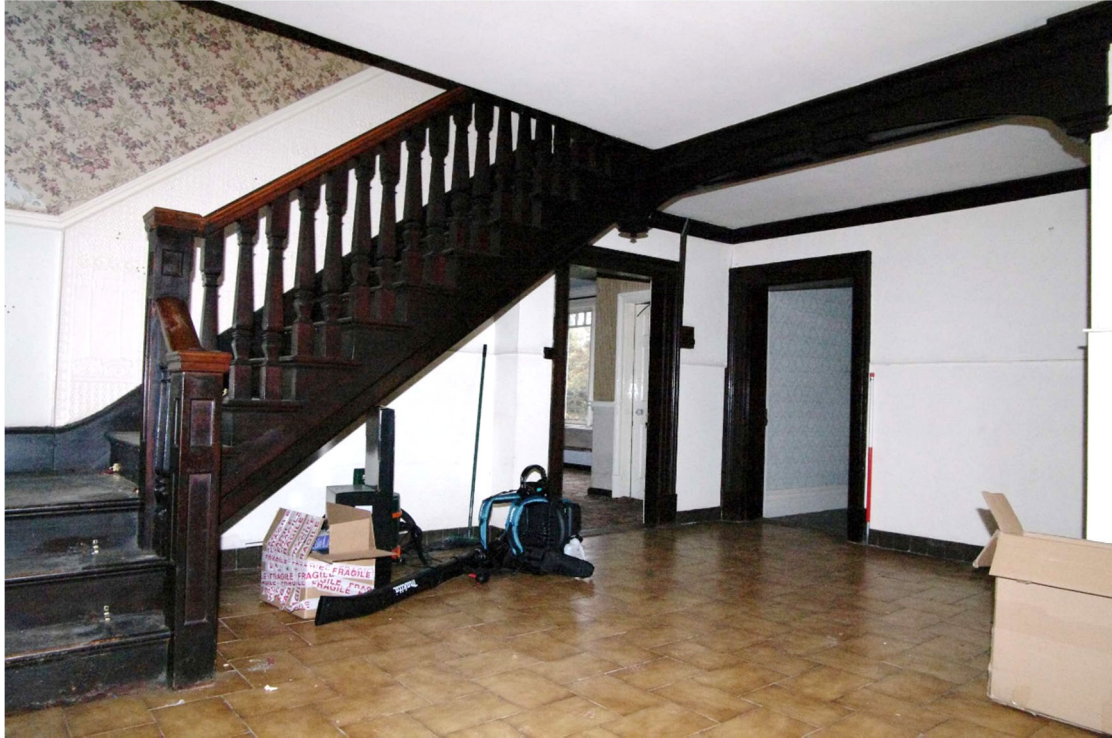
Figure 32 Main hall and stairs Looking east. 1m scale
