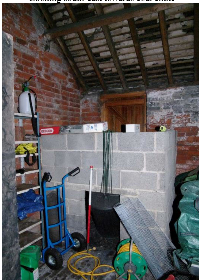
Figure 21 Breeze block coal bunker in store Looking south. 1m scale
