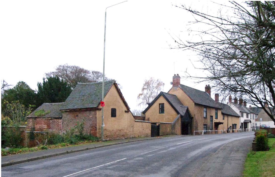
Figure 6 View from Main Street Looking south. Outhouses in foreground
