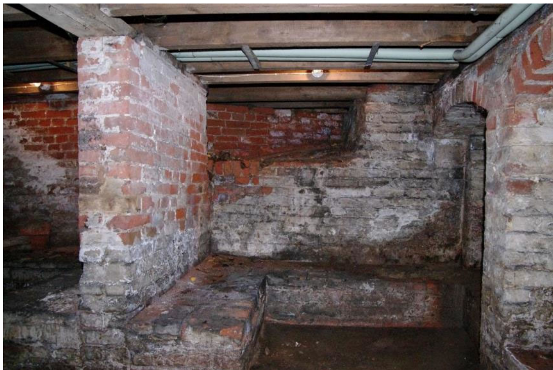
Figure 20 Cellar Looking south-east towards coal chute
