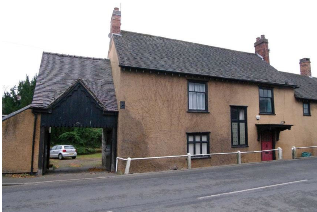
Figure 10 Covered gateway and main body of house Viewed from Main Street looking south. Note low level of doorway compared to the road level
