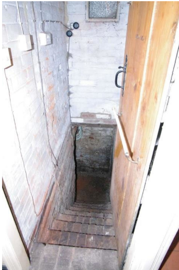
Figure 19 Cellar stairs from kitchen Looking south-east
