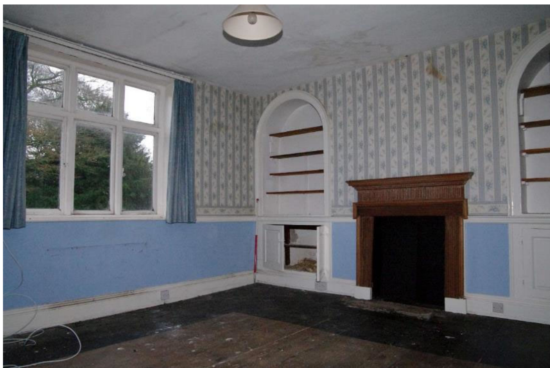
Figure 49 First floor rear bedroom above reception room Looking south. 1m scale
