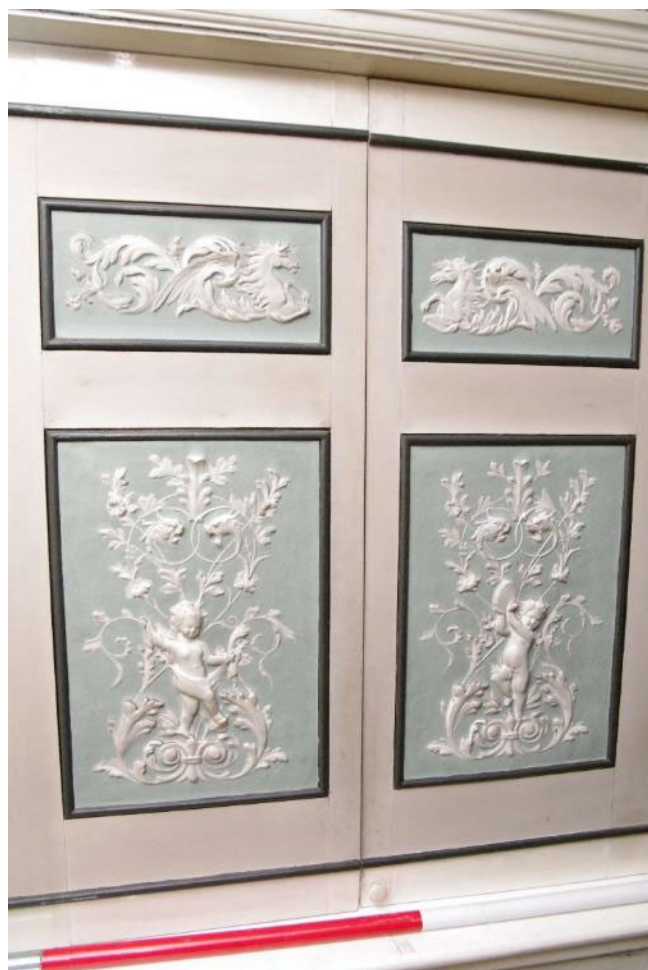
Figure 36 Living room window shutters Looking north-west. 1m scale
