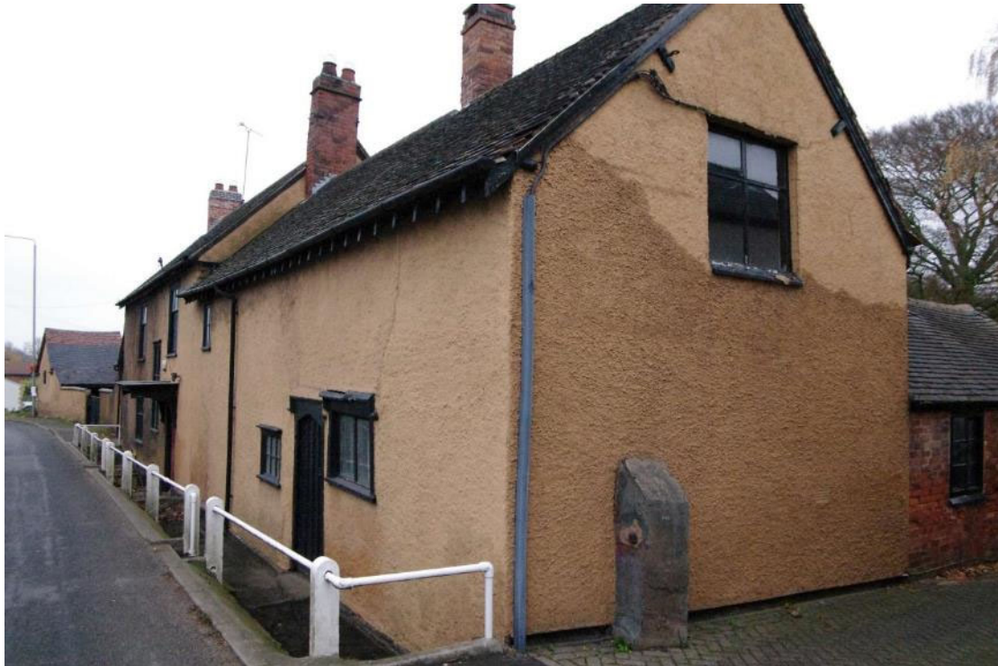
Figure 12 South-west facing gable end of house Looking north-east along Main Street
