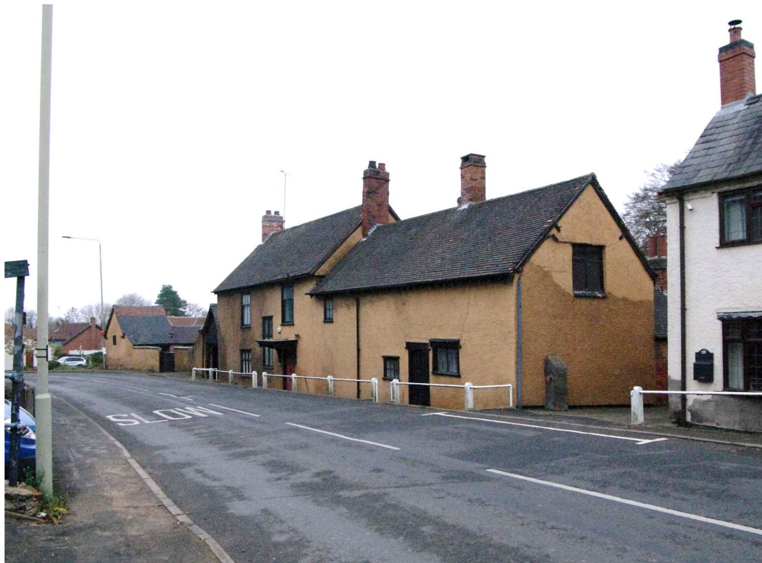
Figure 7 View from Main Street Looking north-east
