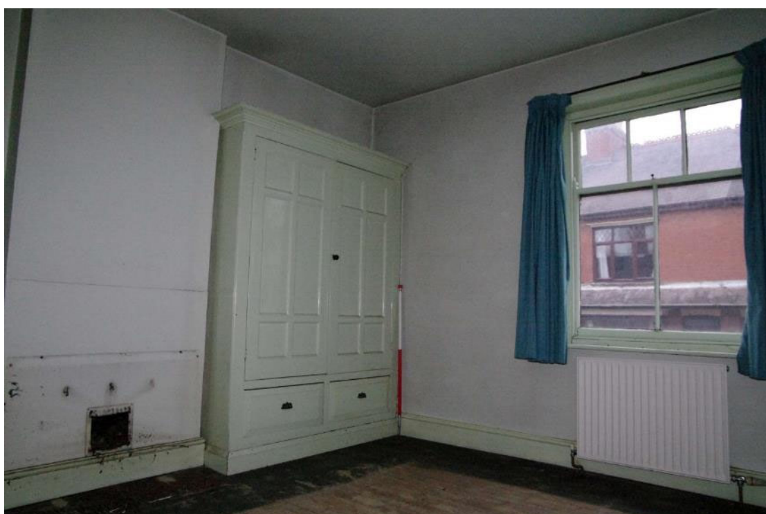
Figure 48 First floor bedroom above ground floor hall Looking west. 1m scale
