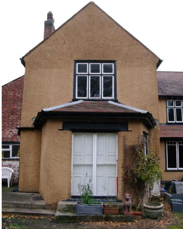
Figure 16 Rear extension and later 3-sided addition Looking north-west. 1m scale
