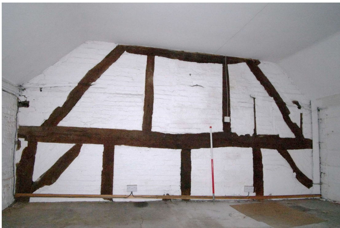
Figure 40 First floor western end room Looking north-east. 1m scale
