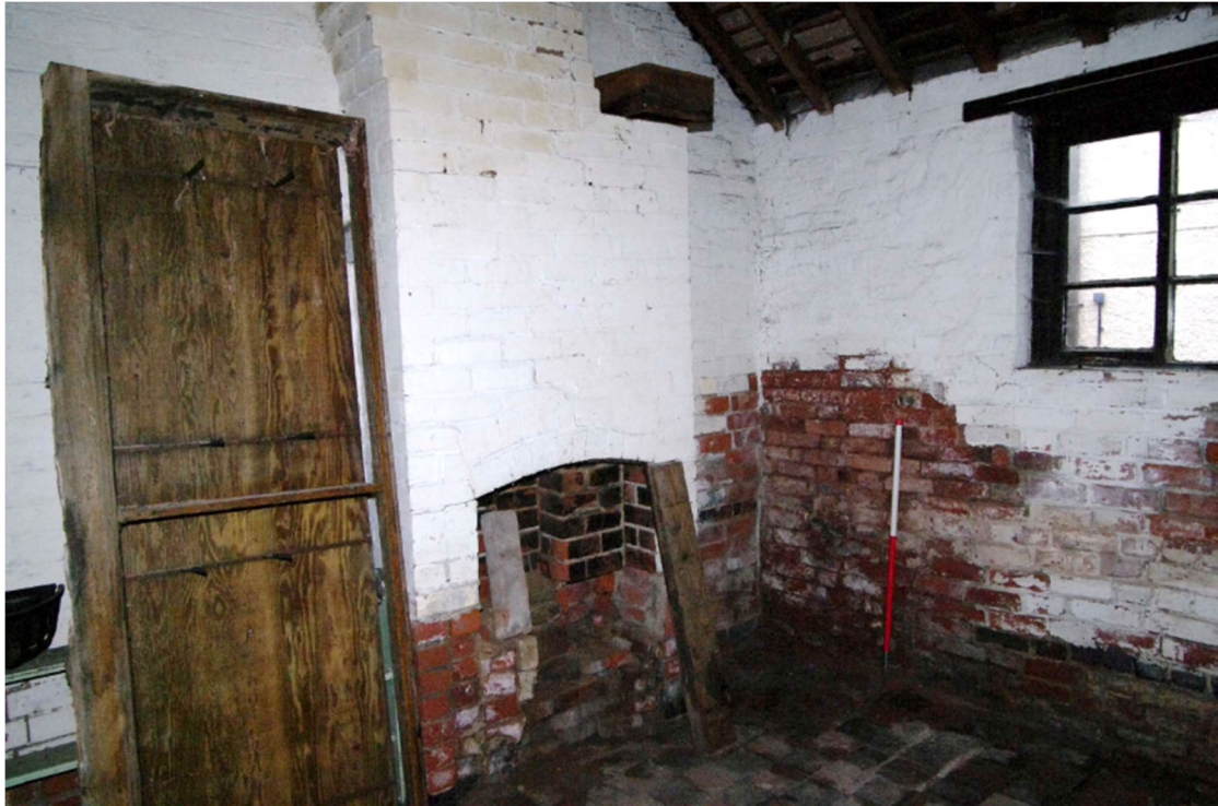
Figure 22 Former wash house Looking south. 1m scale
