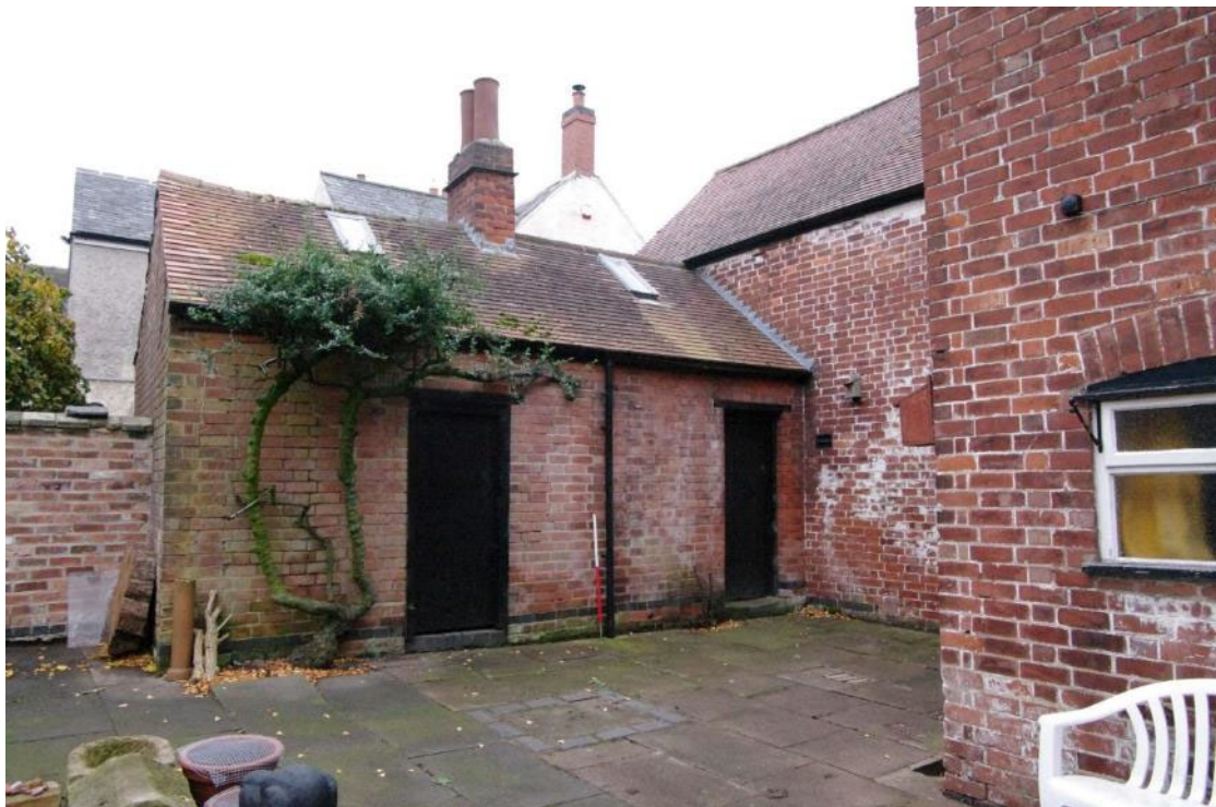
Figure 15 Former store and wash house Looking south-west. 1m scale
