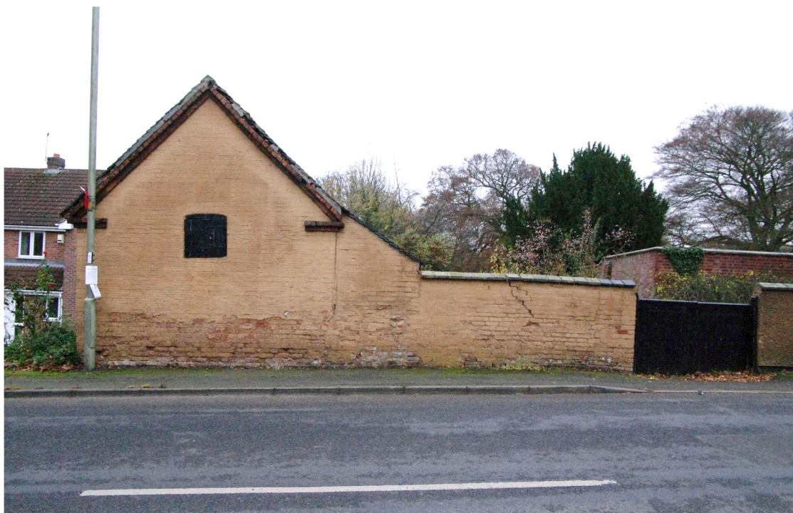
Figure 8 Outbuilding wall facing onto Main Street Looking south-east
