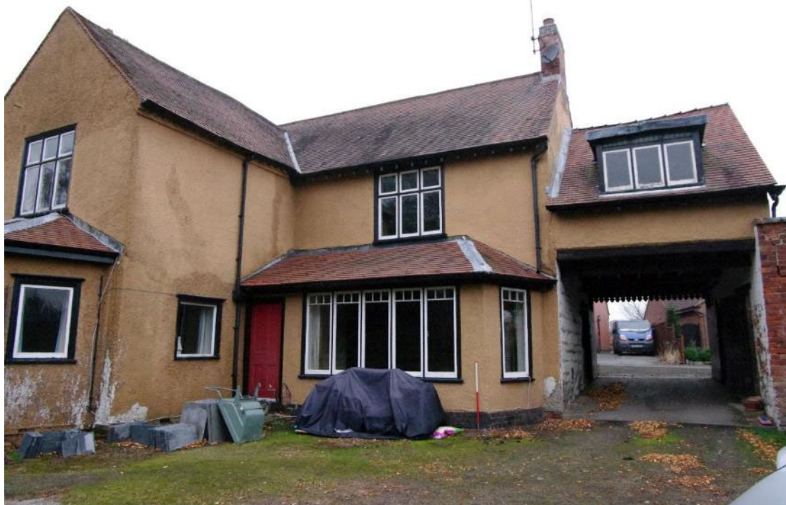
Figure 17 Rear of house and covered gateway Looking west. 1m scale
