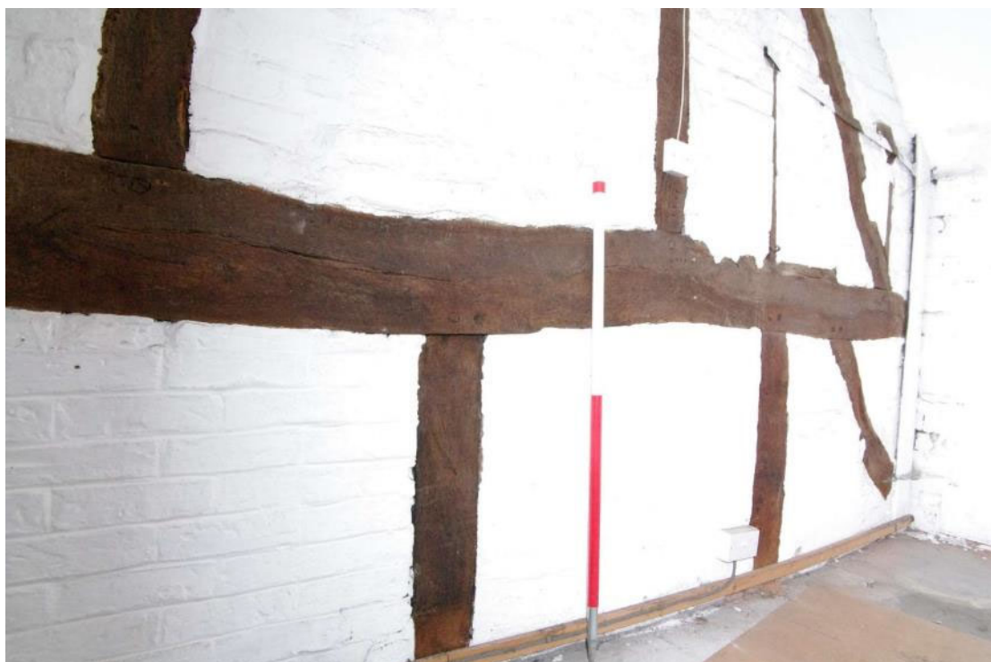
Figure 41 First floor western room timber-frame detail Looking east. 1m scale
