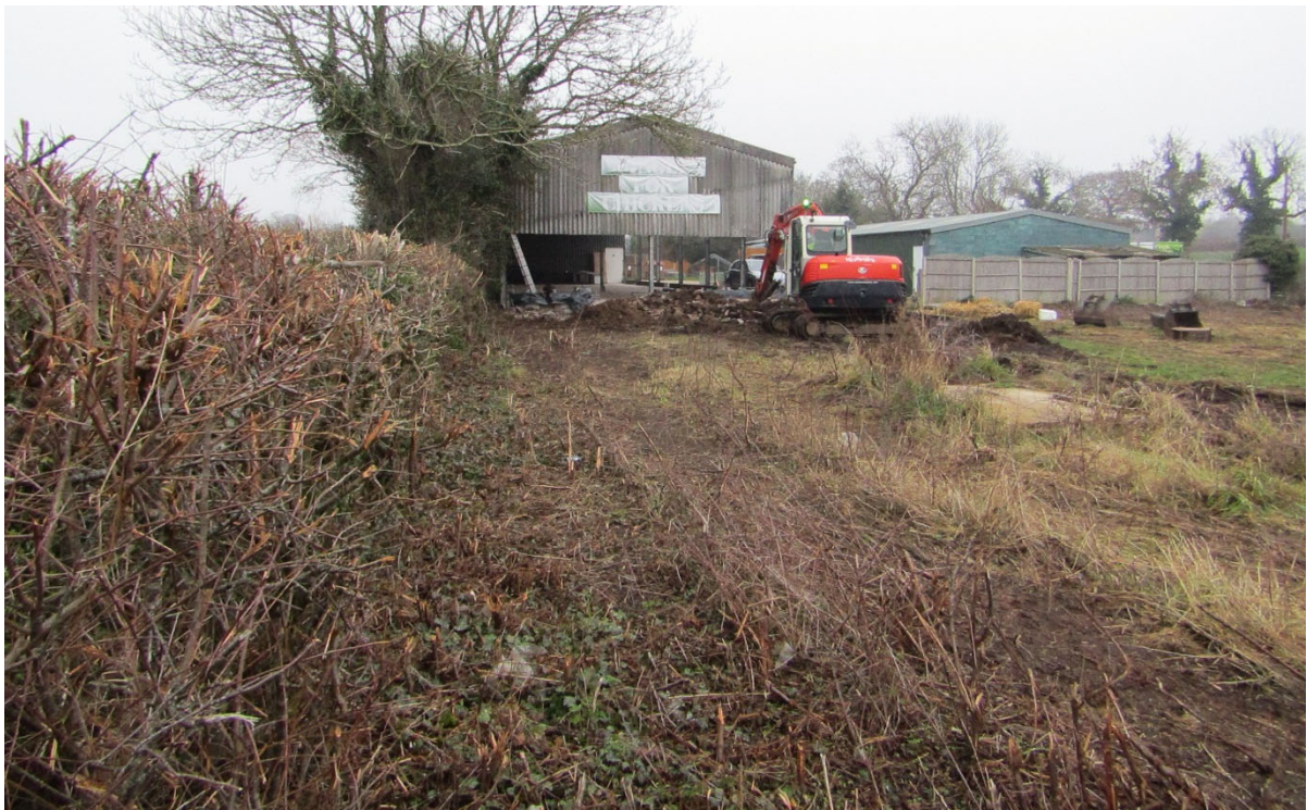
Figure 5 Area of groundworks, note remains of heavy vegetation cover.
