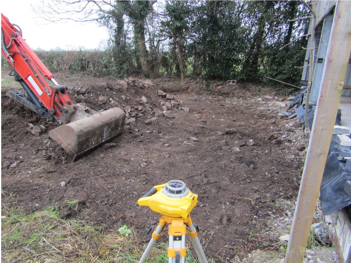
Figure 4 Spread of modern rubble to immediate south of modern barn.
