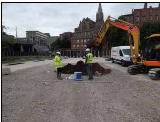
Figure 8 Trial Pit 11 looking North
