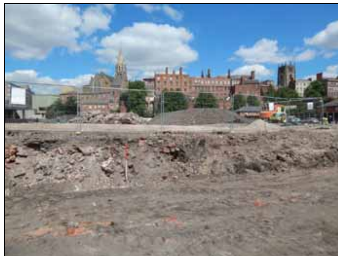
Figure 11 Ground reduction Zone 1 looking north
