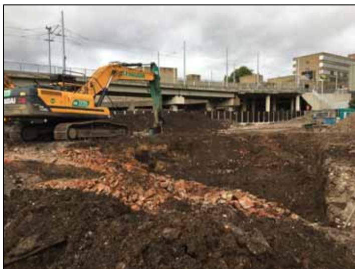
Figure 17 Ground reduction Zone 3
