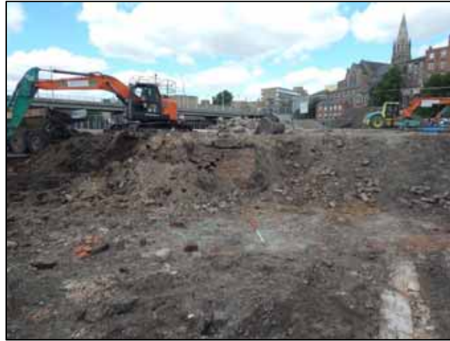
Figure 10 Ground reduction Zone 1 remnants of brick cellars
