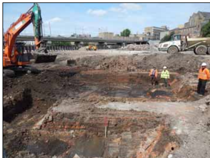
Figure 15 Top of viaduct brick and concrete foundations Zone 1 looking north-west
