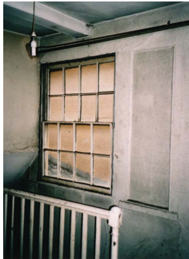
Plate 6 Detail of two parts of the tripartite window set at the head of the staircase rising from second to third floor. The eight-over-eight sash window is the central feature and the section to the right originally had a narrower four-over-four fixed window, now blocked.
