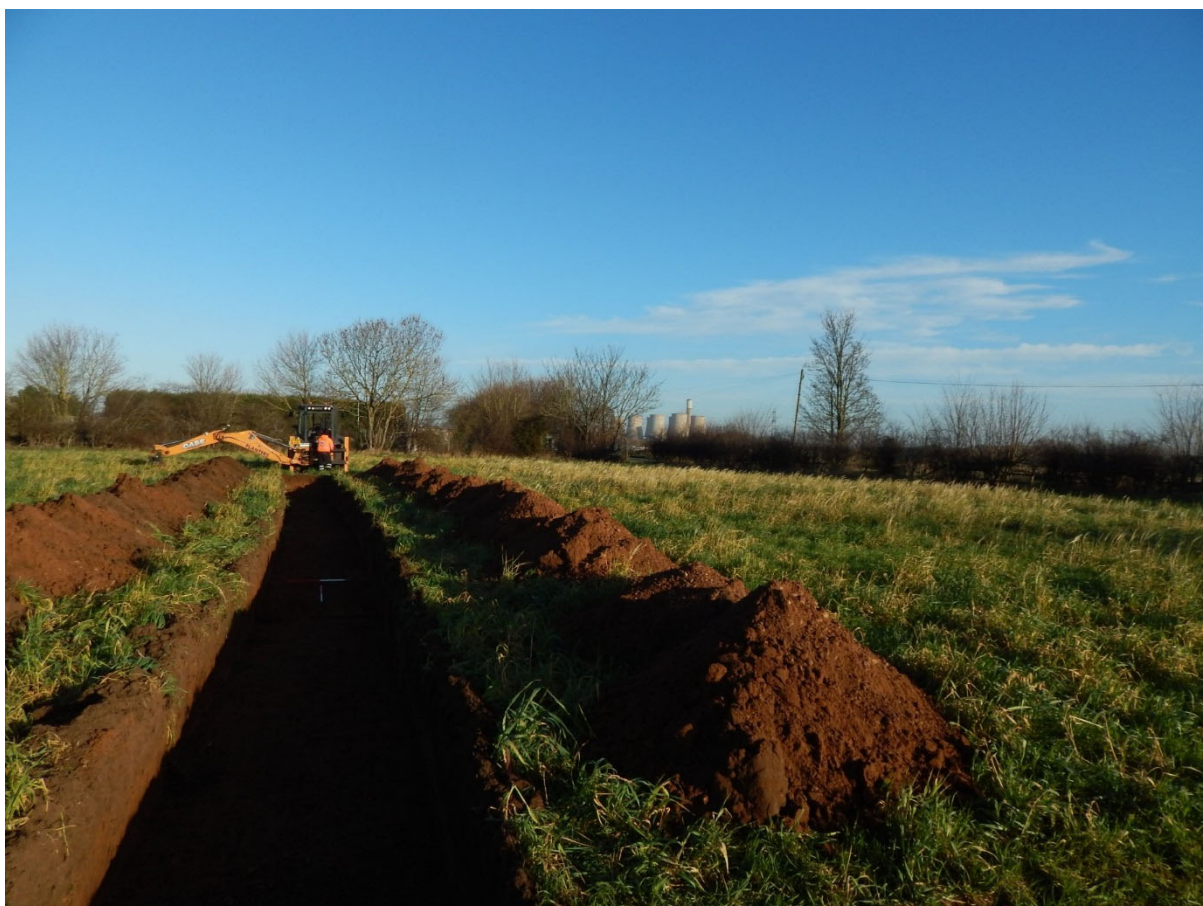
Figure 4: Work in progress on Trench 01, looking north
