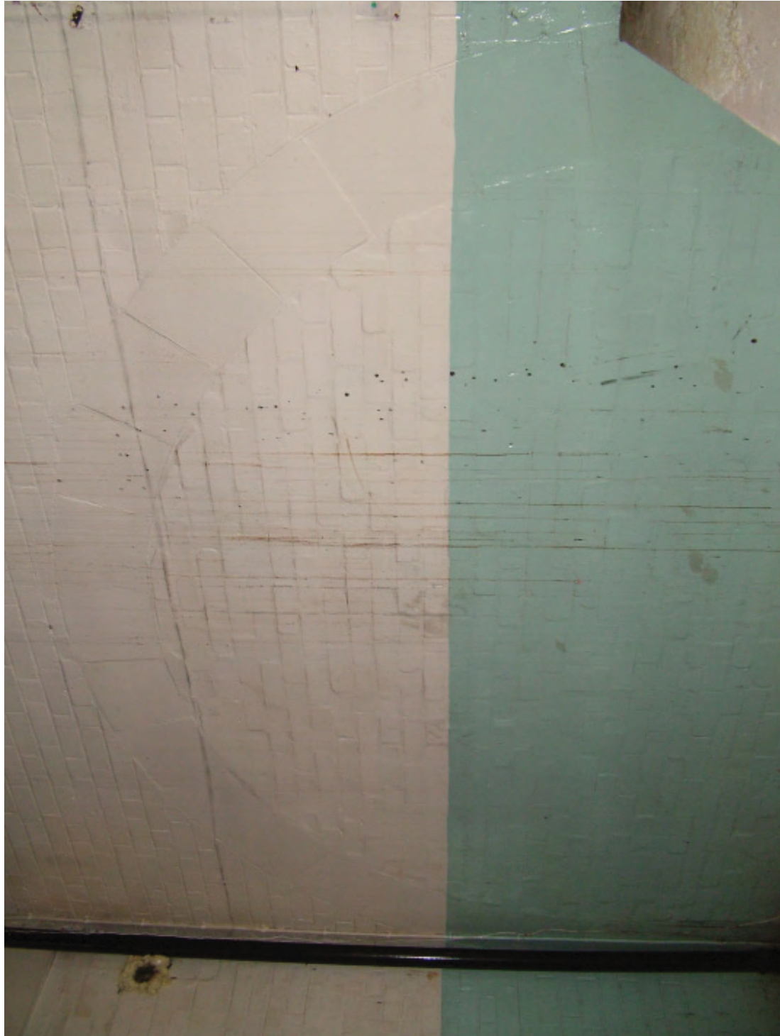
Plate 16: Detail of blocked arch for drive-through loading bay
