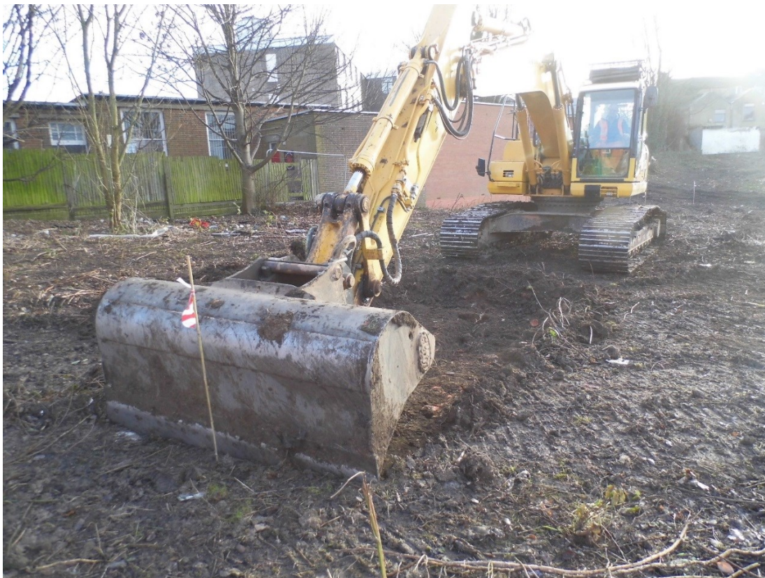
Figure 4: Excavation of the trenches.
