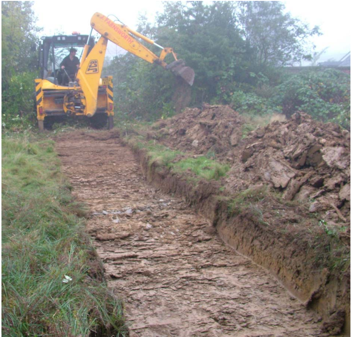
Plate1: Machine stripping trench C. West Facing
