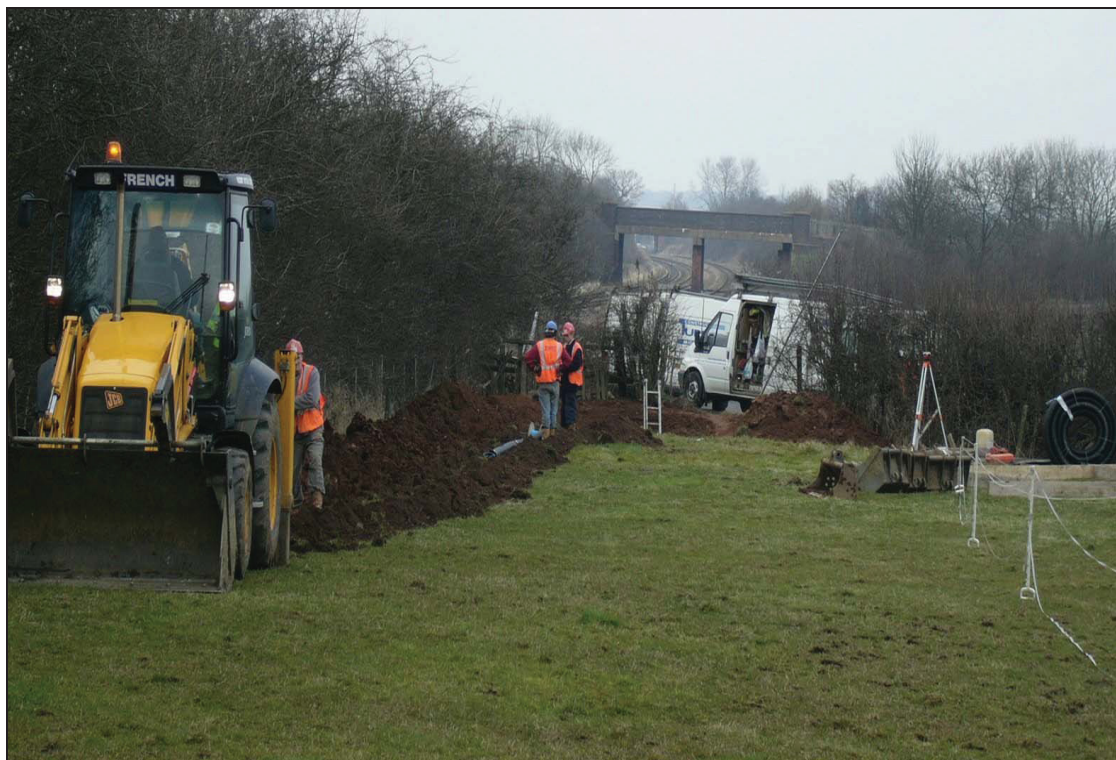
Plate 1: General view south along cable trench towards mast base
