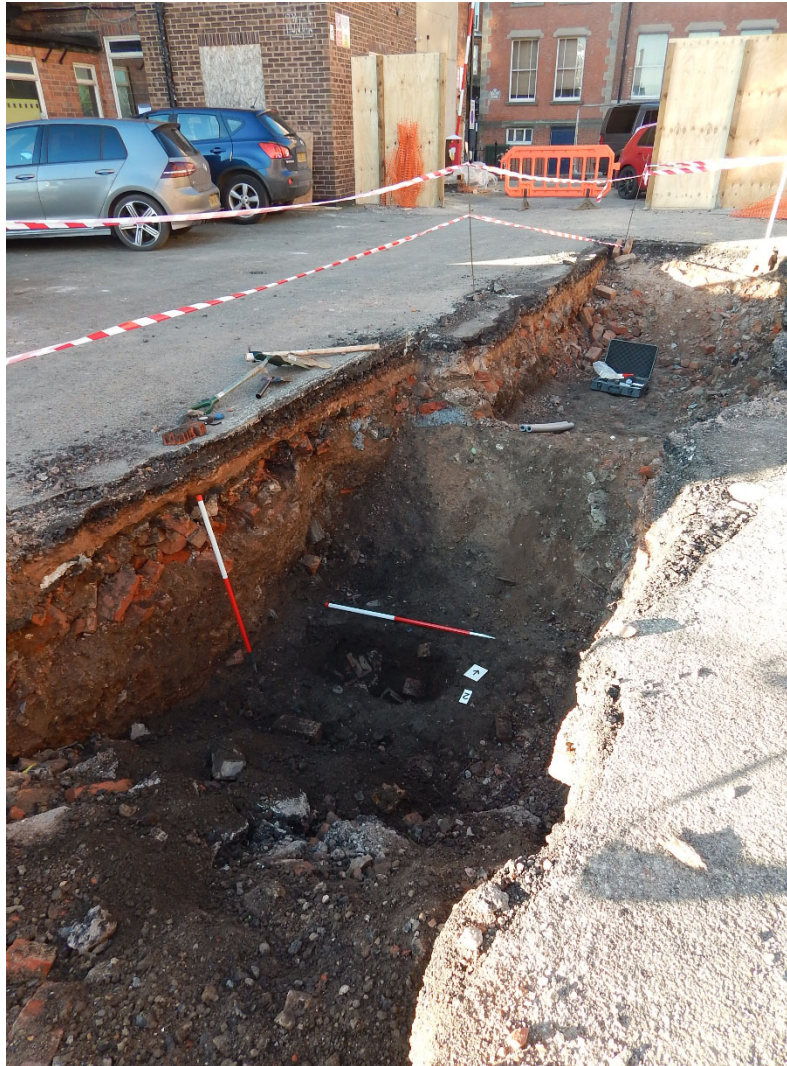
Figure 10 Trench 2 looking north-west
