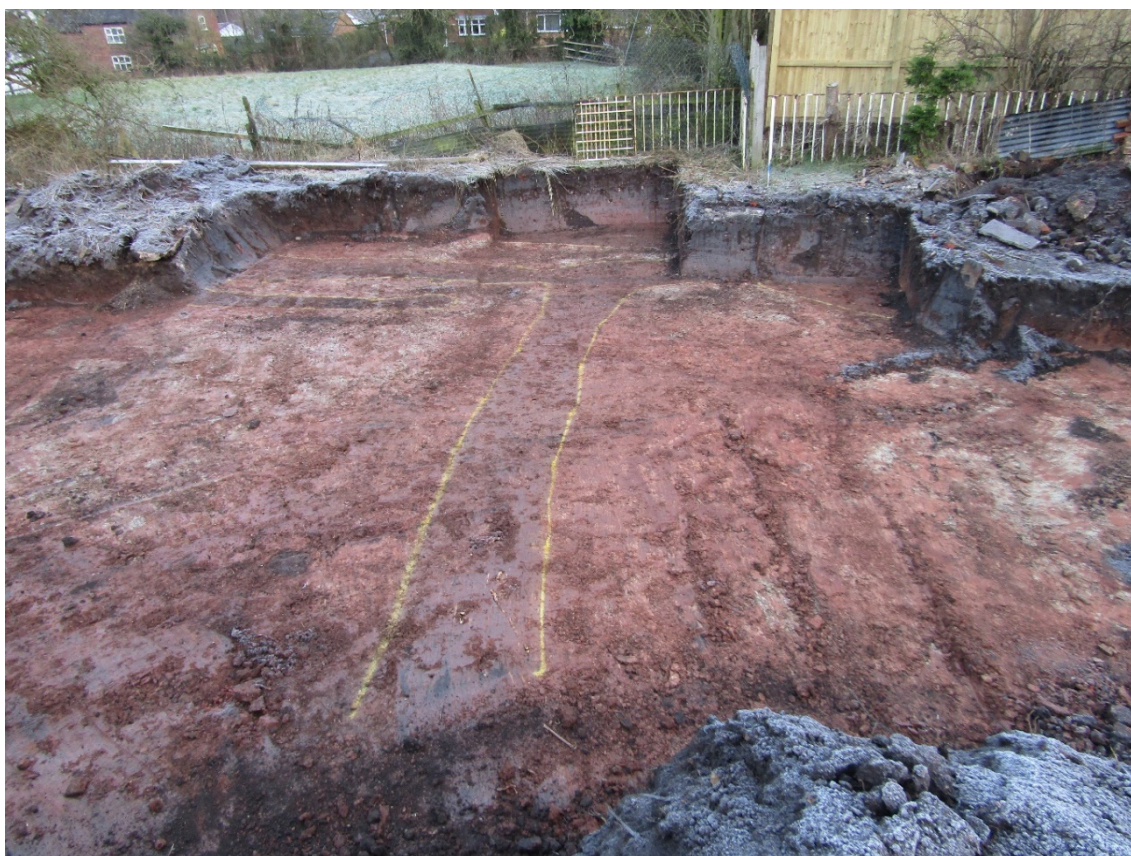
Figure 9: Centre of site prior to excavation, looking north.
