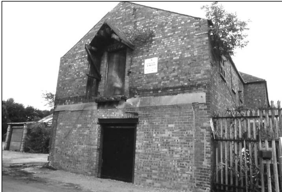
Plate 6. South-west facing elevation. Looking north
