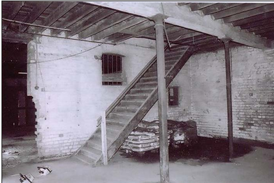
Plate 9. Staircase leading from ground to first floor. Looking south-west.
