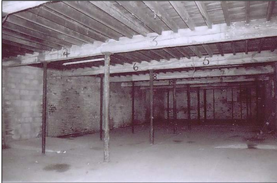
Plate 7. Ground floor, main warehouse. Looking north.
