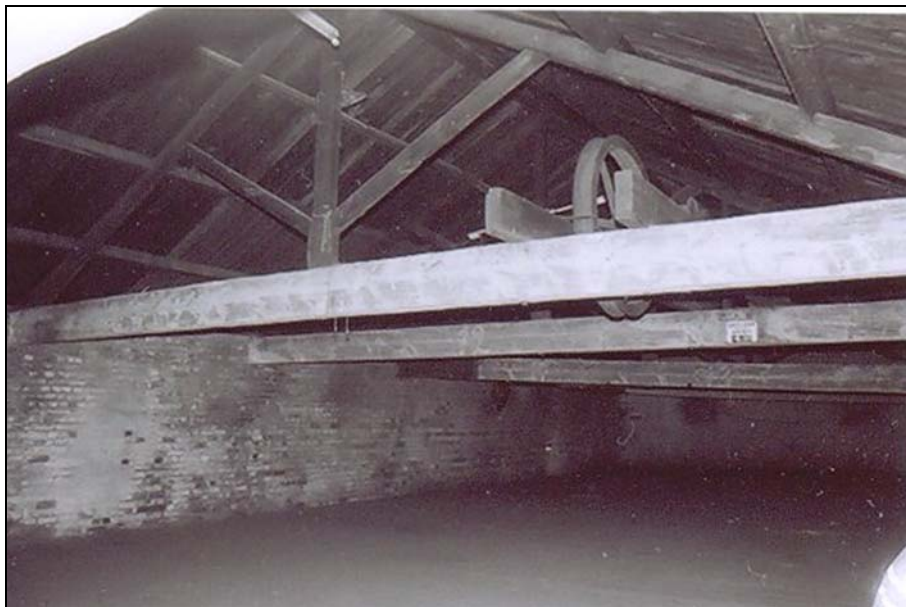
Plate 10. First floor roof structure, main warehouse. Looking north-east.
