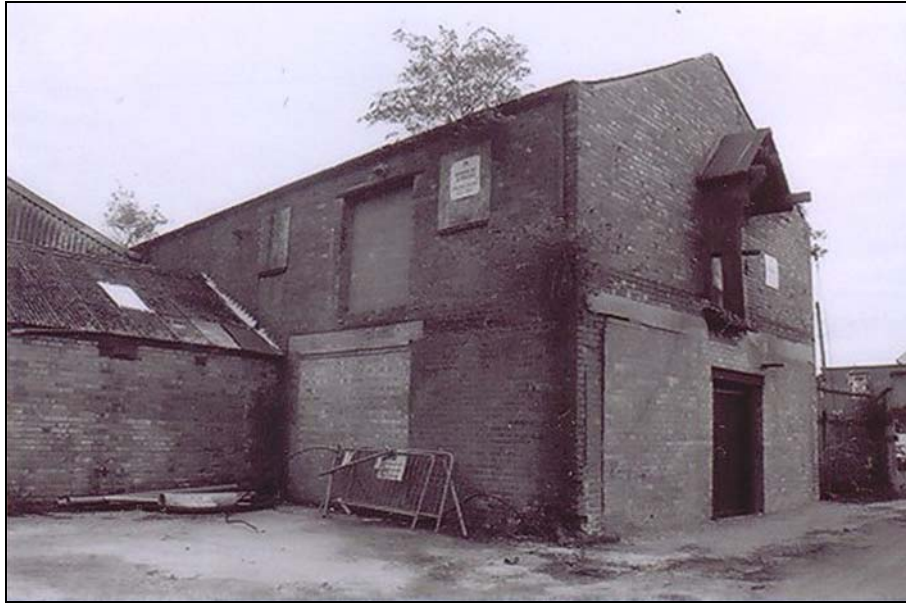
Plate 5. Rear elevation of warehouse annexe. Looking east.
