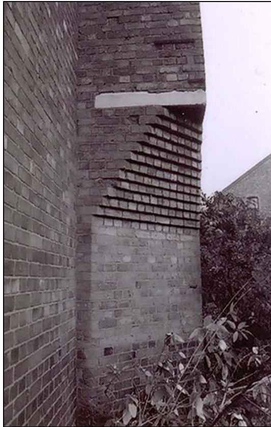
Plate 3. Chamfered corner between main warehouse and annexe. Looking north-east.
