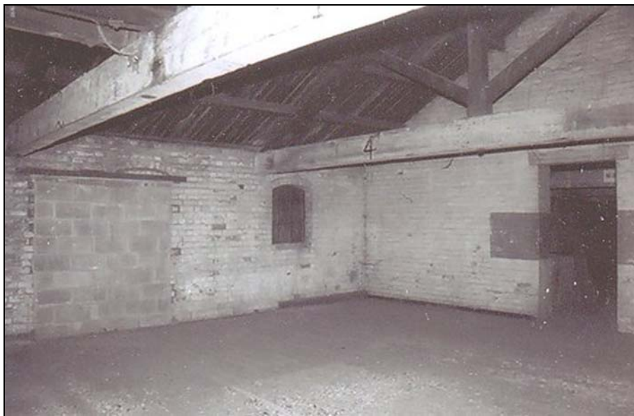
Plate 12. First floor warehouse annexe. Looking north.
