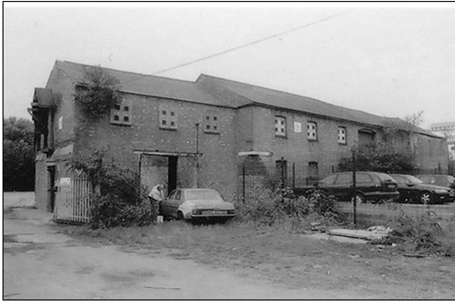
Plate 1. Frontage elevation. Looking north
