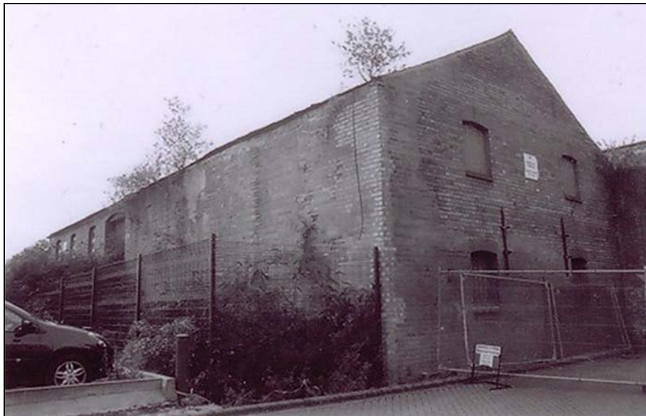
Plate 4. North-east facing gable end. Looking west.
