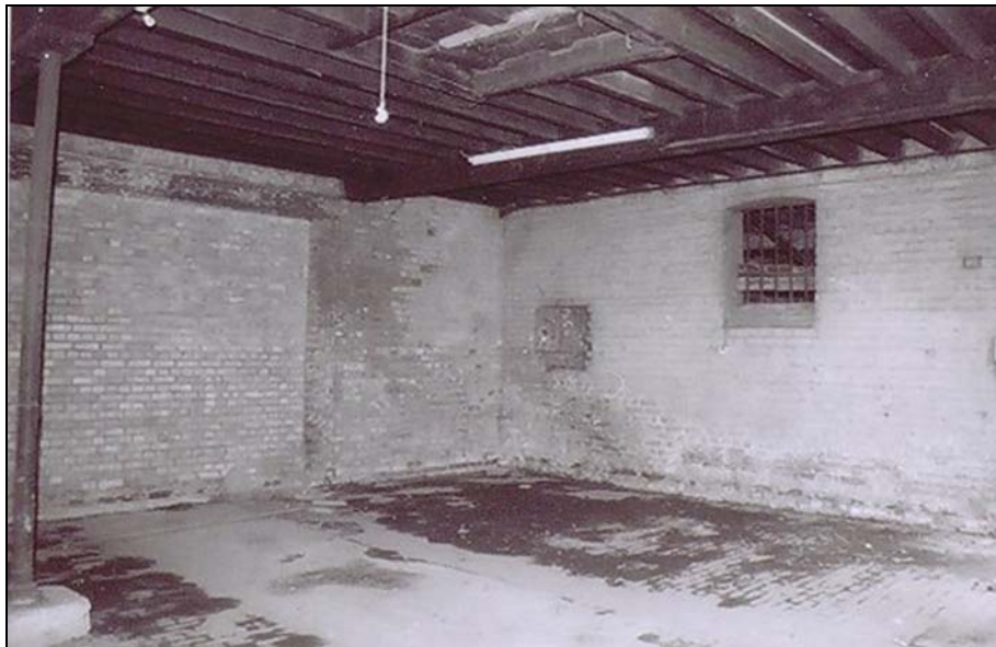
Plate 8. Ground floor, warehouse annexe. Looking north.
