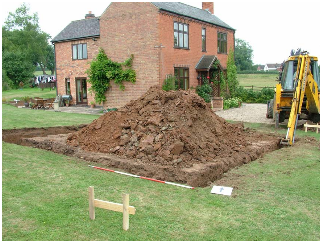
Figure 2 Working Shot of Ground Works (Looking NW)
