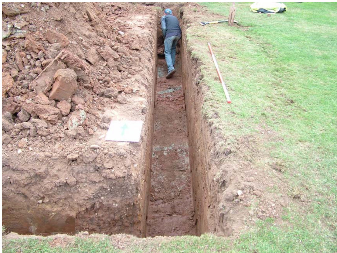
Figure 3 Working Shot Showing Foundation Trench (Looking North)
