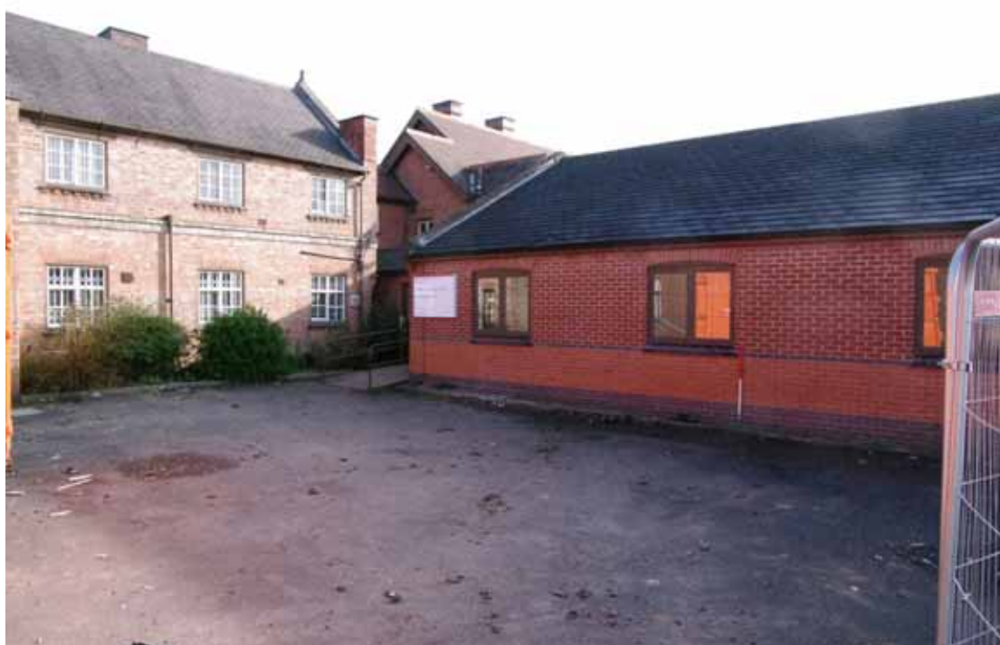
Figure 24 South-west facing elevation and link between blocks Looking east. Modern medical extension building on right
