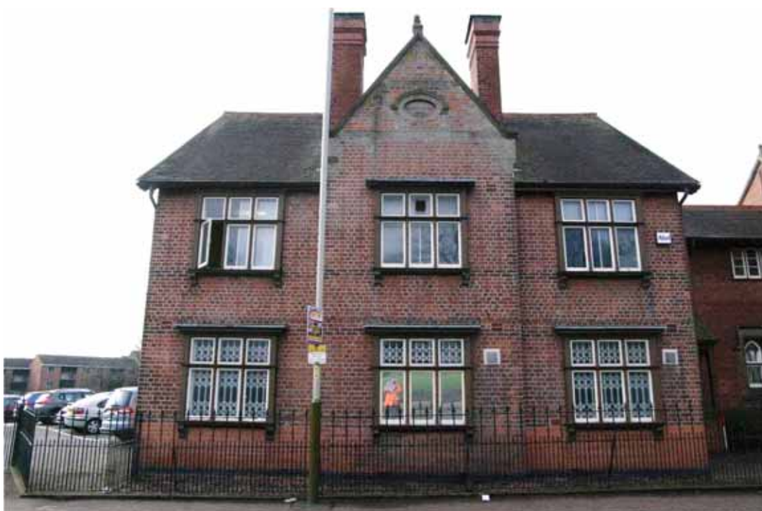
Figure 14 North-east facing elevation of 1893 block Looking south-west. Note faint diaper work between upper and lower windows
