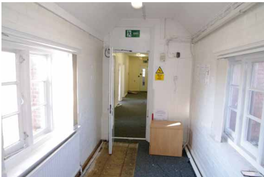
Figure 74 First floor link between 1856 and 1883 blocks Looking north-west towards corridor F14
