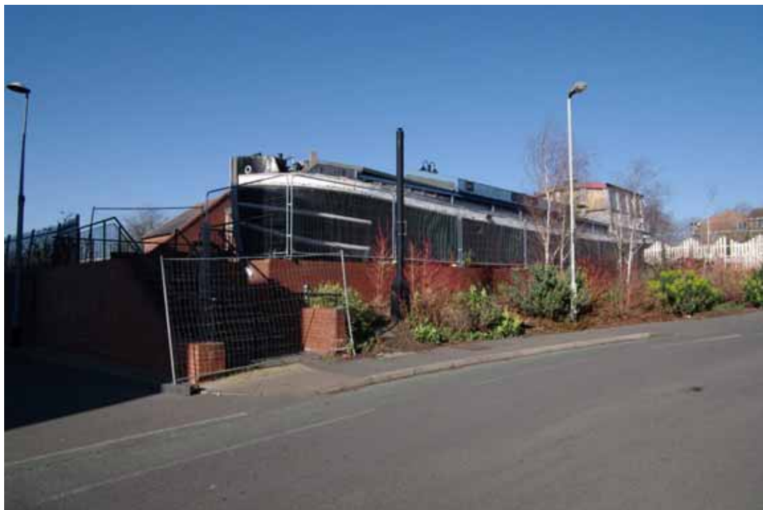
Figure 81 Dry Dock from road leading to Nixon Court Looking north-west
