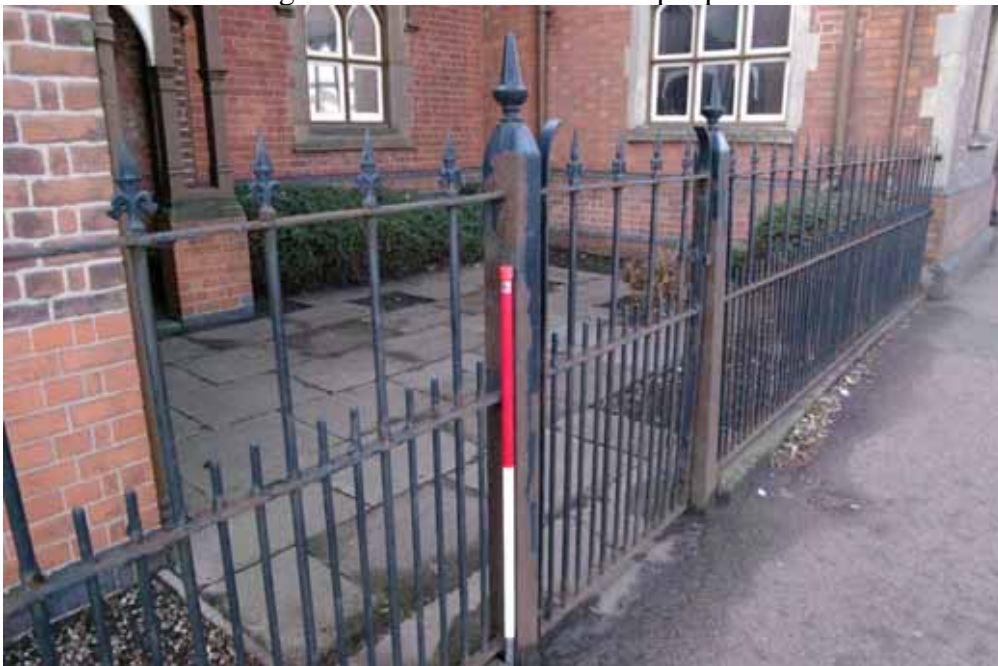
Figure 18 Railings in front of 1893 block Looking west. 1m scale
