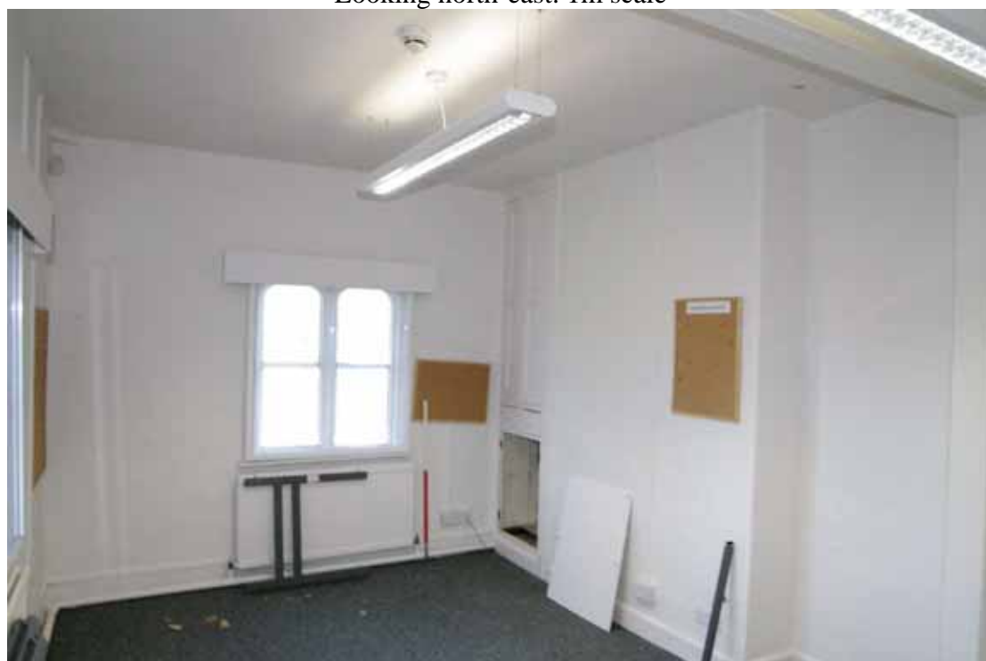
Figure 65 First floor 1856 block, Room F1 Looking north-east. 1m scale
