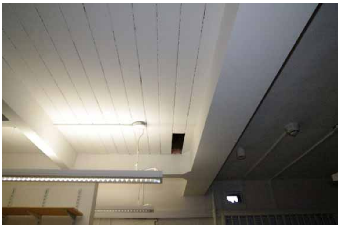
Figure 35 Room G1 wooden ceiling All ceilings elsewhere hidden by modern lowered ceiling
