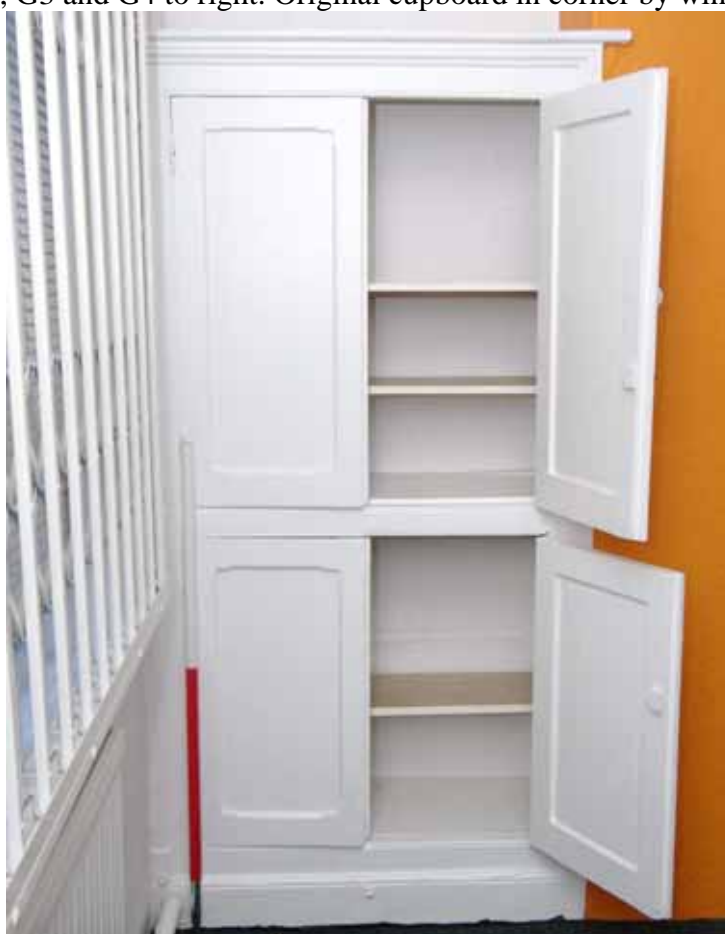
Figure 33 Room G1 cupboard Looking south-east. 1m scale
