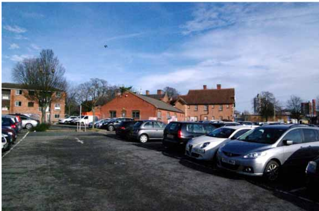
Figure 5 Freeman's Cottages and modern extension viewed from car park Looking north. Main University campus buildings in background on right
