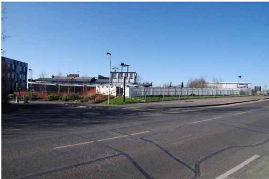
Figure 79 Dry Dock pub seen from Putney Road Looking south-west
