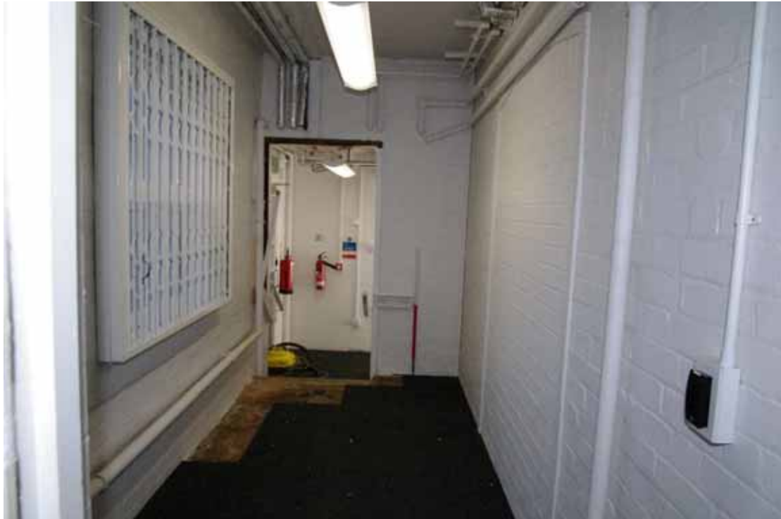
Figure 48 Link between 1856 and 1893 blocks Looking south-east towards 1893 block. Note infilled arch on right which has since been blocked by the modern medical building extension
