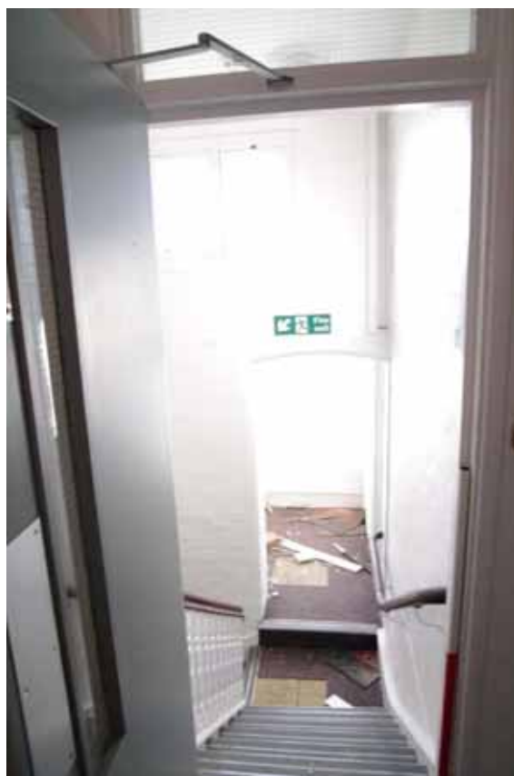
Figure 72 Stairs from corridor F10 Looking south-west
