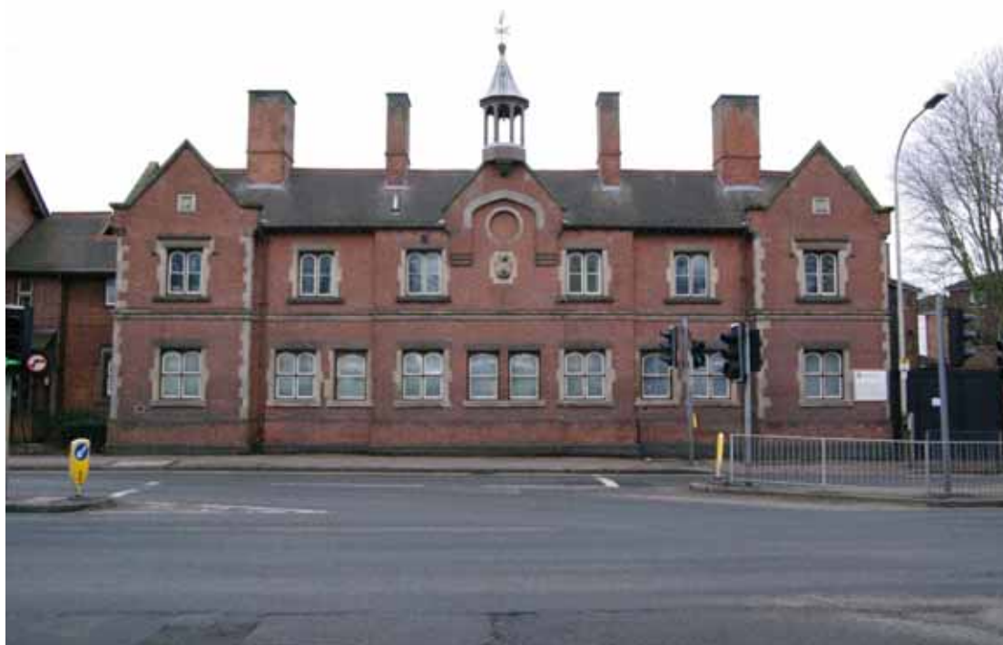
Figure 13 North-east facing elevation of 1856 block Looking south-west. Bell tower is an 1885 addition
