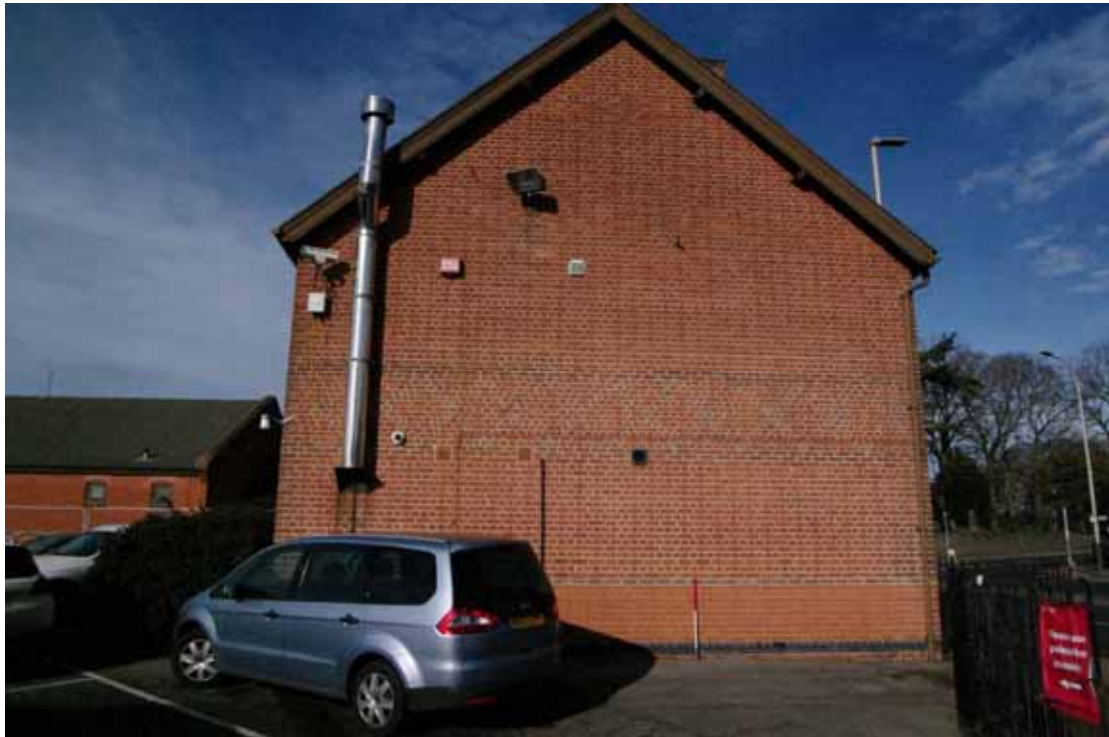
Figure 29 South-west facing gable end of 1893 block Looking north-west. 1m scale
