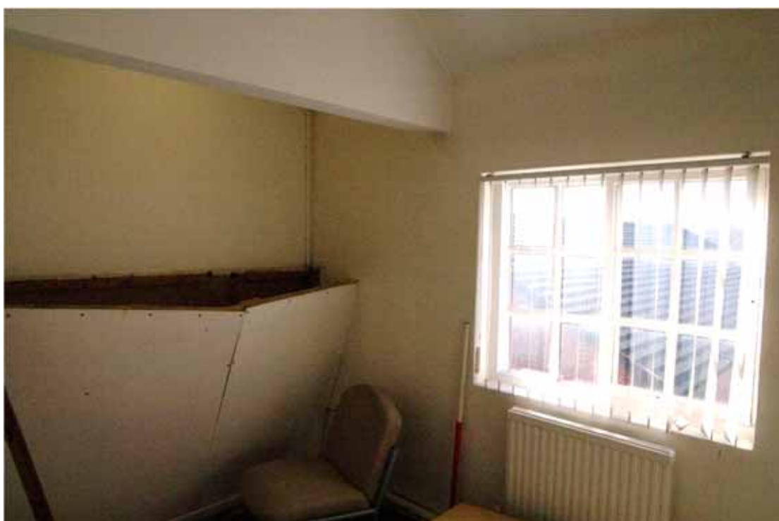
Figure 71 Room F12 Looking south. 1m scale
