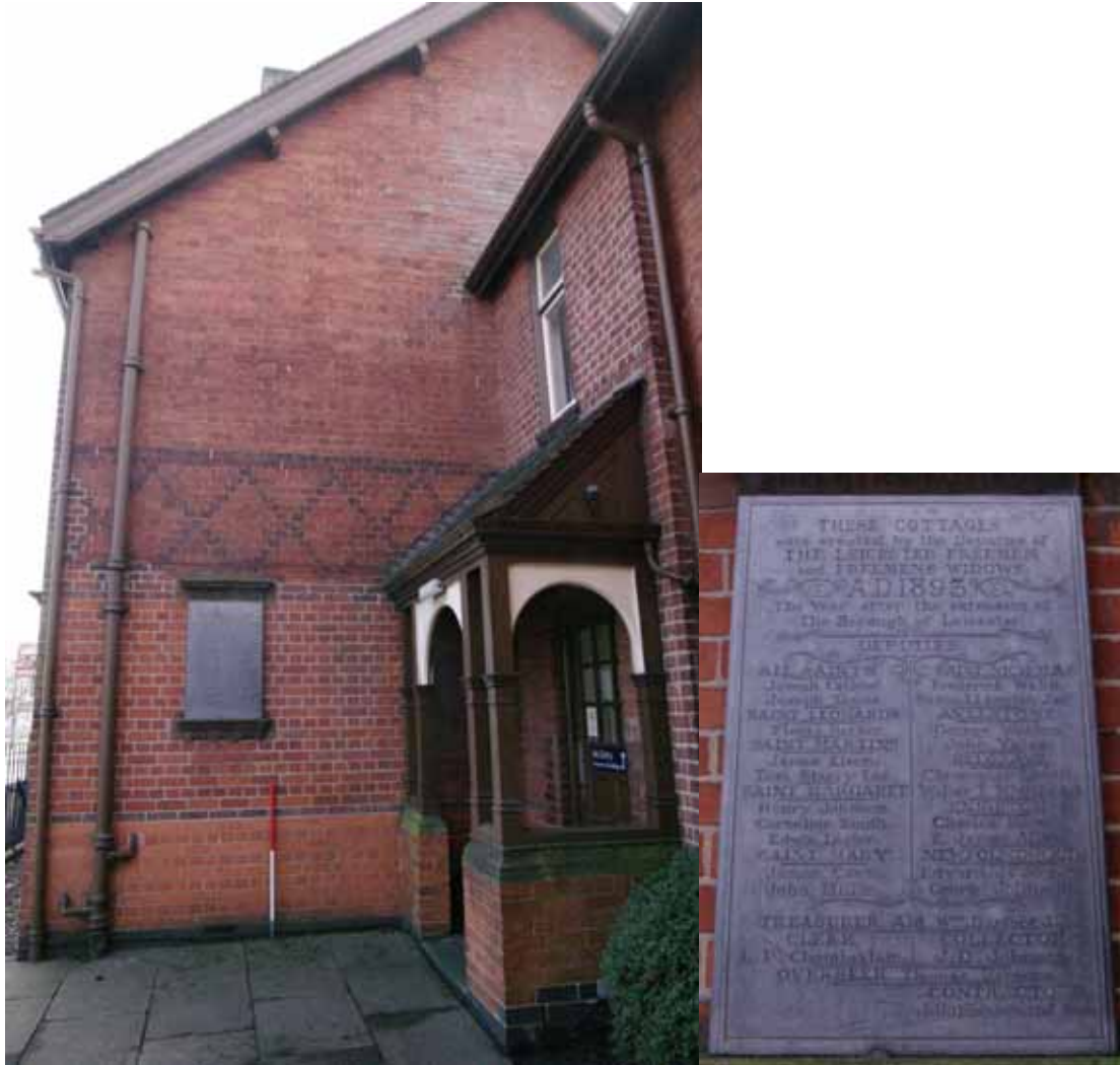
Figure 17 North corner of 1893 block Looking south-east. 1m scale. Inset: plaque detail
