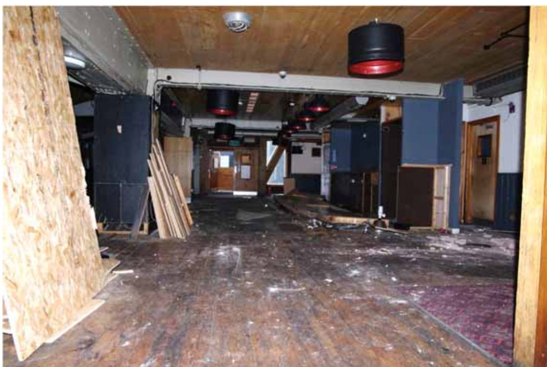
Figure 88 Bar area Looking south. Bar on right barge on left
