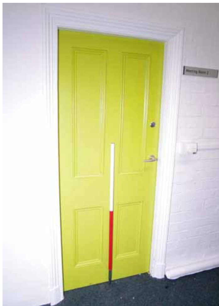
Figure 40 Door to Room G6 Looking south-west from G9. 1m scale
