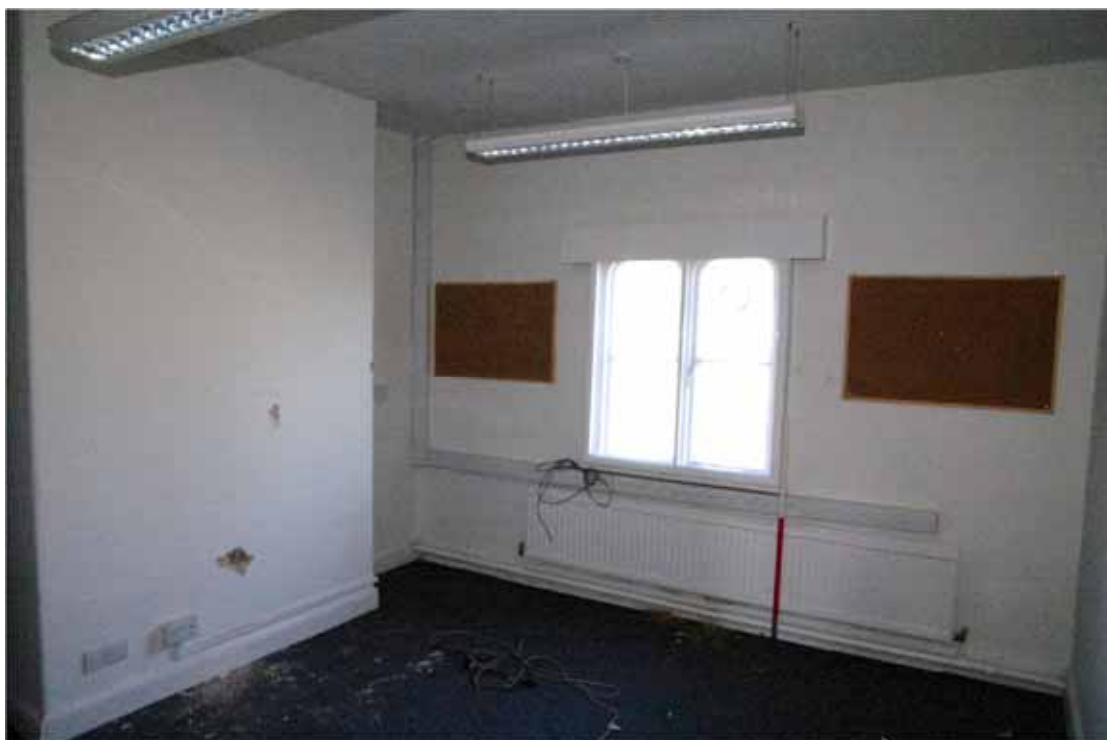
Figure 66 Room F2 Looking north. 1m scale
