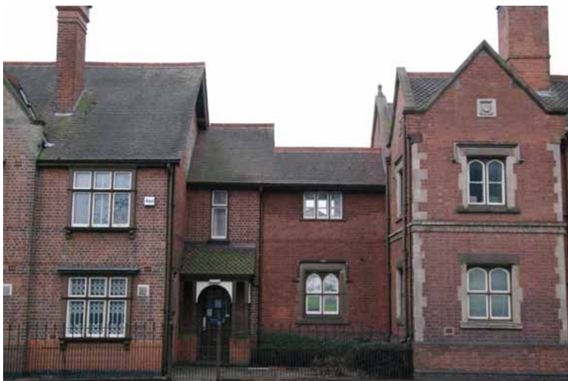
Figure 15 North-east facing link between 1856 and 1893 blocks Looking south-west
