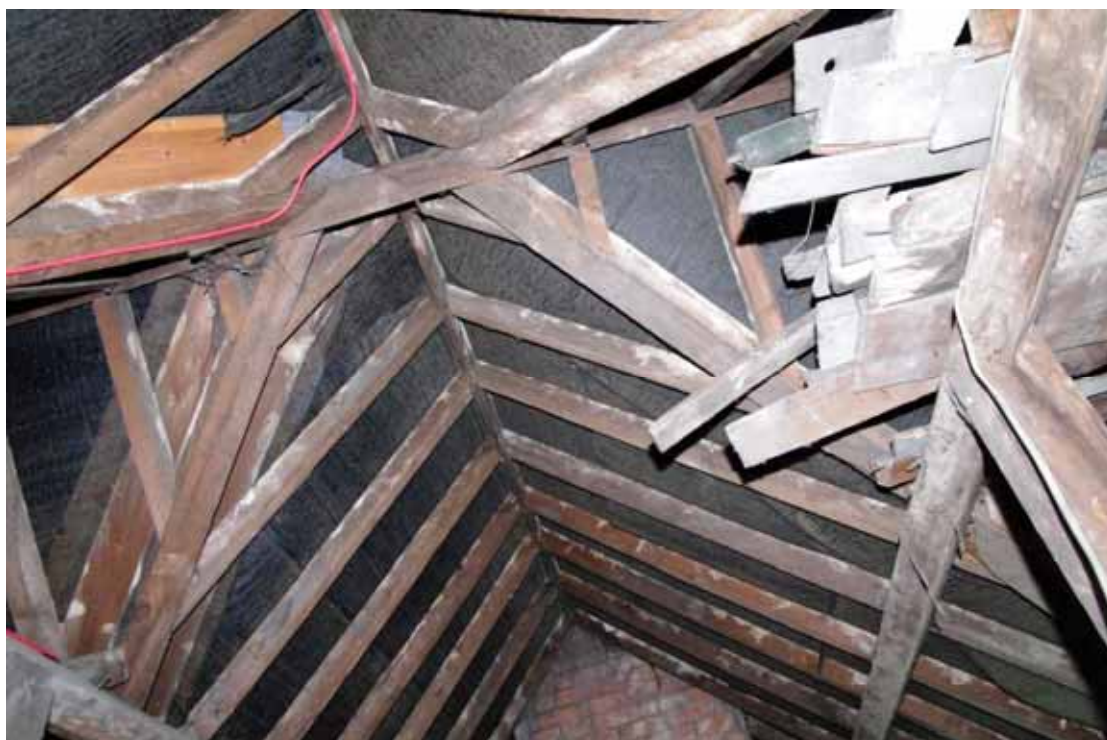
Figure 68 Roof structure seen from Room F4
