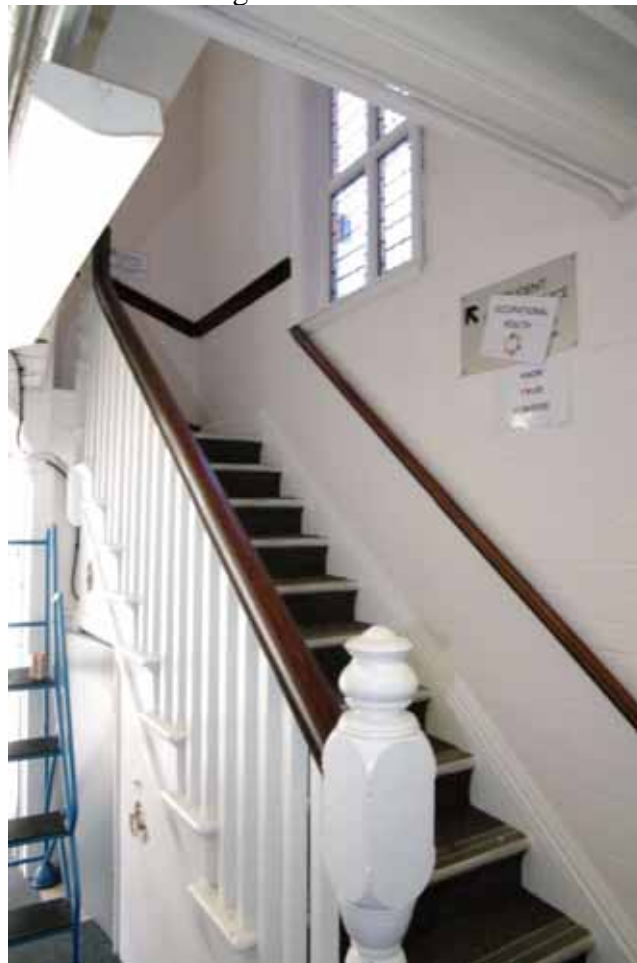
Figure 51 Link building stairs to first floor Looking west
