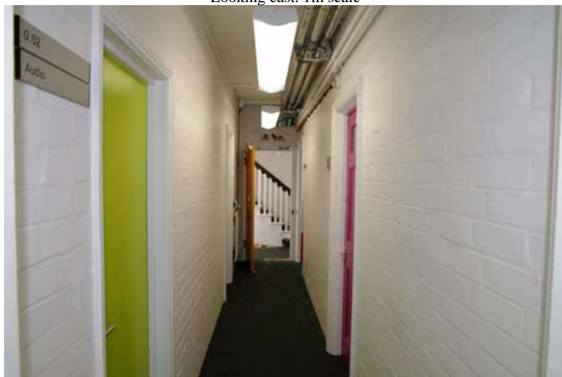
Figure 59 Corridor G22 Looking north-east towards stairs
