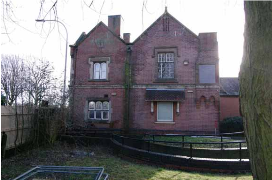
Figure 19 North-west facing elevation of 1856 block Looking south-east
