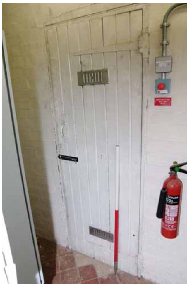
Figure 58 Room G21 store door Looking east. 1m scale
