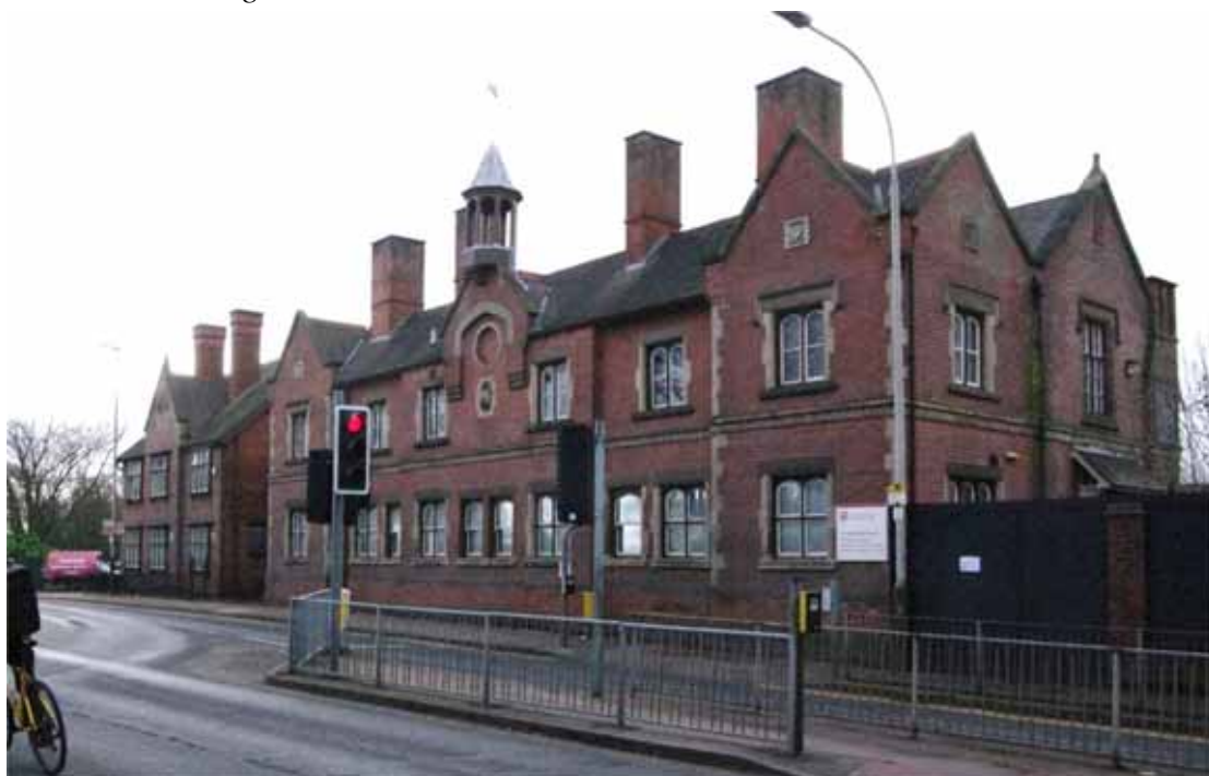
Figure 11 North-east facing elevation Looking south. 1856 block in foreground, 1893 block on left
