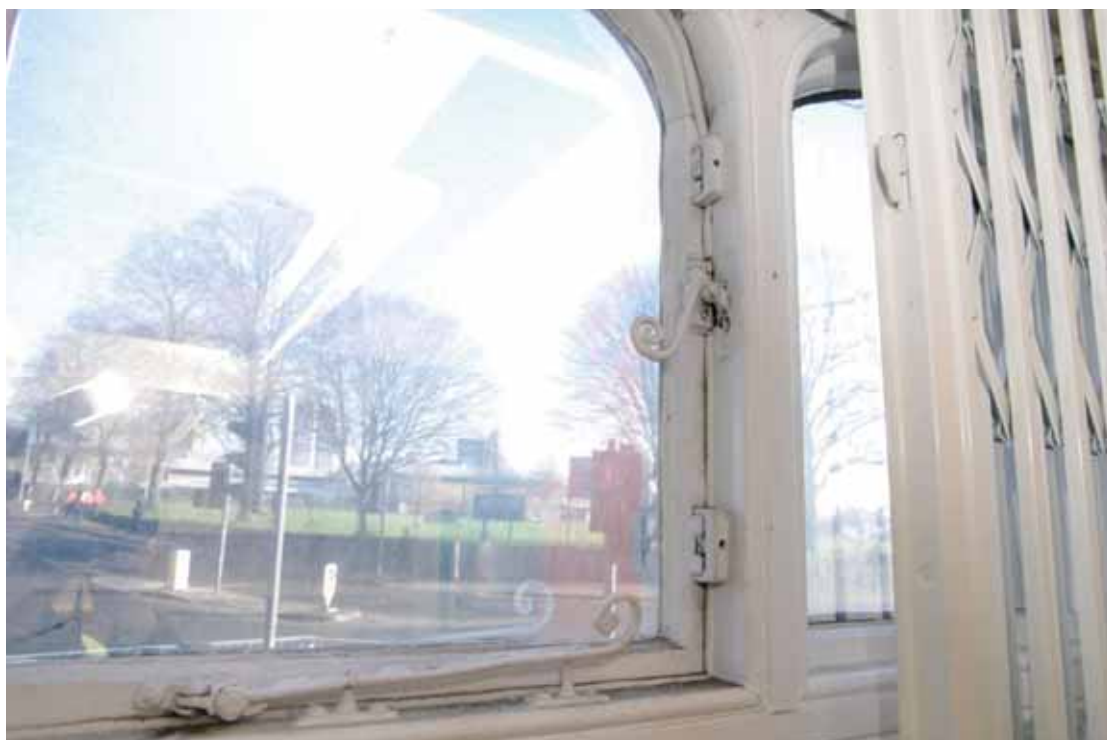
Figure 34 Room G1 window fittings Fittings vary from room to room
