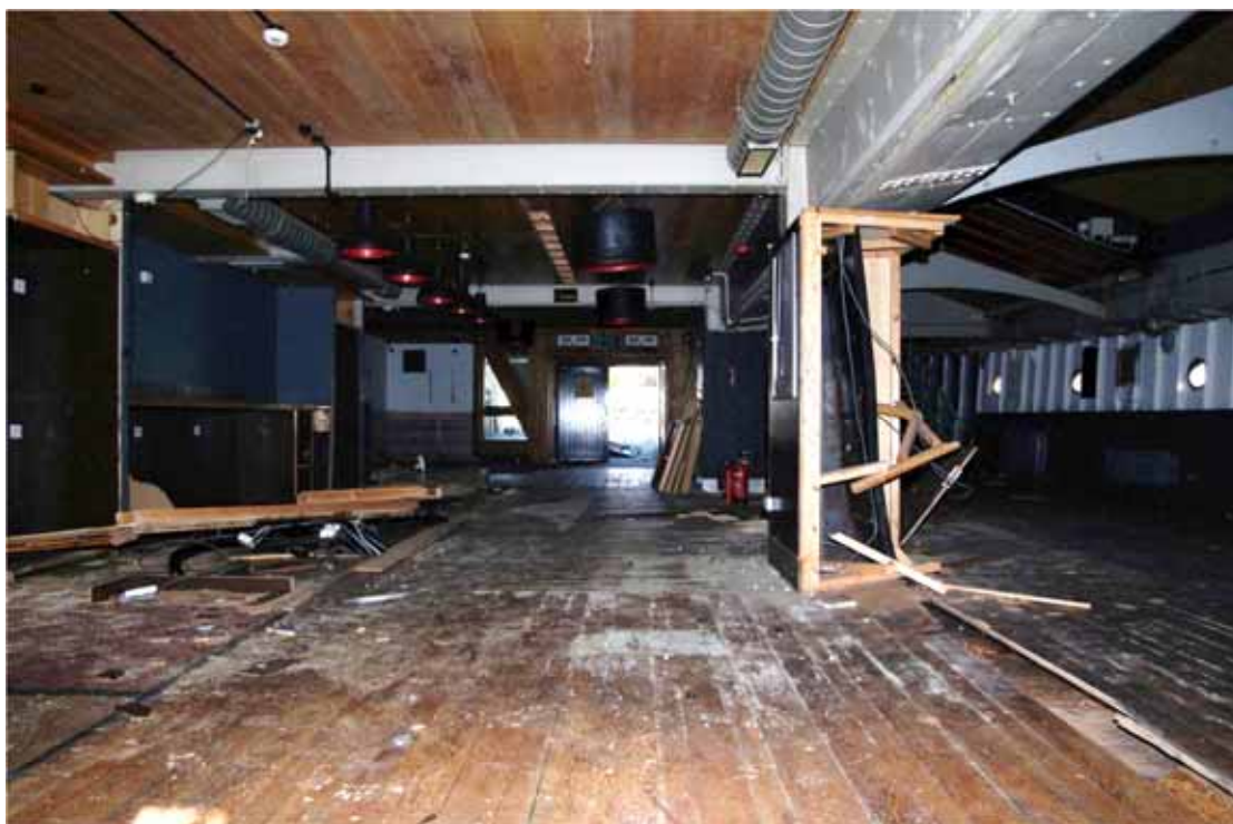
Figure 89 Bar area Looking north
