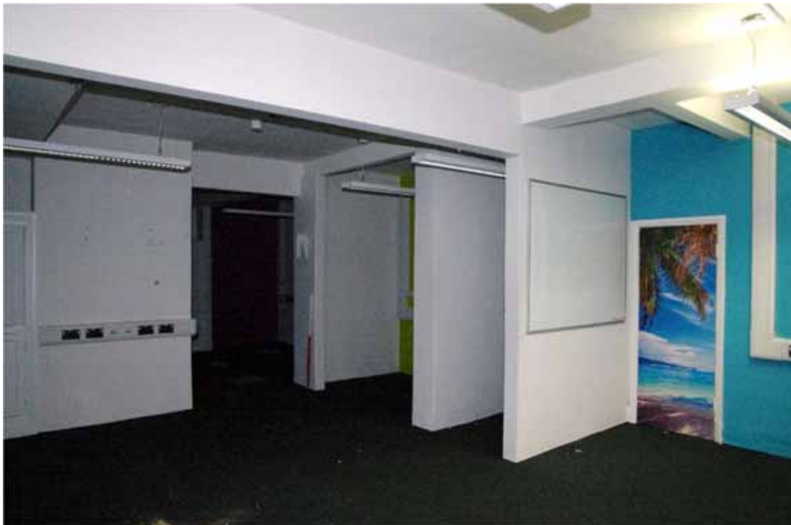
Figure 37 Rooms G3 and G4 Looking south showing stubs of original dividing walls and doors out to connecting corridor. 1m scale
