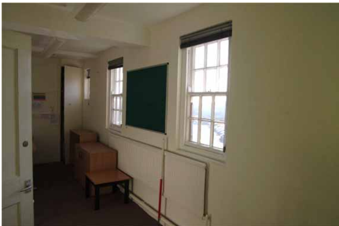
Figure 76 Room F20 Looking south. 1m scale
