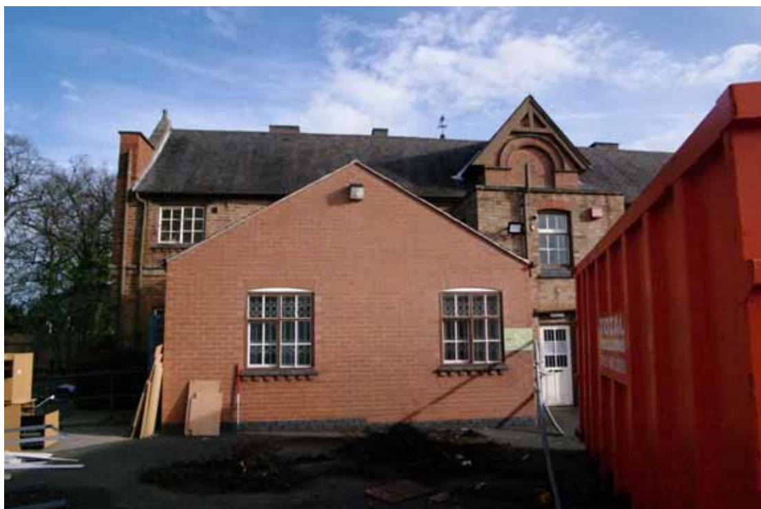
Figure 21 South-west facing elevation of 1856 block Looking north-east. Modern office extension in foreground
