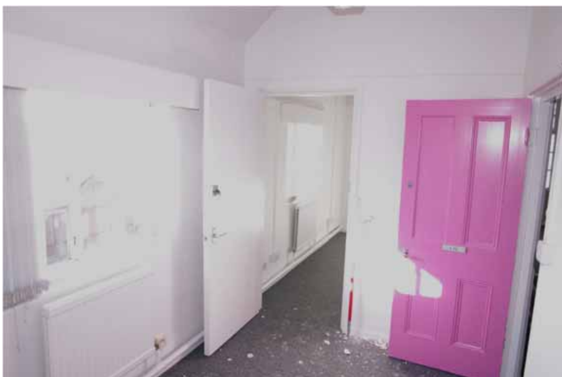
Figure 69 Room F9 looking through to F8 Looking west. 1m scale
