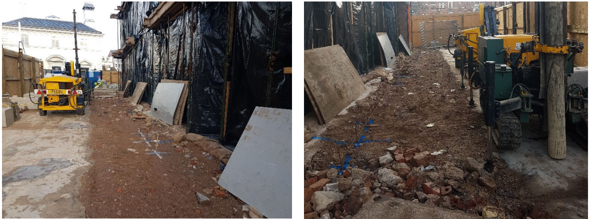
Figure 6. The pile locations marked out and located on the site
