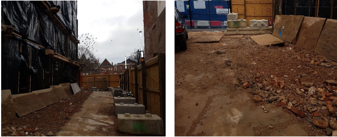
Figure 5. The site before groundworks/piling commenced
