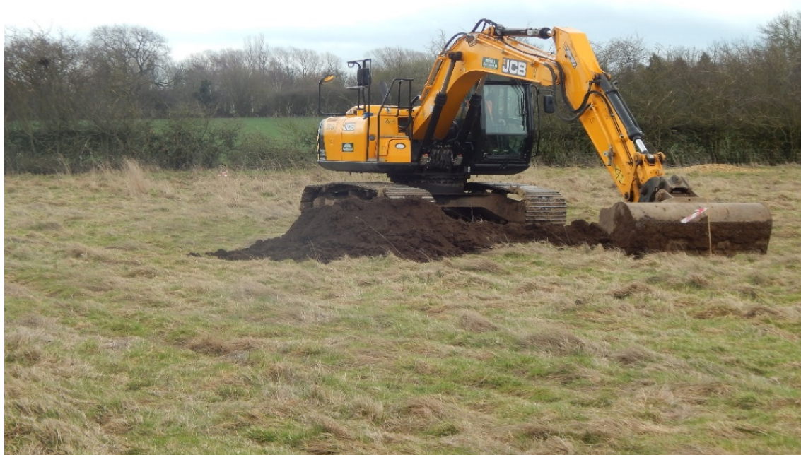
Figure 4: Excavation in progress of Trench 2, looking south-east.
