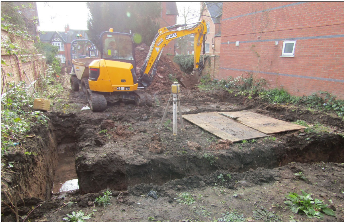
Figure 6: The site on arrival looking east.
