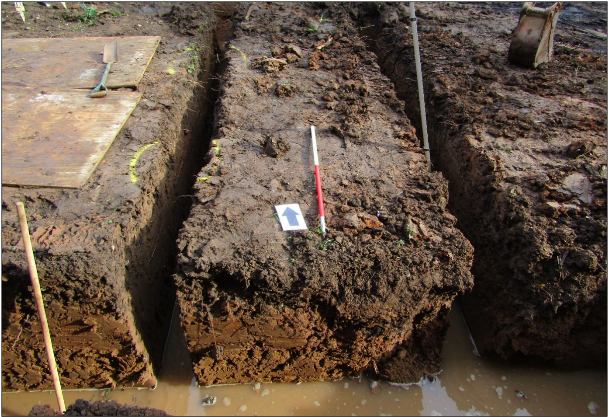
Figure 9: Internal foundation trenches looking north-northeast (1m scale).
