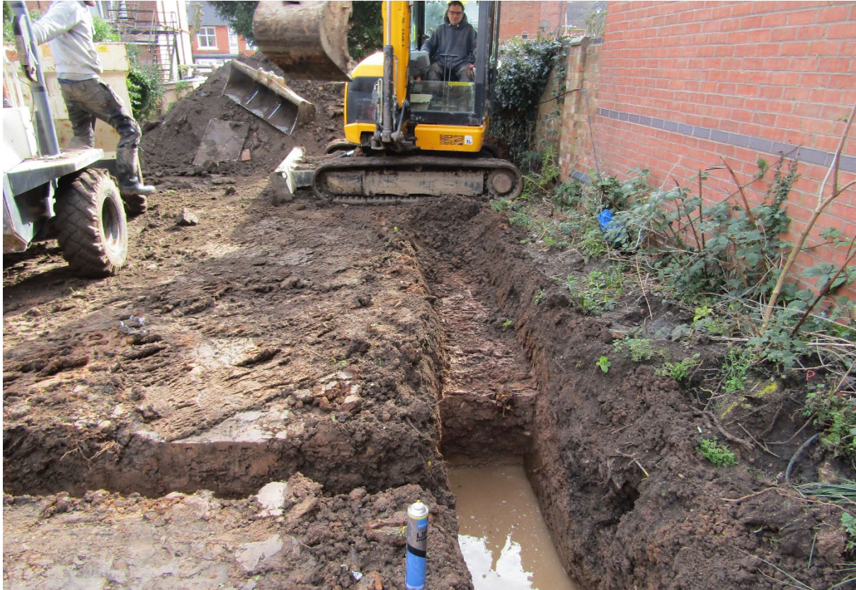
Figure 10: Eastern foundation trenches under excavation looking east.
