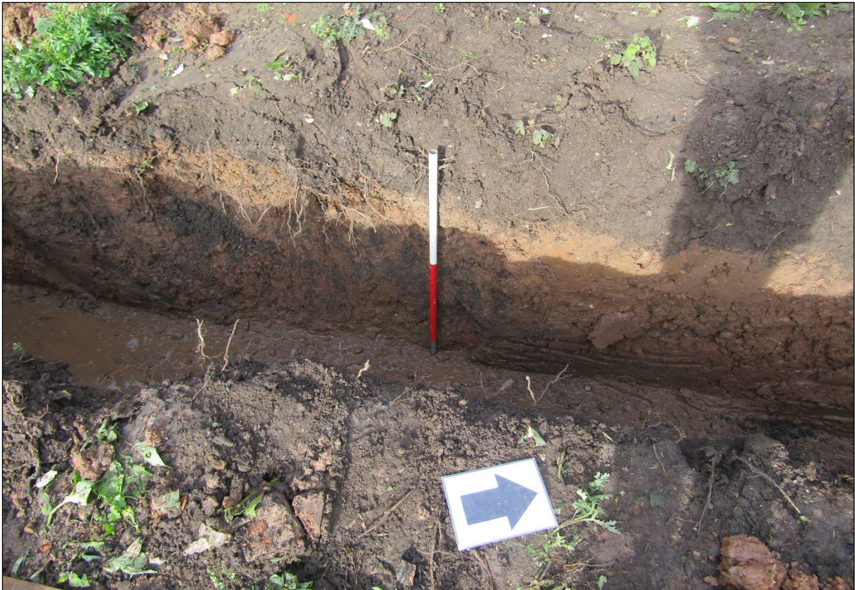
Figure 7: Section of the westernmost foundation trench looking west (1m scale).
