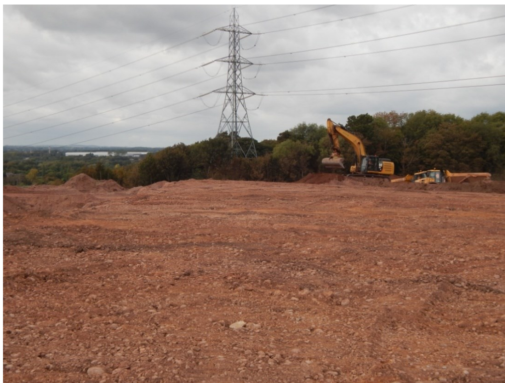
Figure 3: Soil stripping August 2018. Looking west
