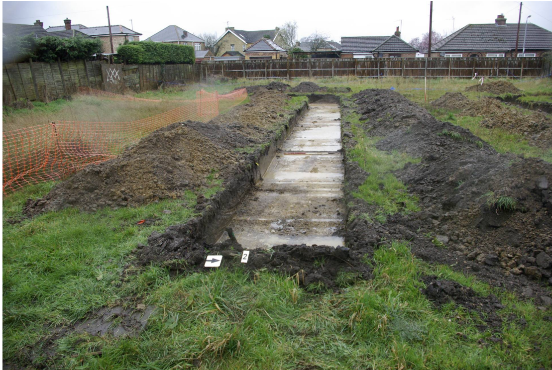
Figure 11 Trench 2 looking west. Spur at far end of trench. Disturbed area closest to camera. 1m scale
