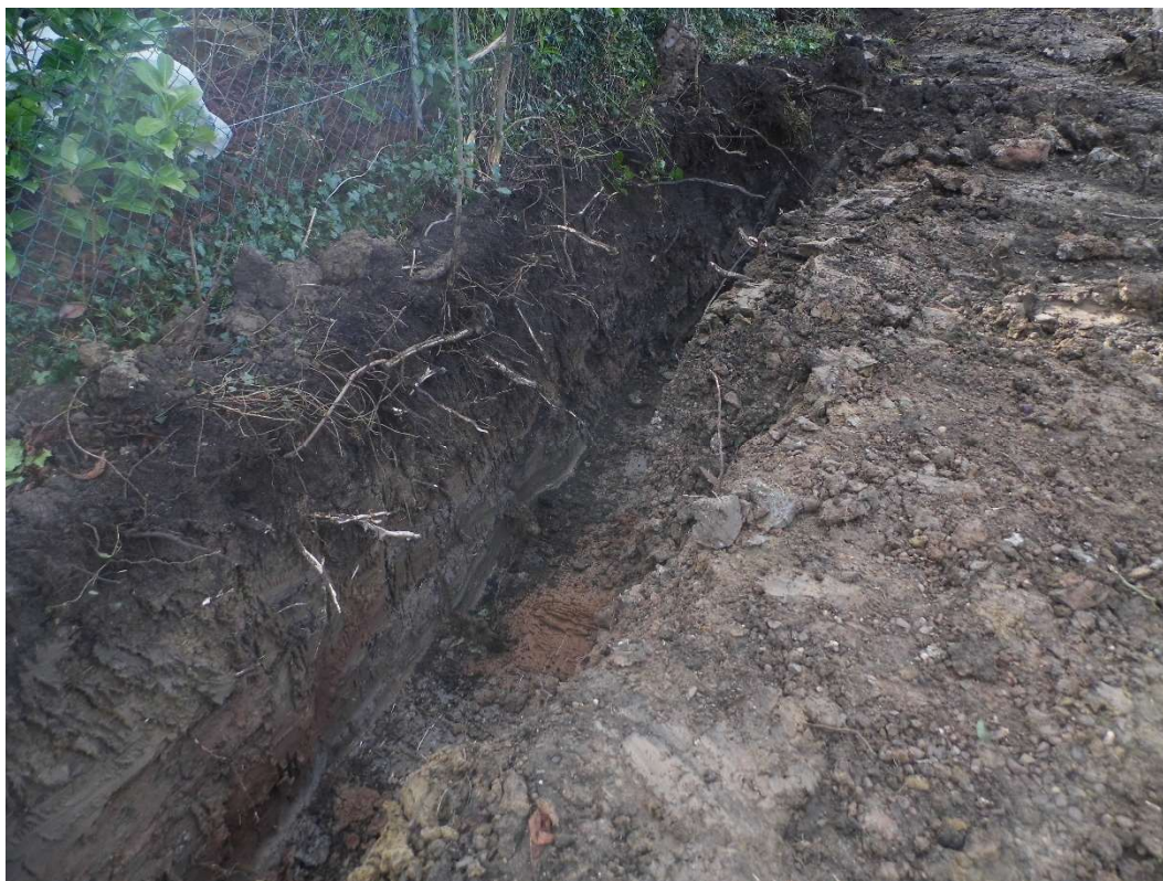
Figure 54: Possible alluvial layer in southern boundary pipe trench
