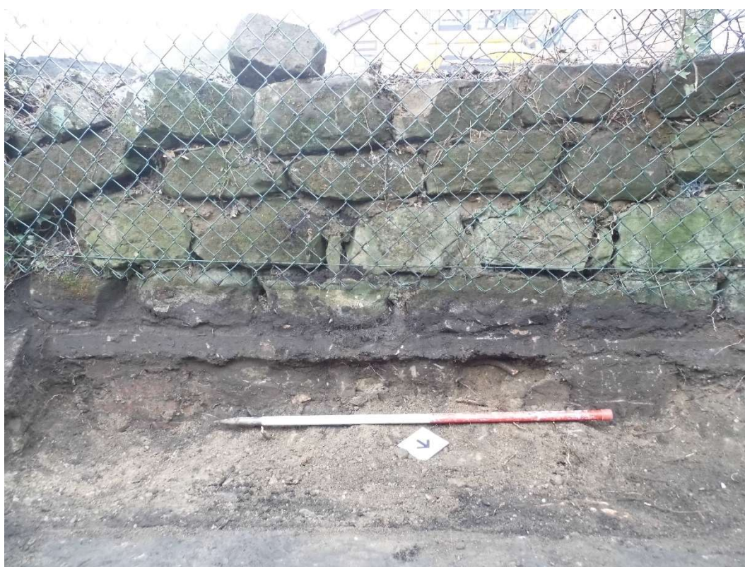
Figure 25: Rebuilt wall on original foundations
