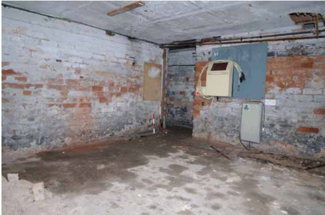
Figure 20 General view of Number 12 cellar Looking south
