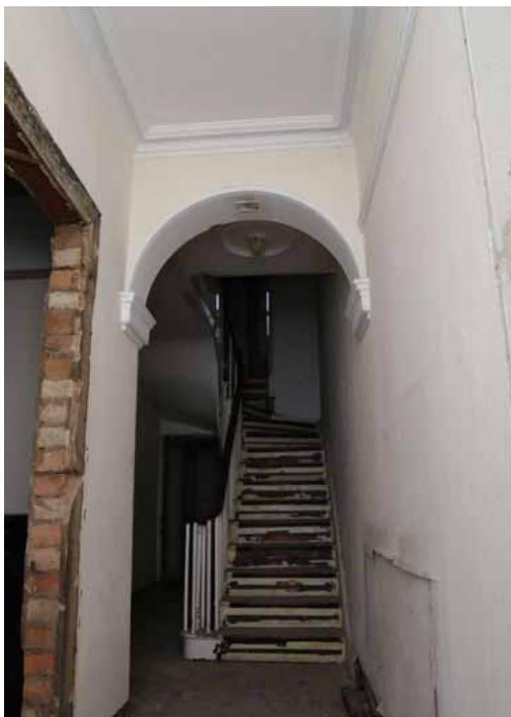
Figure 40 Number 16 staircase Looking south-east from front door
