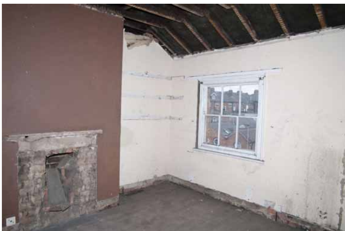
Figure 67 Number 16 second floor rear room Looking east
