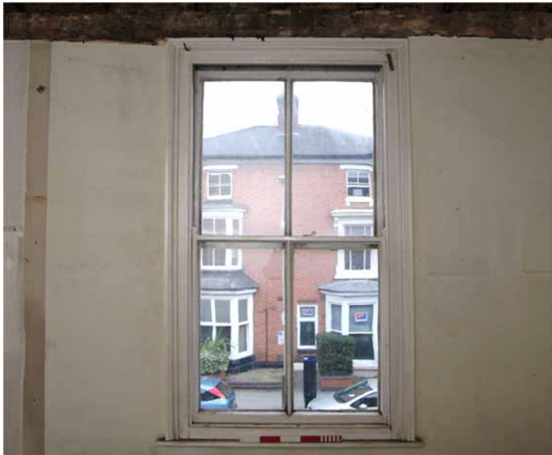
Figure 47 Number 12 first floor front room window detail
