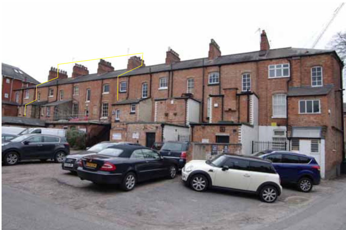
Figure 11 Rear, south-east, facing elevation Looking west. 12-16 highlighted
