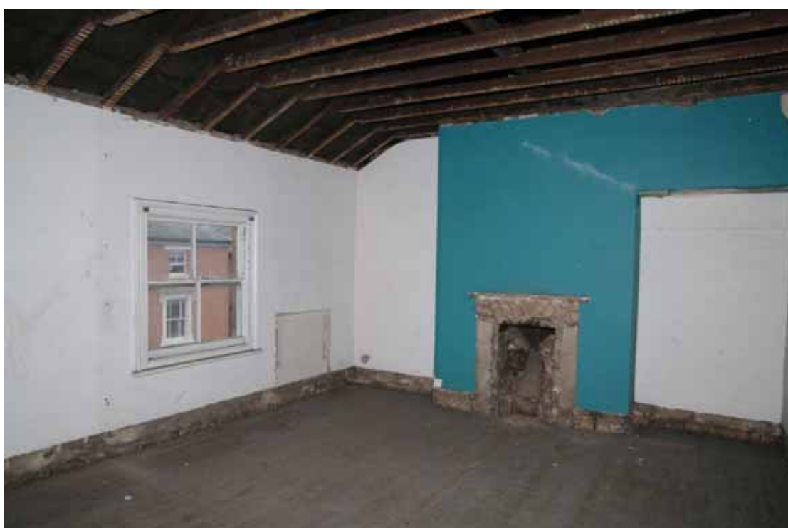
Figure 65 Number 16 second floor front room Looking north
