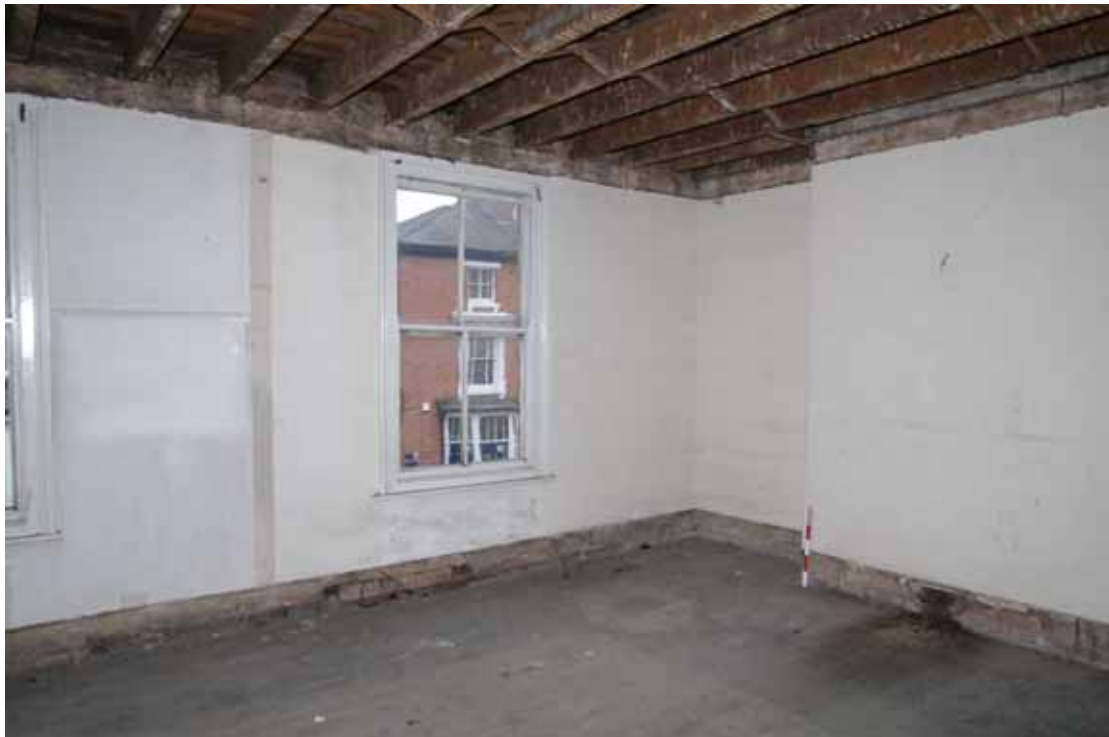
Figure 45 Number 12 first floor front room Looking north
