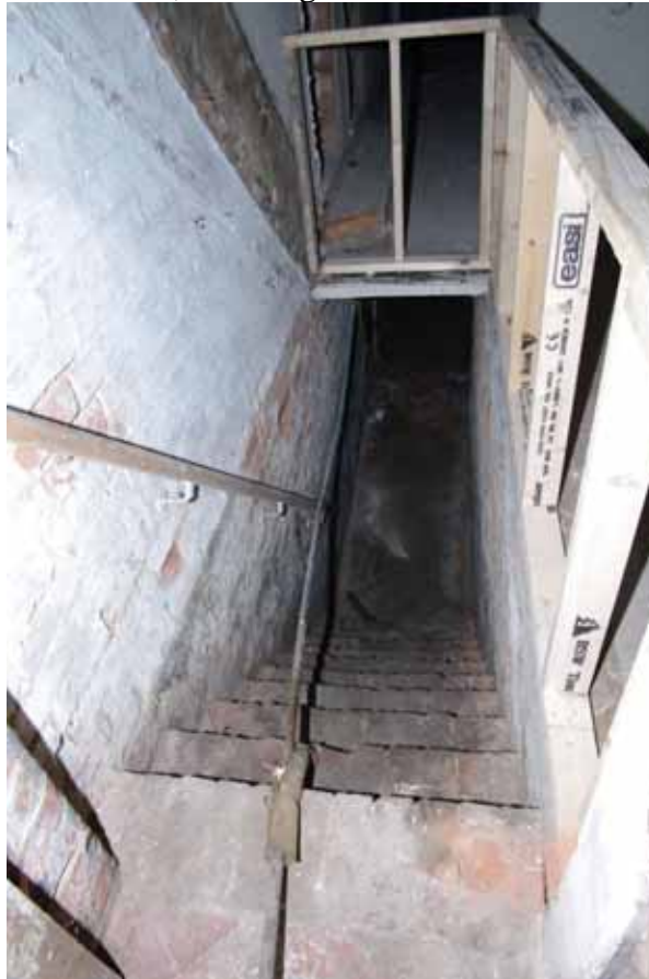
Figure 17 Stairs down to cellar of Number 12 Looking north-west
