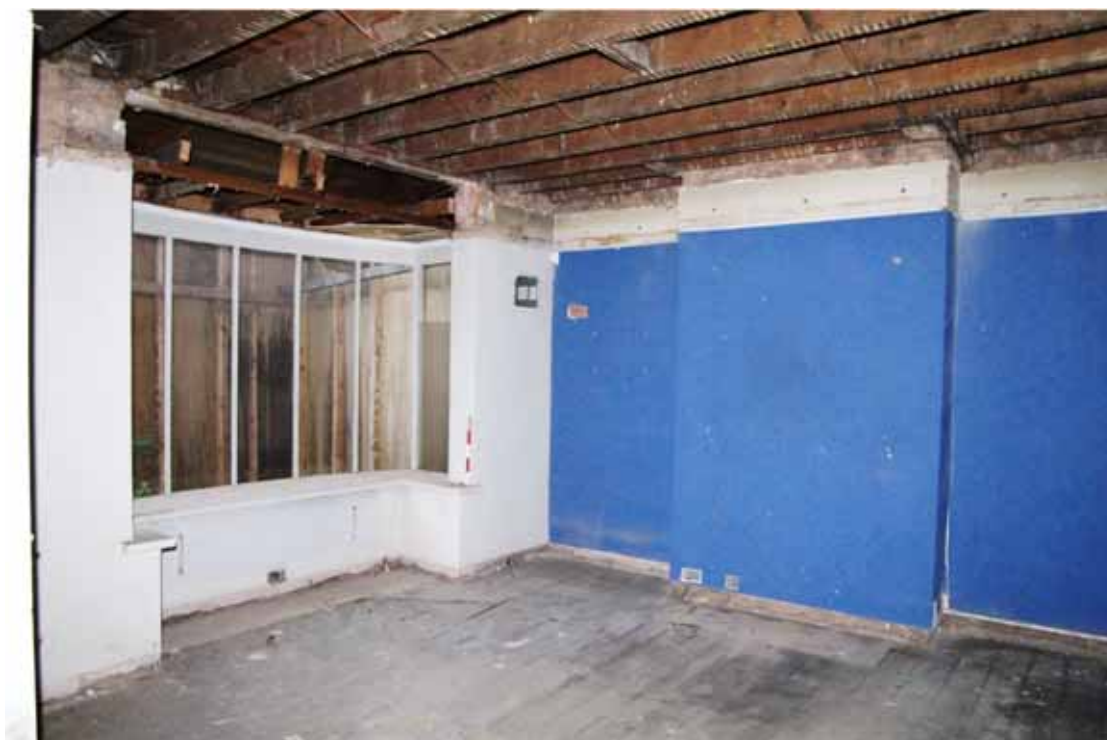
Figure 22 Number 12 ground floor front room Looking north-west
