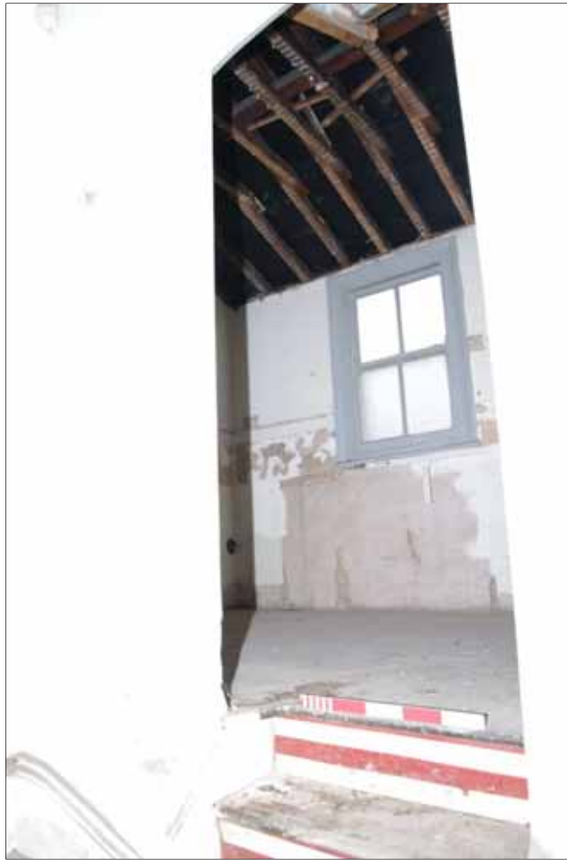
Figure 56 Number 16 first floor rear toilet block Looking south-east from stairs
