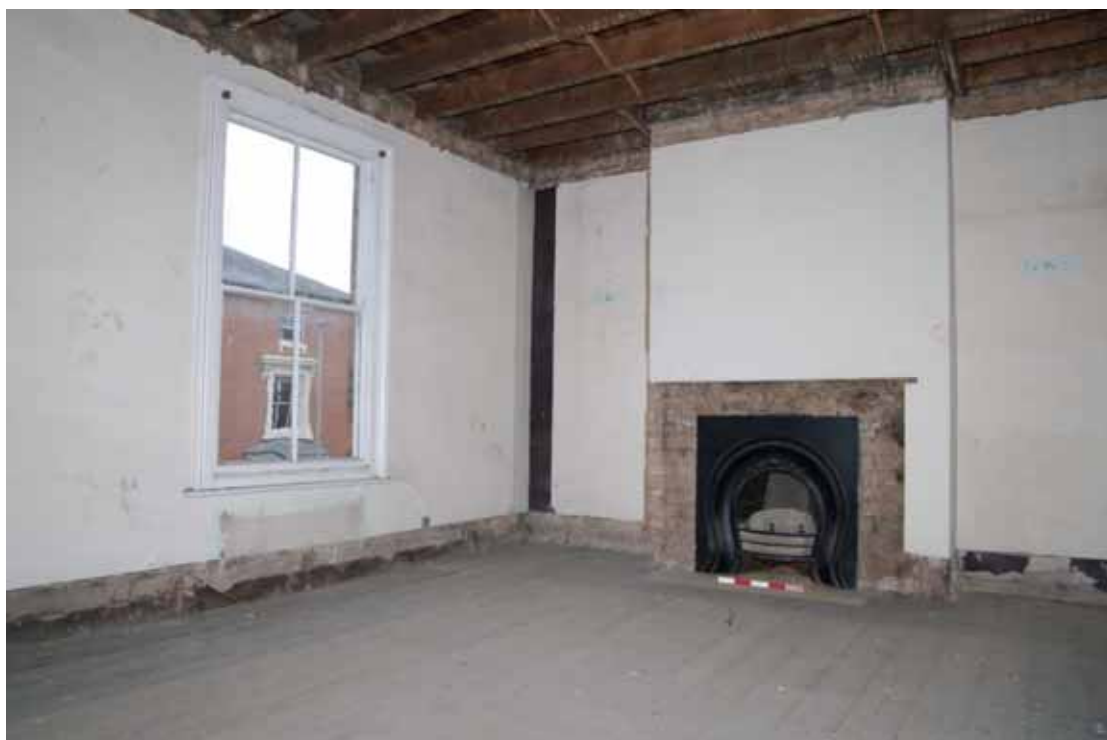
Figure 54 Number 16 first floor front room Looking north
