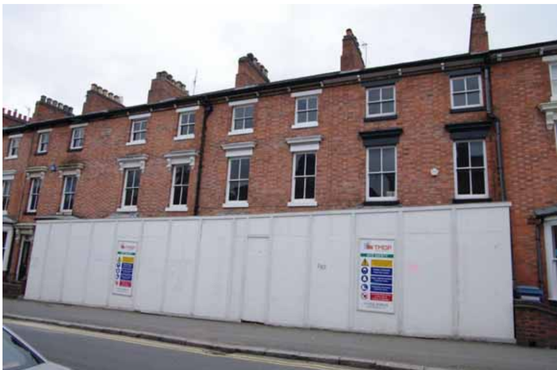
Figure 7 North-west facing elevation detail of 12-16 Looking east
