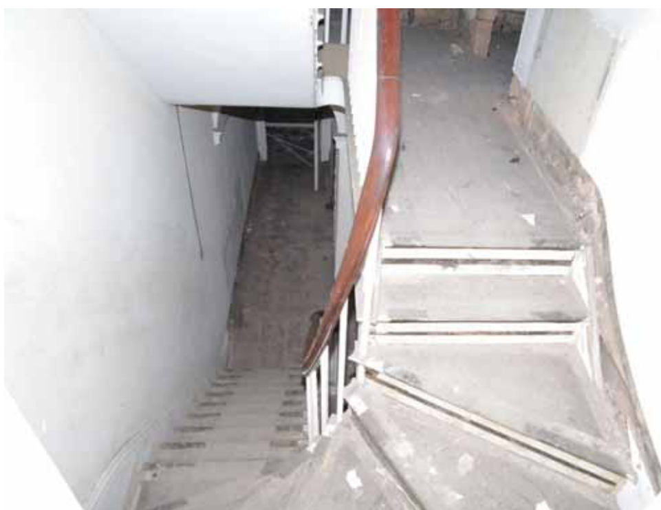
Figure 43 Number 16 staircase Looking south-east. Ground floor on left
