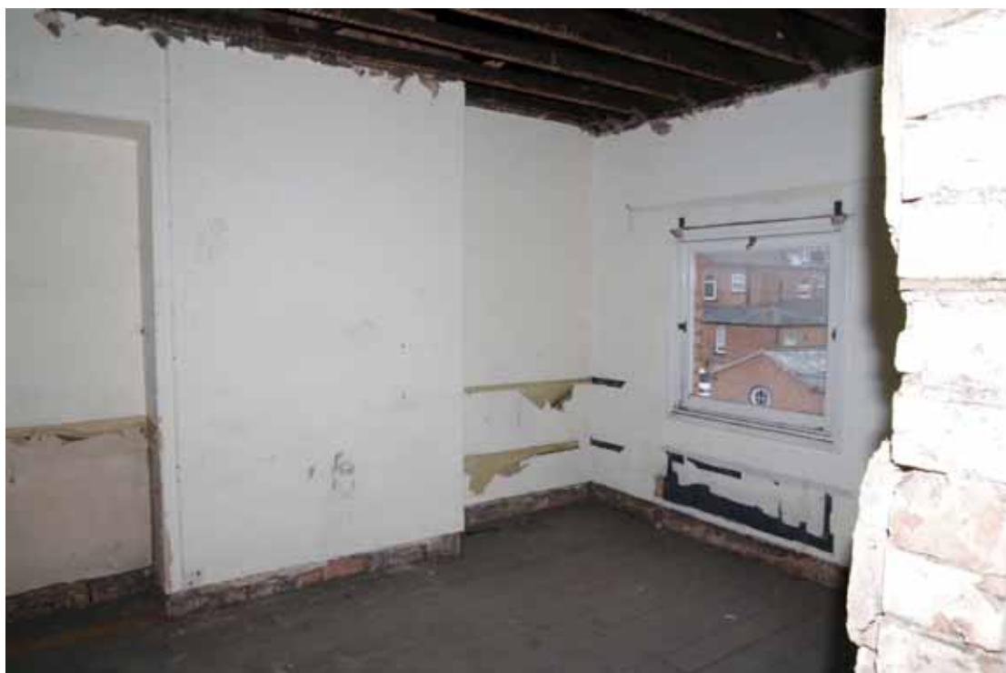
Figure 62 Number 12 second floor rear room Looking east
