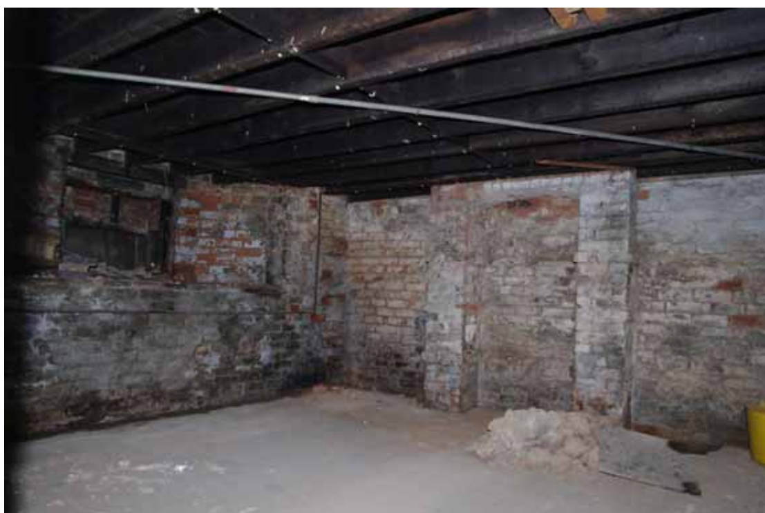
Figure 19 General view of Number 16 cellar Looking north
