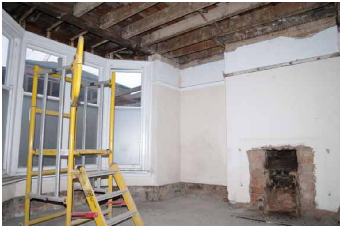
Figure 39 Number 16 front ground floor room Looking north
