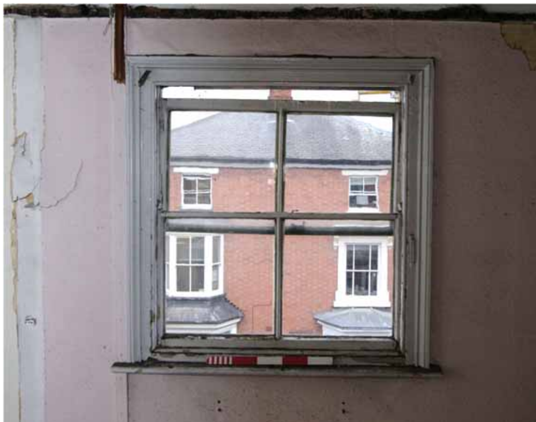
Figure 60 Number 12 second floor front room window detail
