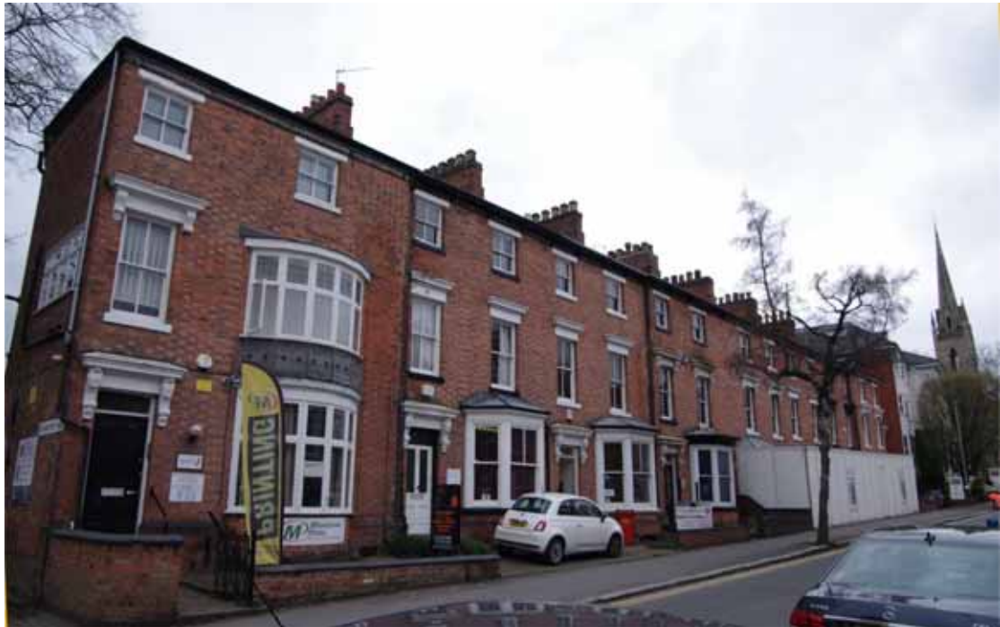
Figure 6 De Montfort Place Terrace Looking south-east. Numbers 12-16 behind white hoarding. Note Bow-fronted bay of Number 4 compared with the other ground floor bays of the remaining terrace
