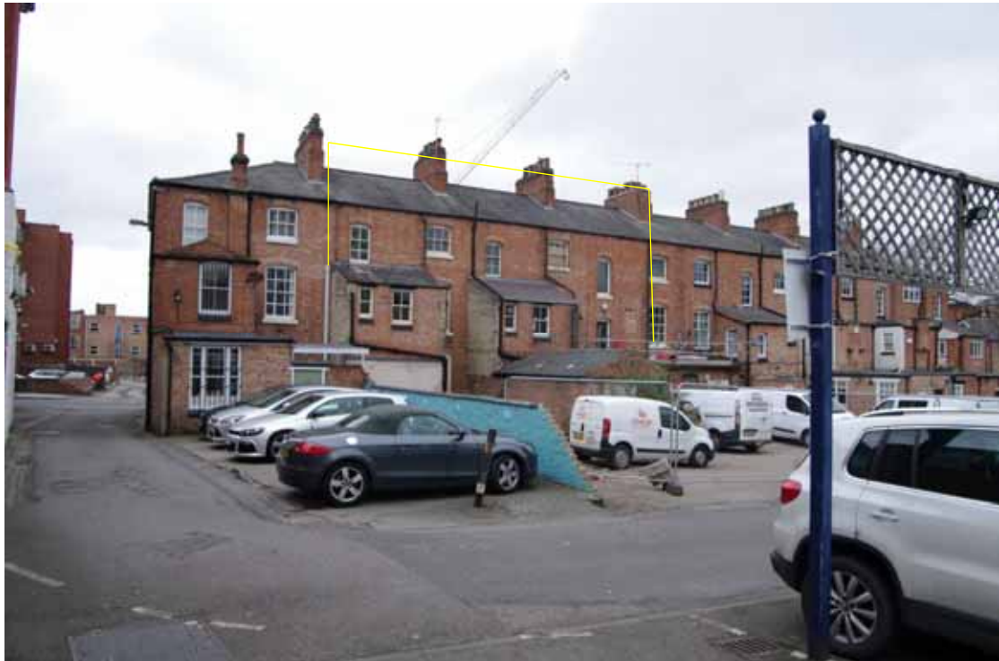
Figure 10 Rear, south-east, facing elevation Looking north. 12-16 highlighted
