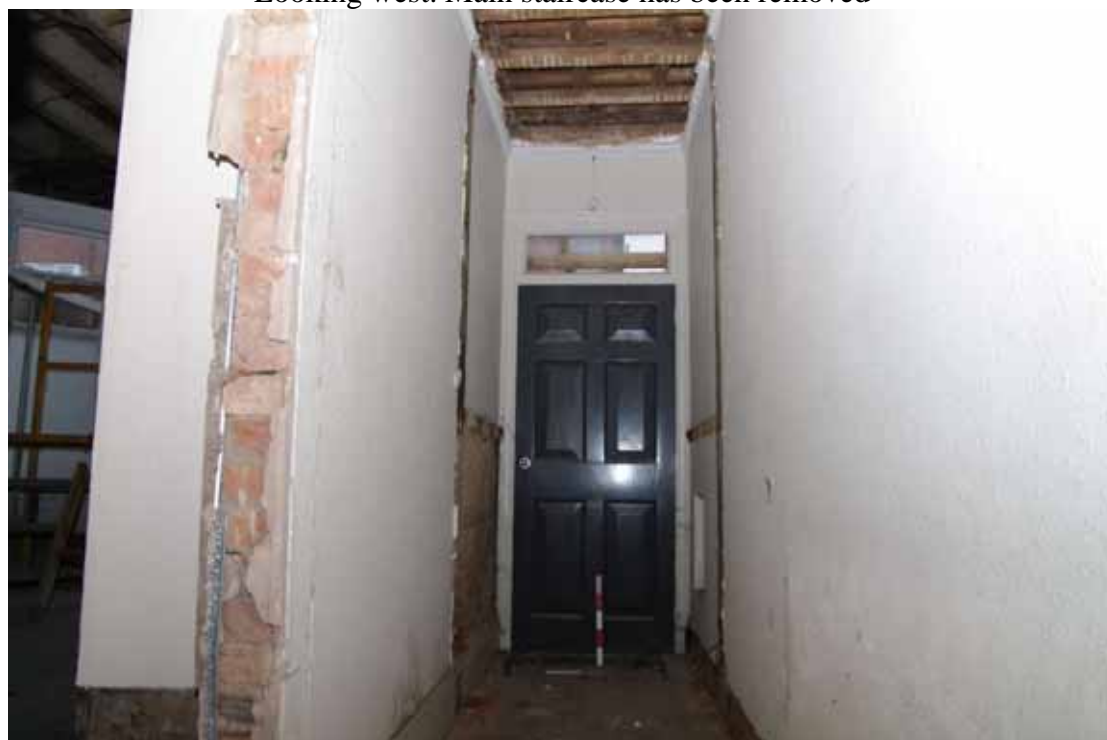
Figure 35 Number 14 front door Looking south-east. Knocked-through doorway to Number 16 on right
