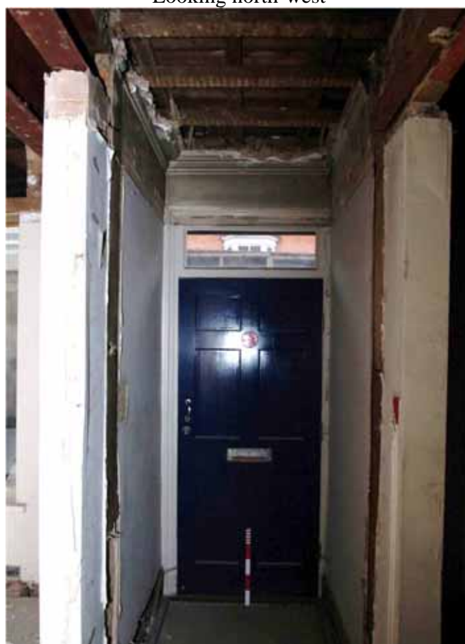
Figure 23 Hallway and front door of Number 12 Looking west
