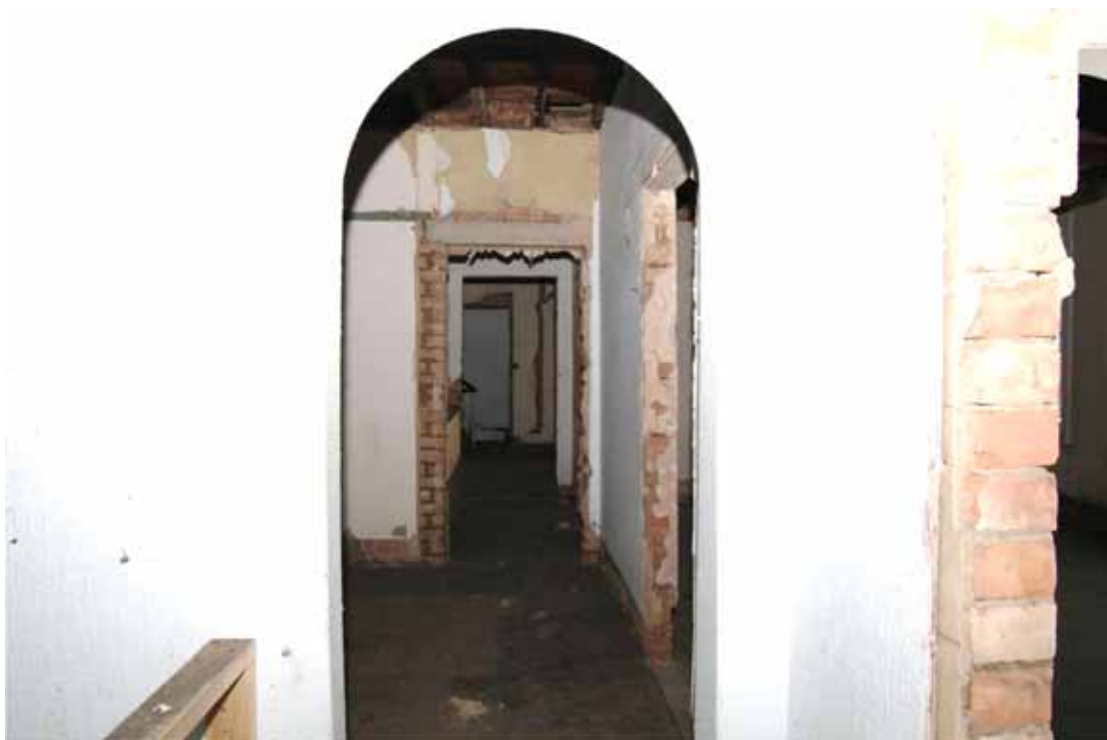
Figure 50 First floor connecting corridor Looking south-west from Number 12
