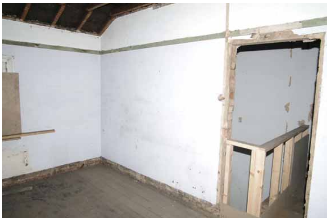
Figure 64 Number 14 second floor rear room Looking south
