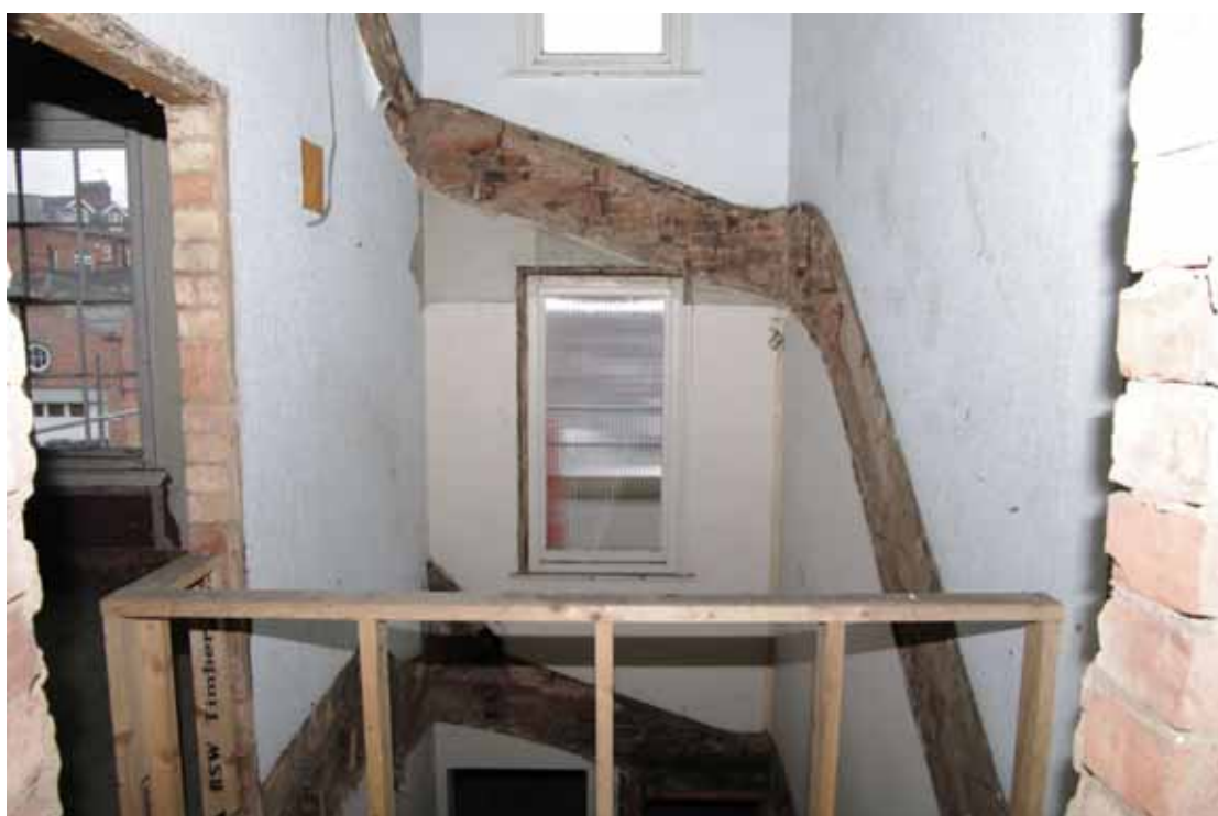
Figure 49 Number 12 removed stair case at first floor level Looking south-east
