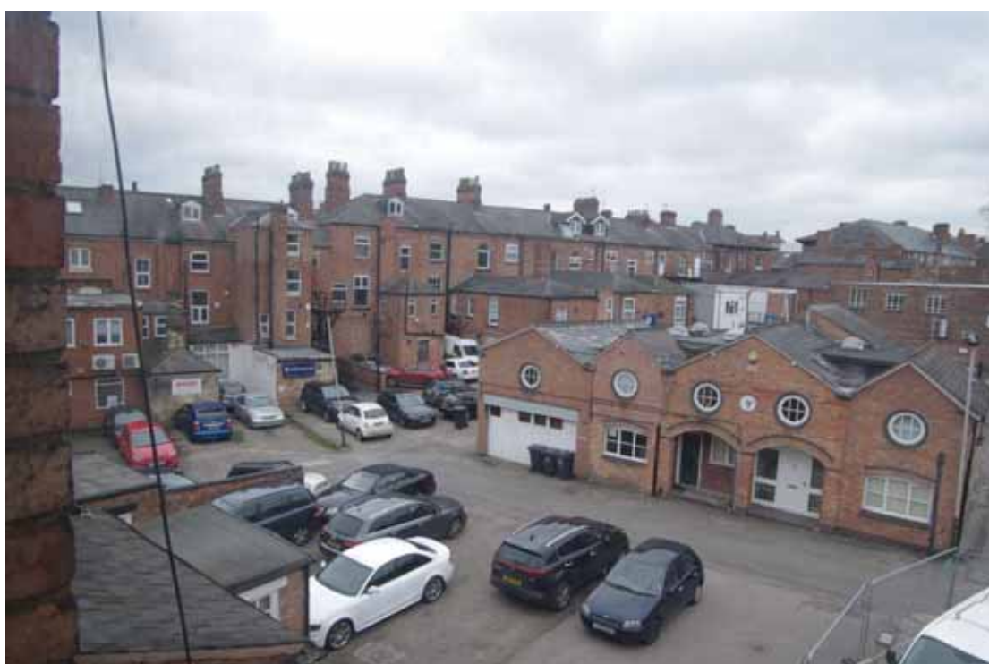
Figure 15 Former stable block to rear of 12-16 Looking east from first floor of Number 12. Houses fronting onto London Road on left of photograph
