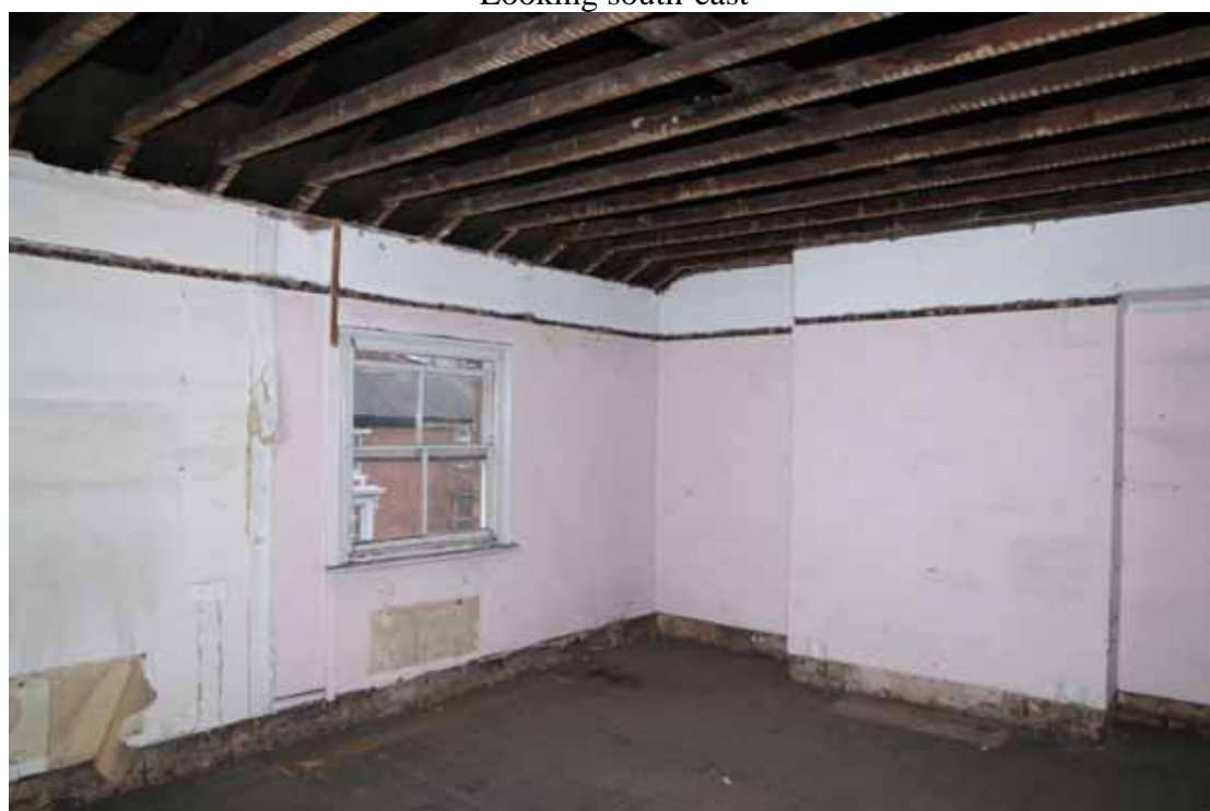
Figure 59 Number 12 second floor front room Looking north
