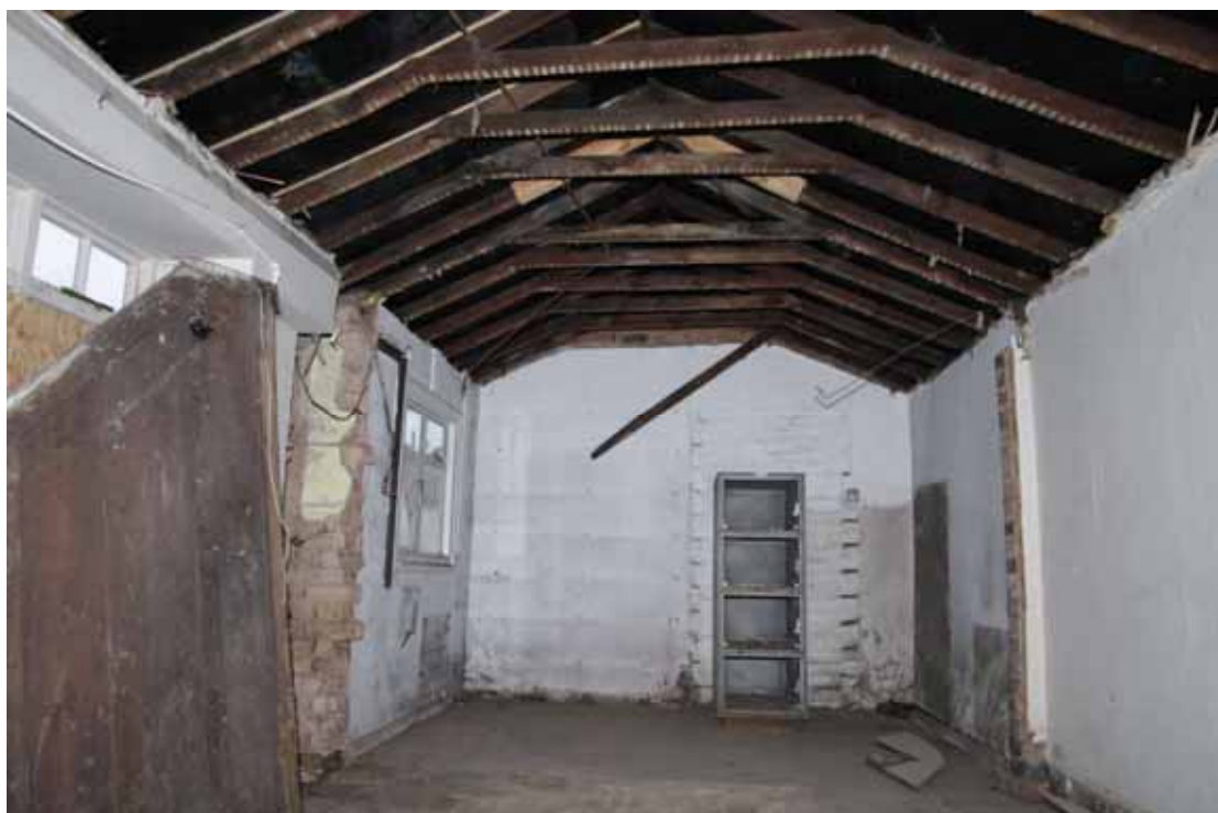
Figure 37 Rear extension to rear of Number 14 Looking south-east
