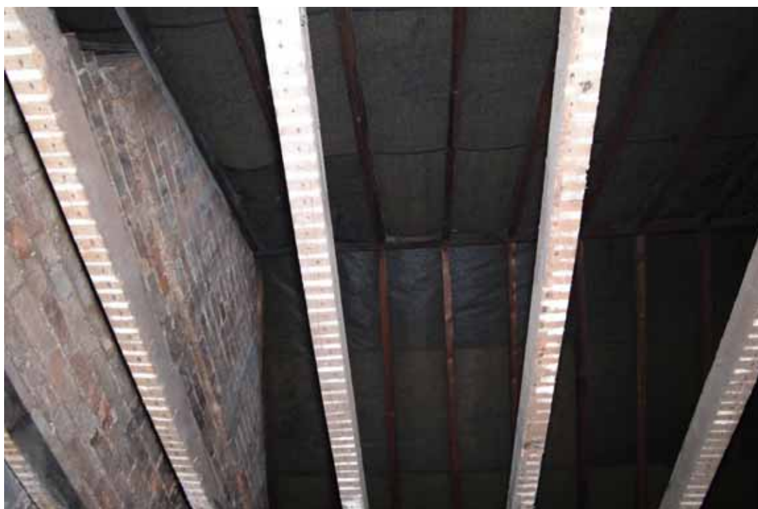
Figure 61 Number 12 underside of roof detail
