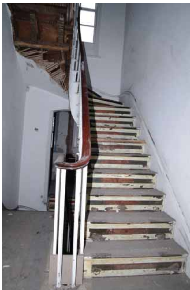
Figure 58 Number 16 staircase up from first to second floor Looking south-east
