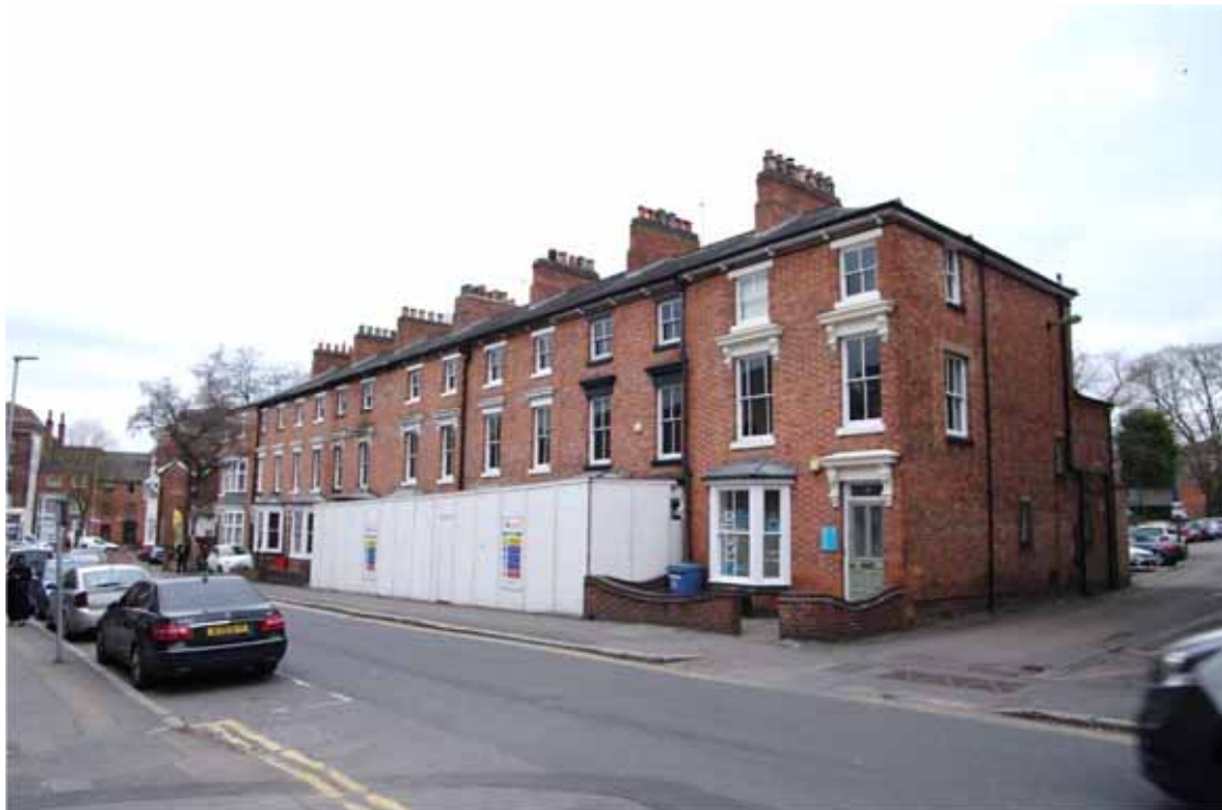
Figure 5 De Montfort Place Terrace facing onto De Montfort Street Looking north-east. London Road on left. Numbers 12-16 behind white hoarding
