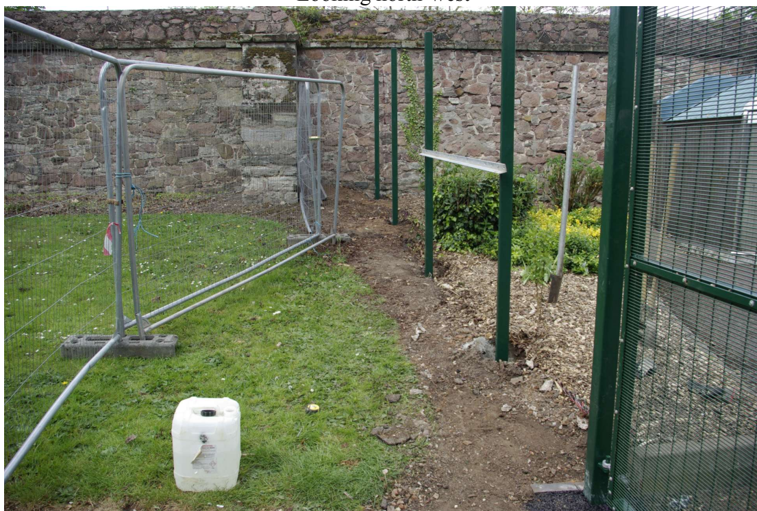
Figure 6 North-westernmost post holes after setting up new posts Looking north-west
