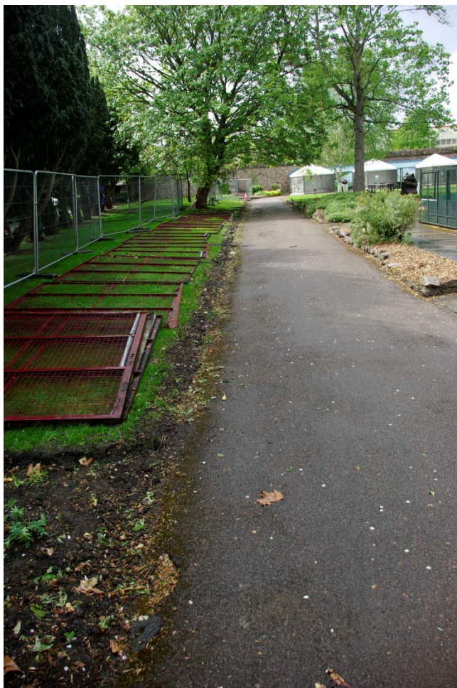
Figure 5 Old fence after removal Looking north-west
