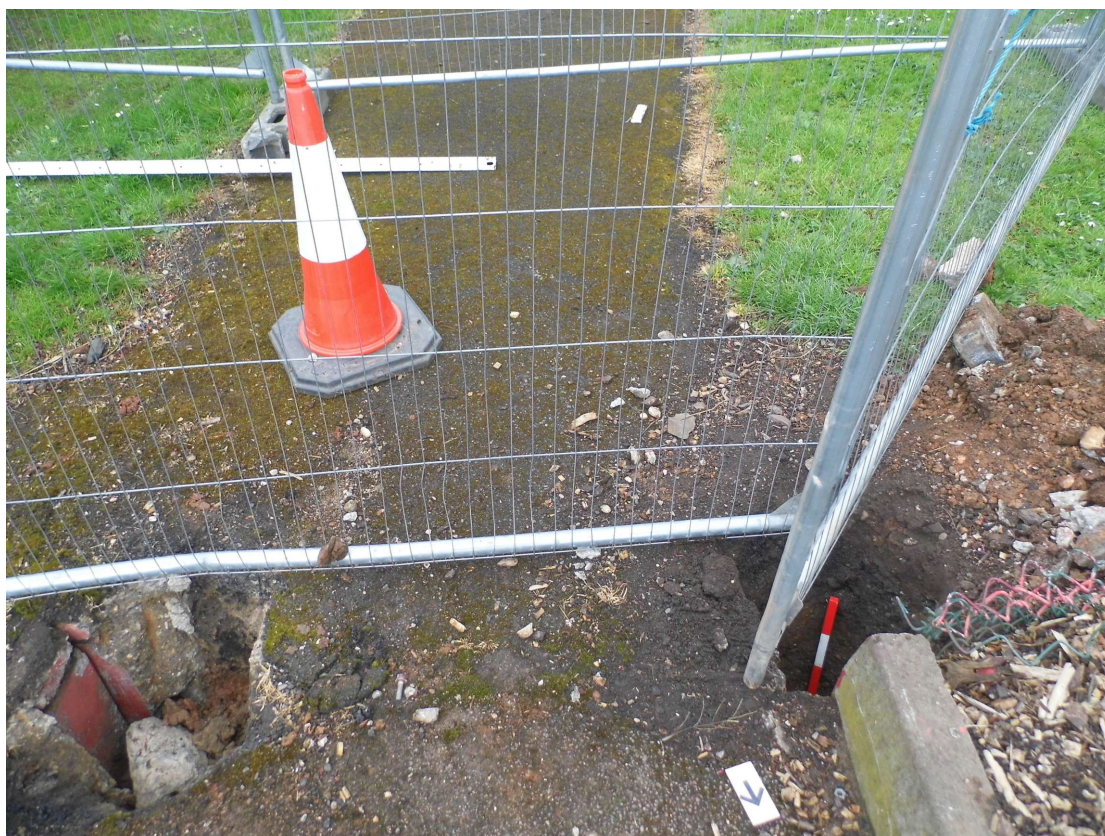
Figure 7 Gatepost holes near to north-western end of new fence
