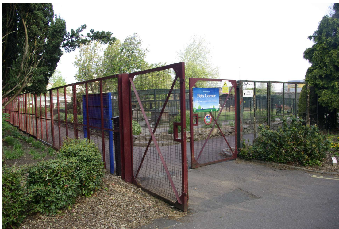
Figure 4 Old fence and gate to be replaced Looking north-west. Only the fence panels on the left were being replaced
