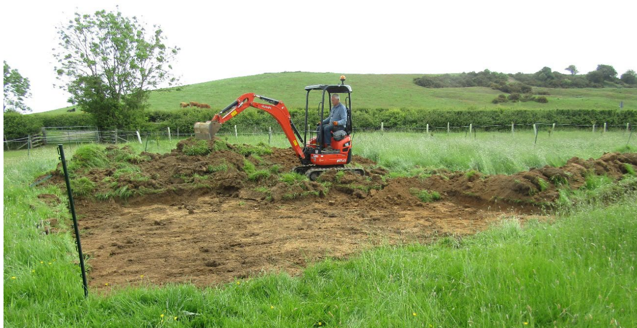
Figure 7: Excavation underway. Looking north-east.
