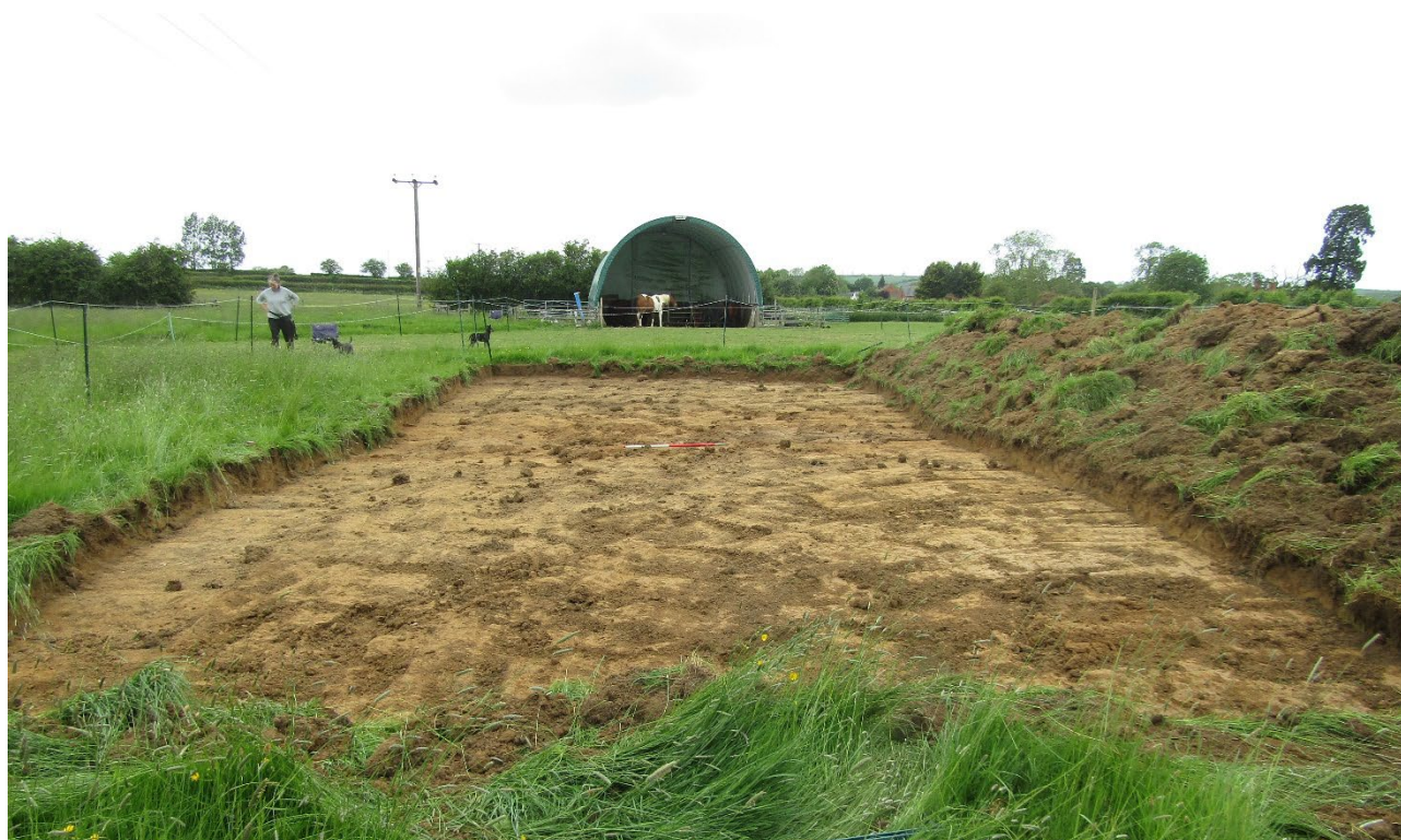
Figure 8: Site fully stripped. Looking north west.
